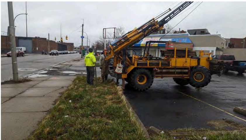
11. View of BH-4 location looking north-northeast
