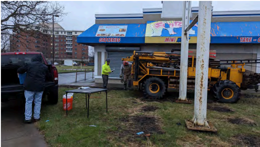
1. View of BH-1 location looking southeast
