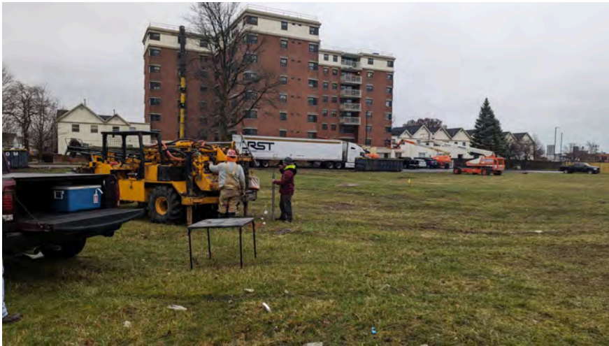
13. View of BH-5 location looking southeast
