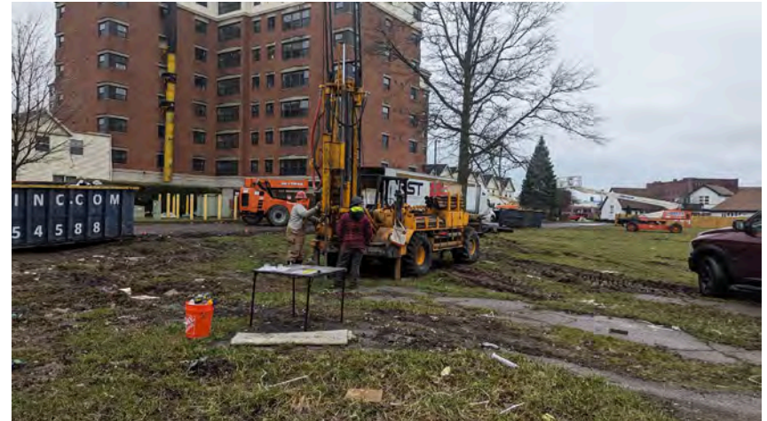
16. View of BH-6 location looking southeast
