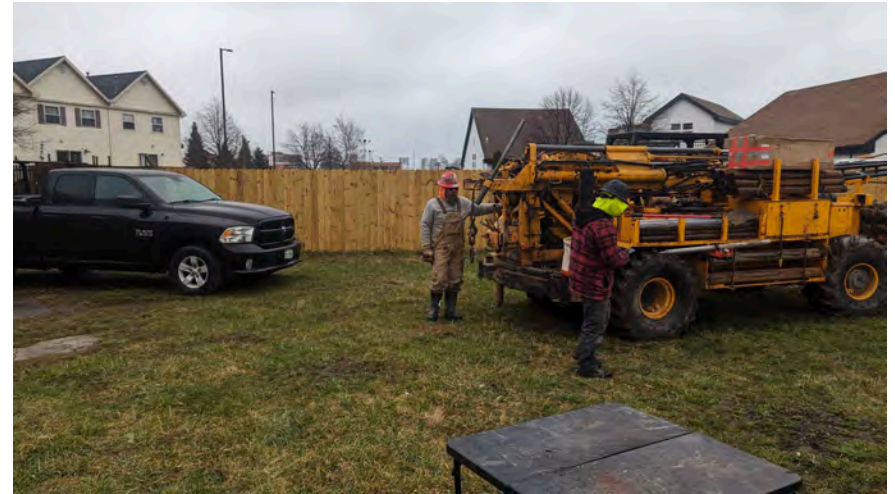
38. View of BH-13 location looking south
