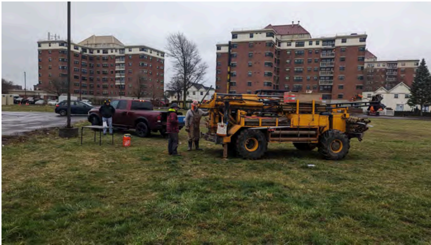
25. View of BH-9 location looking east
