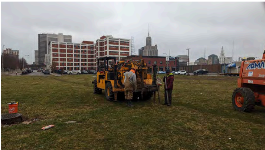
31. View of BH-11 location looking northwest
