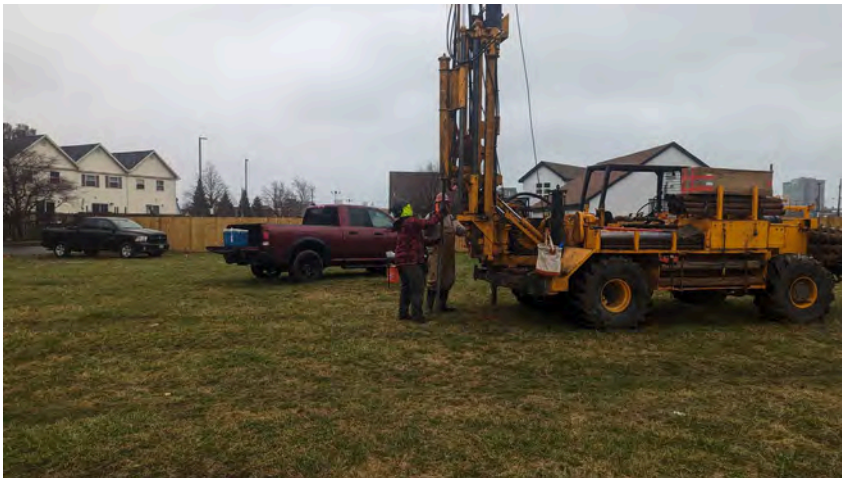
35. View of BH-12 location looking south
