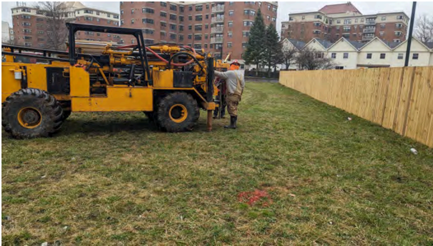
41. View of BH-14 location looking east
