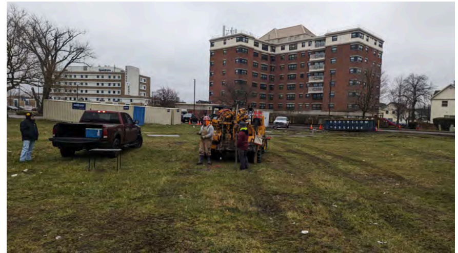
14. View of BH-5 location looking east-northeast
