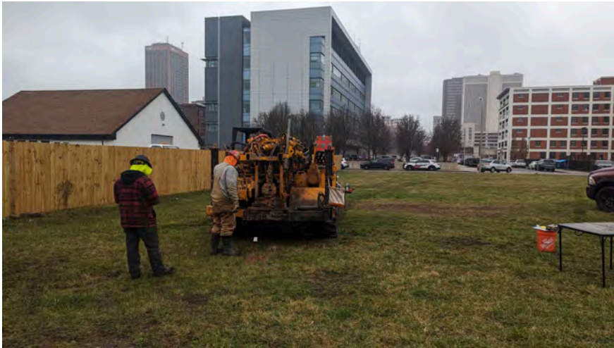
37. View of BH-13 location looking southwest
