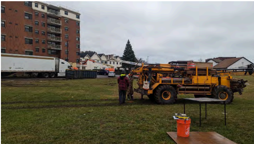
19. View of BH-7 location looking south
