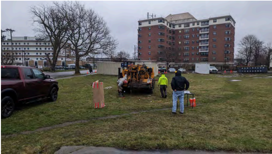
5. View of BH-2 location looking southeast
