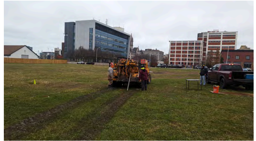
20. View of BH-7 location looking southwest
