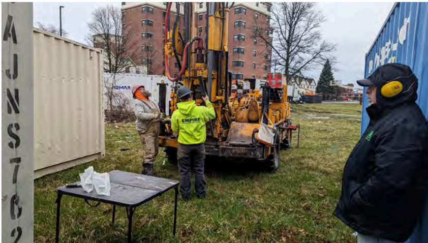
7. View of BH-3 location looking south
