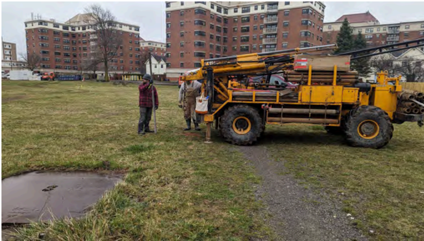
29. View of BH-10 location looking east
