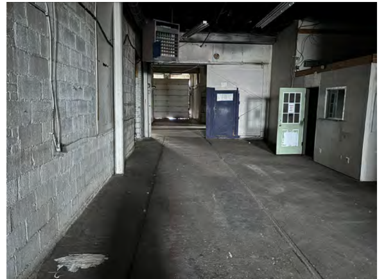
32. View of western portion of 1628 Elmwood Avenue
