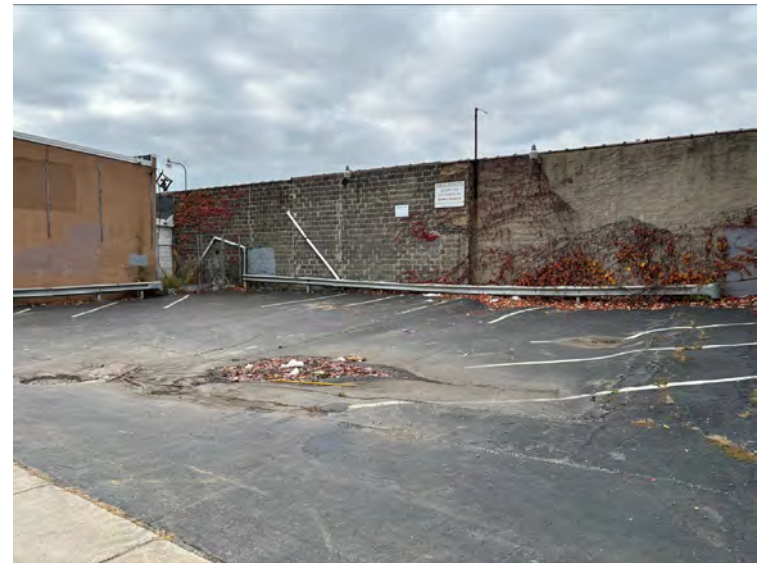
8. View of 1624 Elmwood Avenue and east side of 680 Amherst Street, facing west
