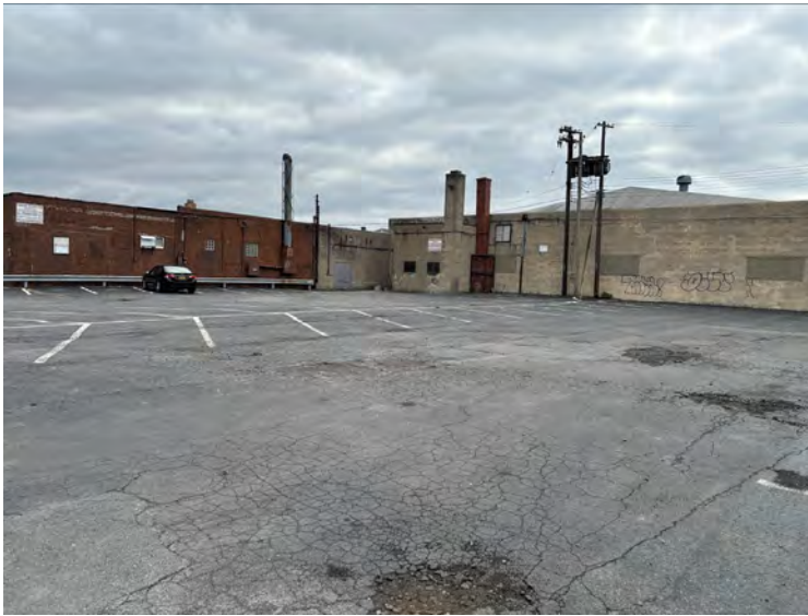
1. View of north side of 680 Amherst Street and west side of 1628 Elmwood Avenue facing southeast.
