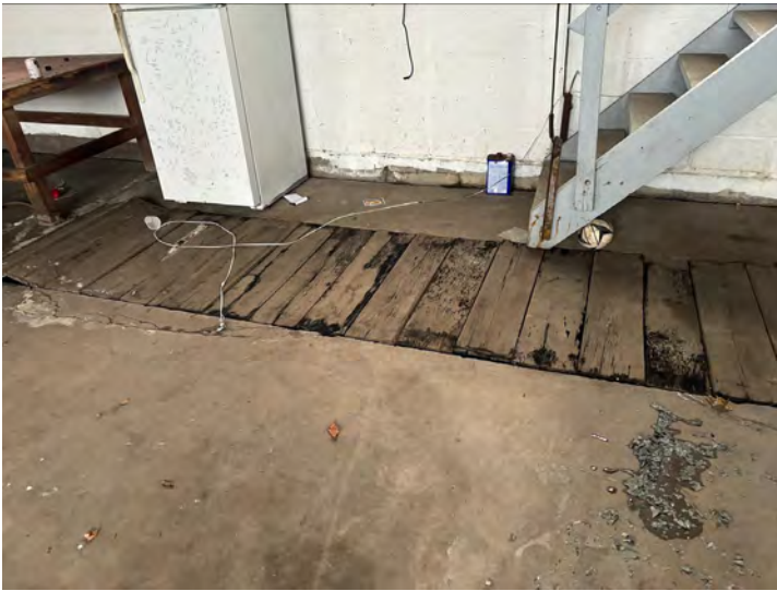
25. Covered crawl space on western side of 155 Marion Street.
