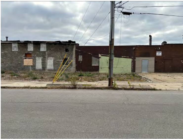
5. View of 1634 Elmwood Avenue and northside of 1628 Elmwood Avenue, facing south
