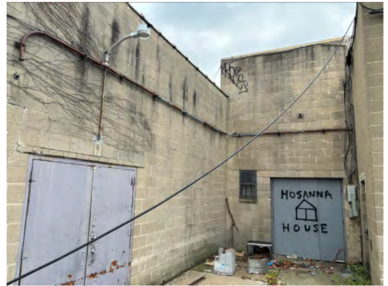
2. View of northeast corner of 680 Amherst Street, facing southeast
