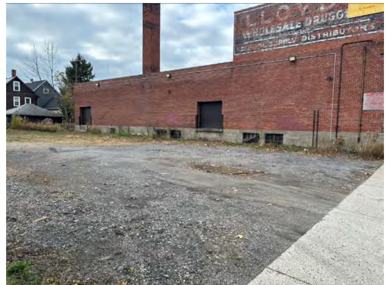
20. View of adjacent properties of 155 Marion Street, facing west.
