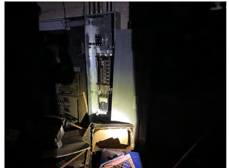
46. Utilities in basement of 680 Amherst Street.
