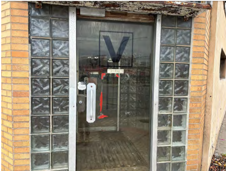
11. Front entrance to Voelker's Bowling Lanes on southeast corner of 680 Amherst Street.
