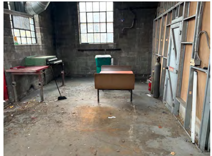
28. Southwest corner of 155 Marion Street.
