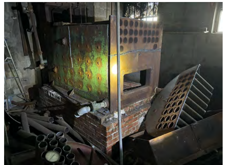
44. Machinery on northwestern side of 680 Amherst Street.
