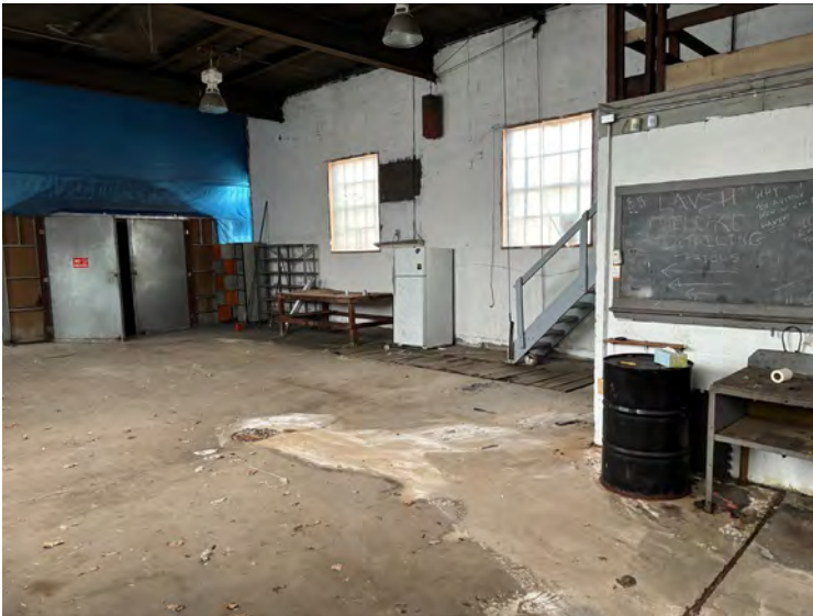
23. Western wall of 155 Marion Street.
