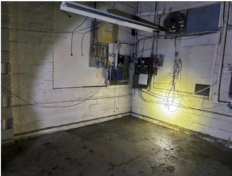
35. Utilities on southern portion of 1628 Elmwood Avenue..
