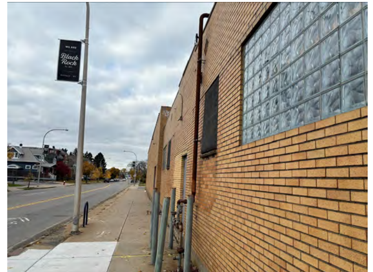
12. View of south side of 680 Amherst Street, facing west
