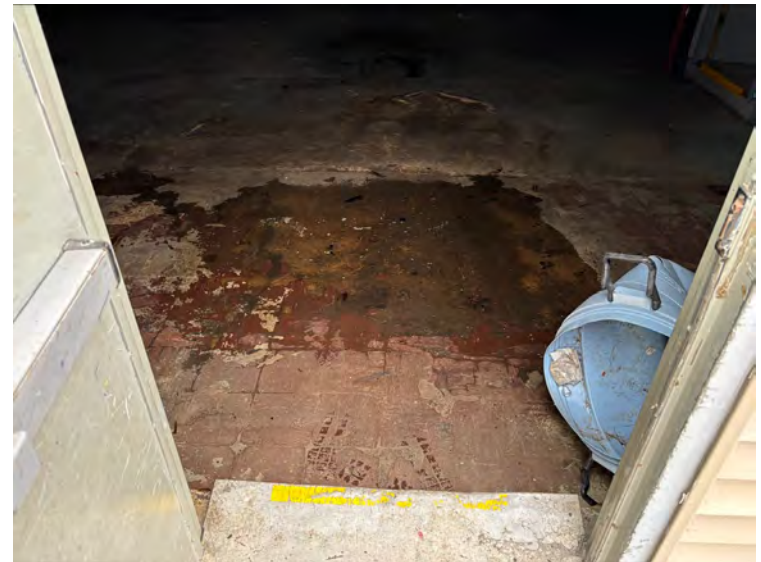
36. Northern entrance to 1628 Elmwood Avenue.
