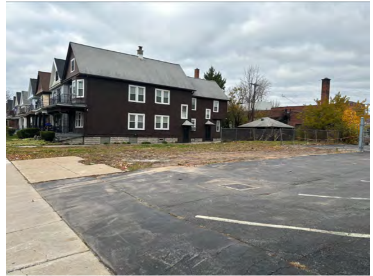
14. View of 670, 668, and 666 Amherst Street (vacant lots and parking spaces). Facing northwest.
