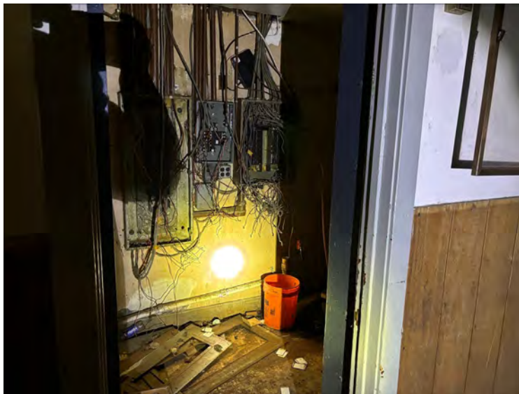
43. Utilities on northwestern side of 680 Amherst Street.
