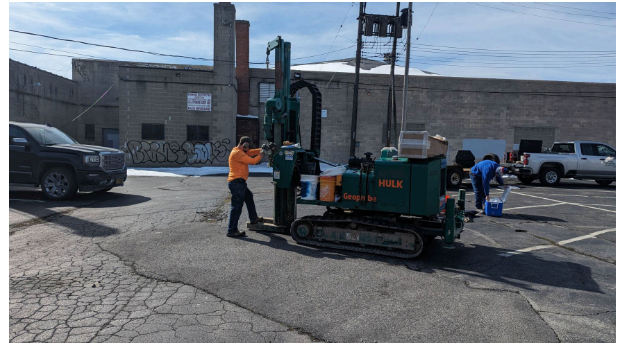
22. View of BH-8 location looking south
