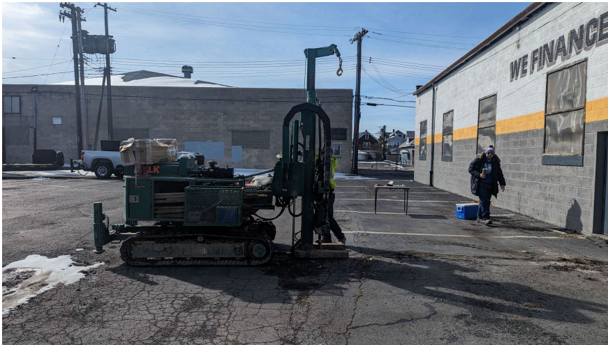
17. View of BH-6 location looking south
