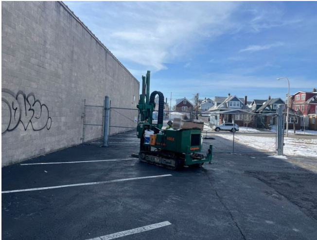
13. View of BH-5 location looking south
