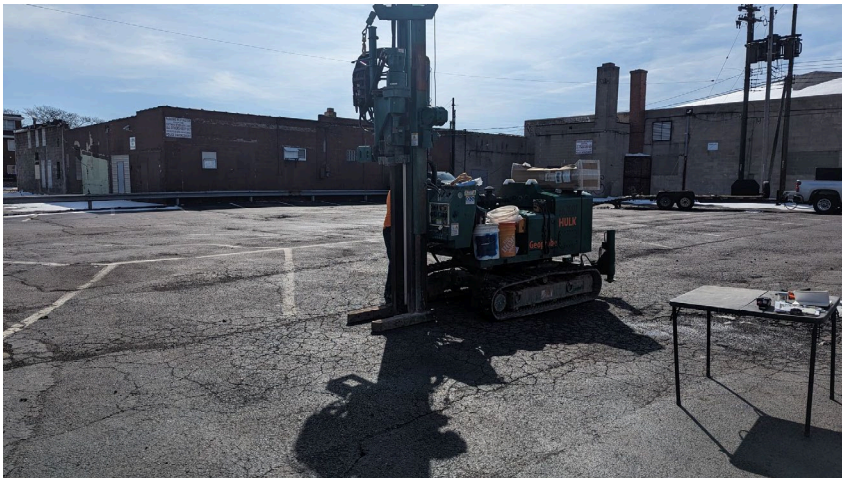
19. View of BH-7 location looking southeast
