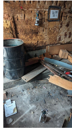
42. View of SS-5 and IA-5 location
