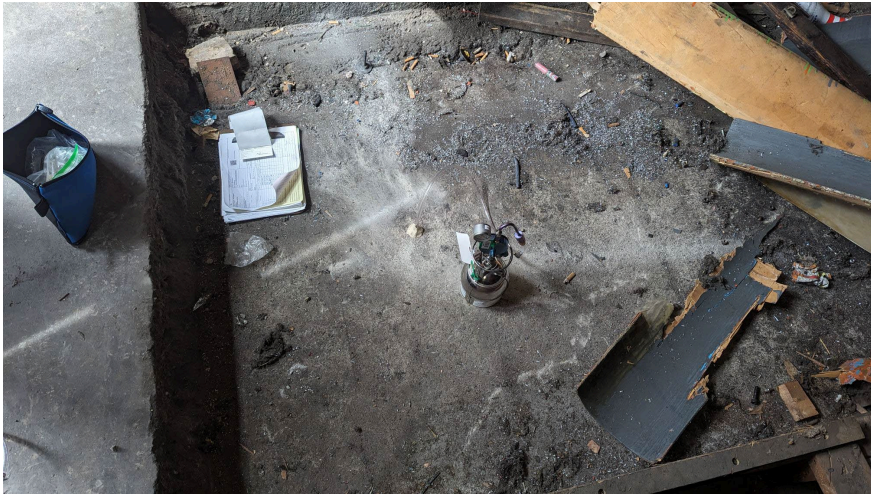
41. View of SS-5 location
