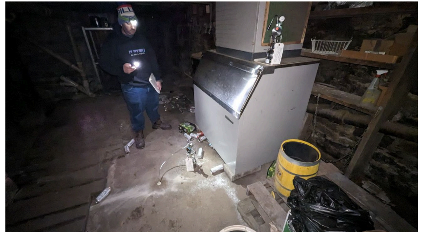
40. View of SS-1 and IA-1 location
