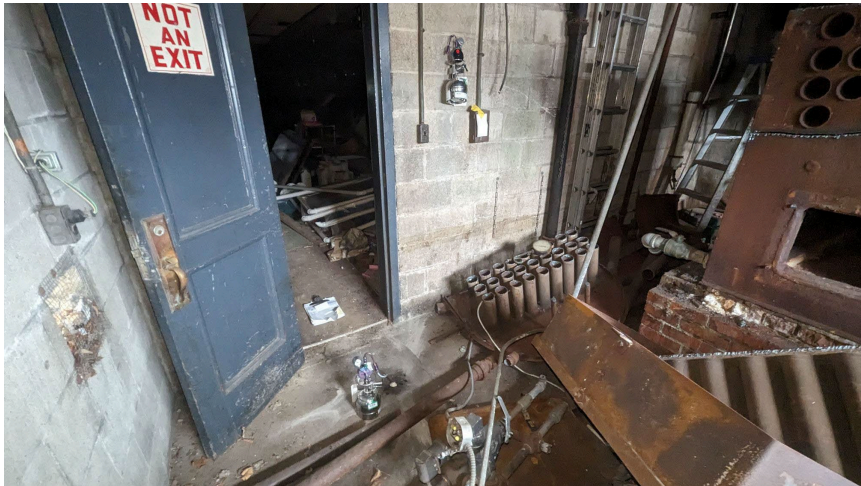
43. View of SS-3 and IA-3 location
