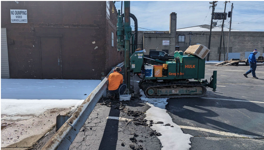
25. View of BH-9 location looking south
