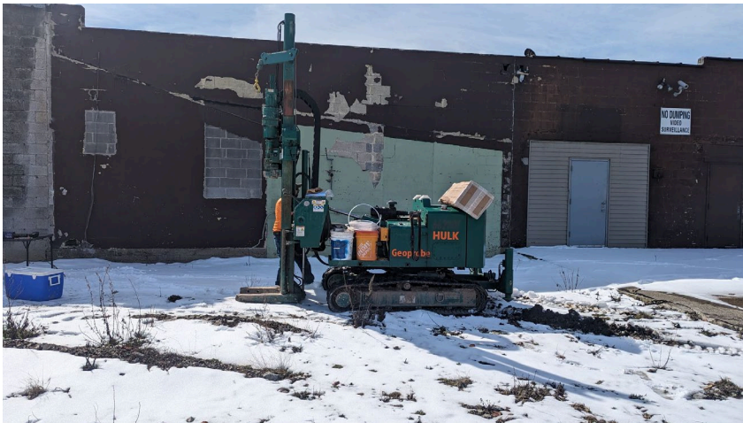
27. View of BH-10 location looking south
