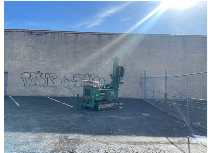
14. View of BH-5 location looking east
