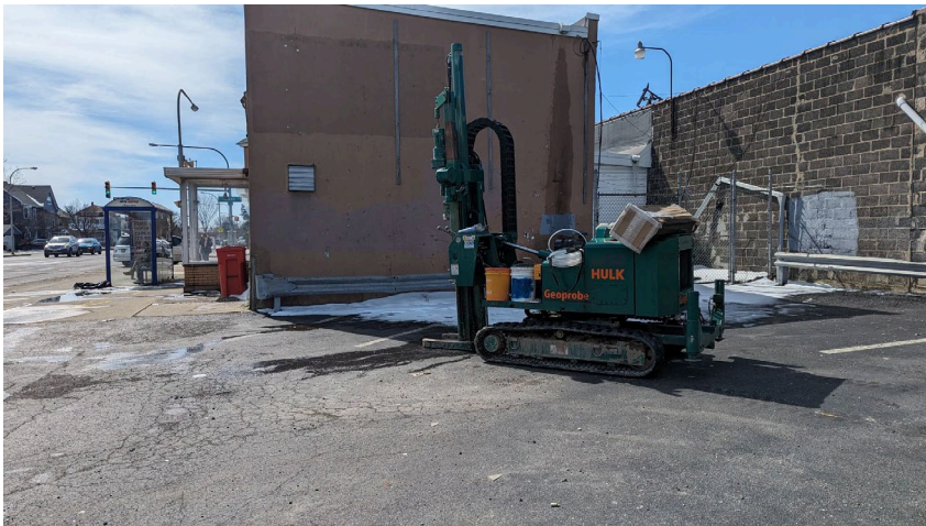
35. View of BH-13 location looking south
