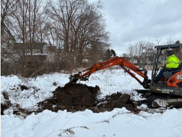
13. Test pit 7 location.
