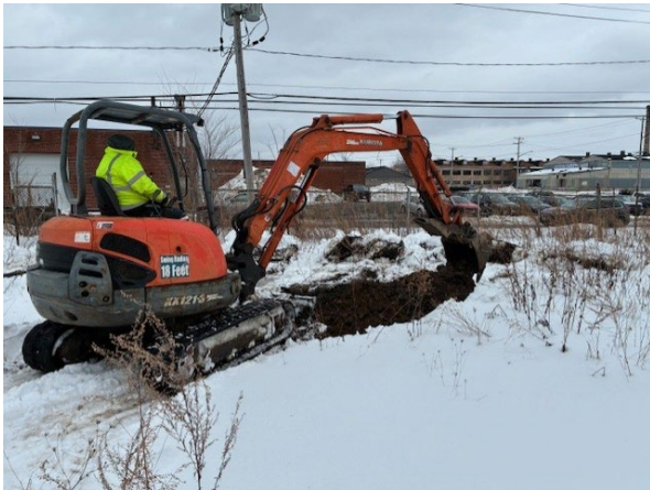
15. Test pit 8 location.
