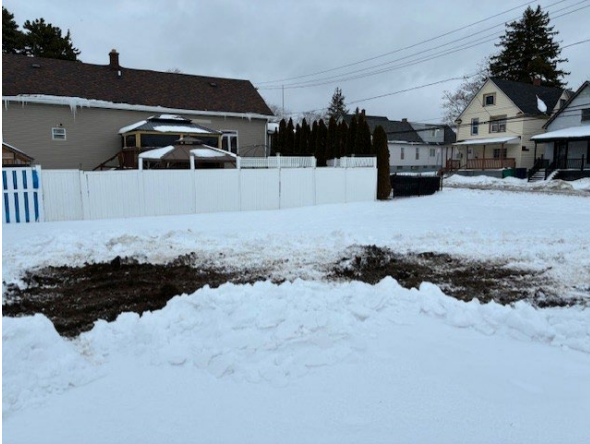
1. Test pit 1 location.
