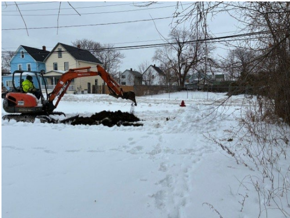
7. Test pit 4 location.
