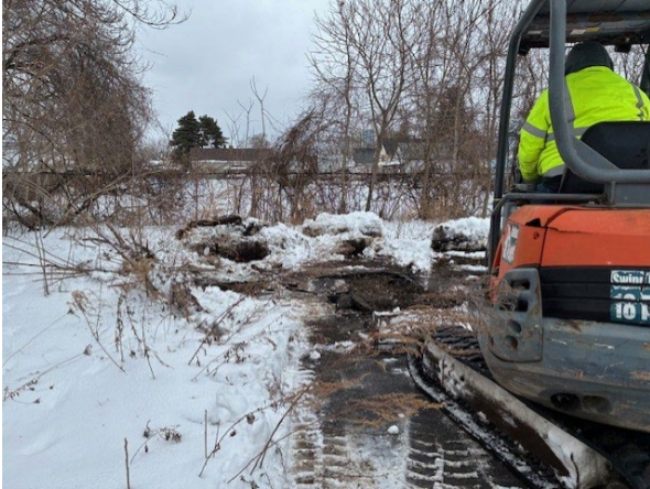
9. Test pit 5 location.
