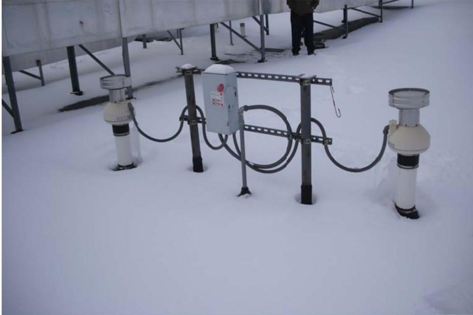
Photograph No. 5 – Sub-slab Depressurization System discharge vents and blowers.
