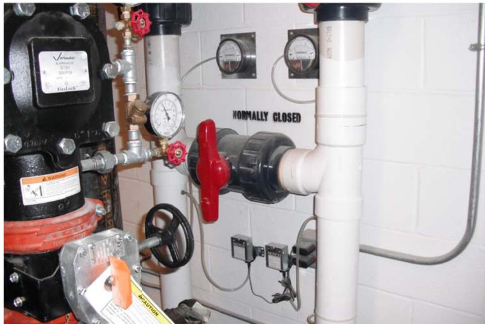
Photograph No. 4 – Sub-slab Depressurization System in basement, depicting alarms, pressure gauges and stack discharge piping.
