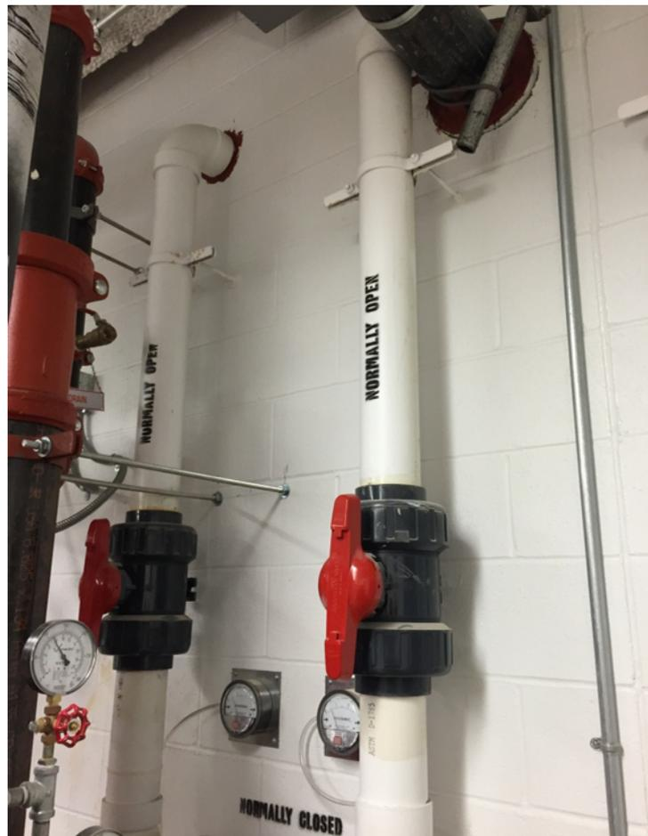
Photograph No. 4 – Sub-slab Depressurization System in basement, depicting pressure gauges and stack discharge piping.
