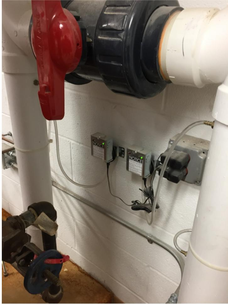
Photograph No. 5 – Sub-slab Depressurization System in basement, depicting alarms and stack discharge piping.
