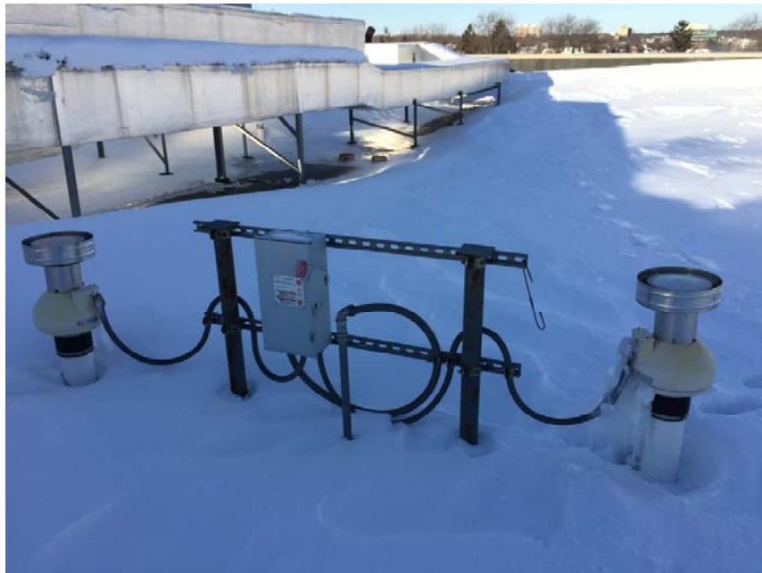
Photograph No. 6 – Sub-slab Depressurization System discharge vents and blowers and power control for discharge vents.
