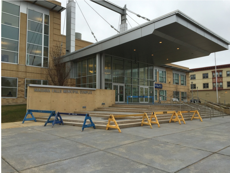
Photograph No. 1 – Exterior of Niagara Falls Municipal Complex Building, west side.
