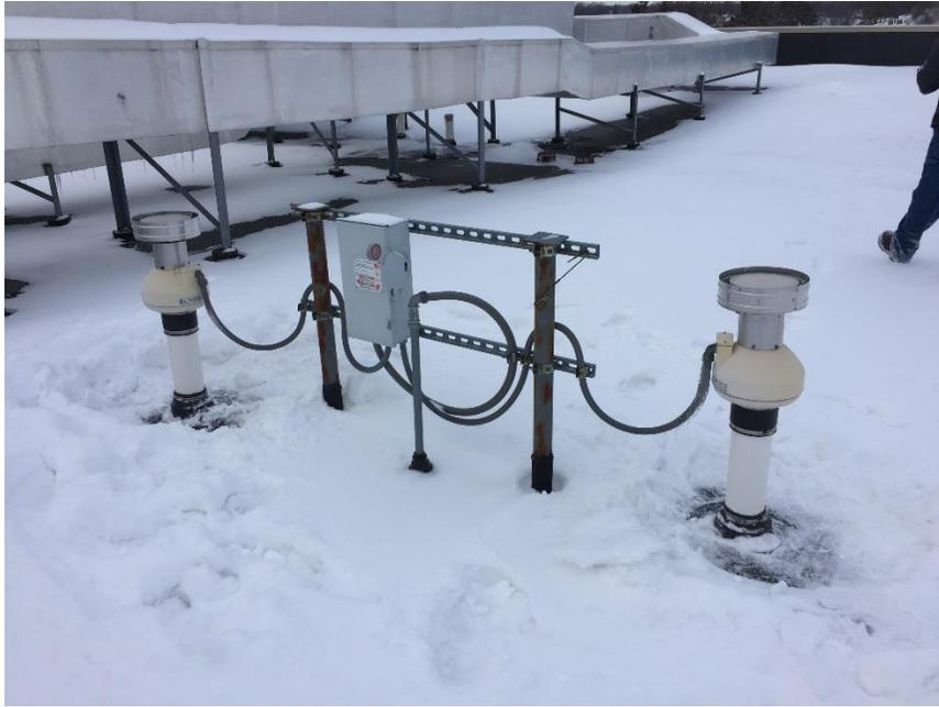
Photograph No. 9 – Sub-slab Depressurization System discharge vents and blowers and power control for discharge vents.
