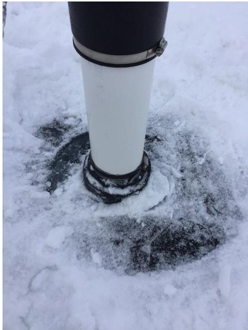
Photograph No. 14 – Roof penetration of northern discharge vent.
