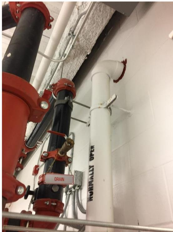
Photograph No. 4 – Sub-slab Depressurization System in basement, depicting stack discharge piping.
