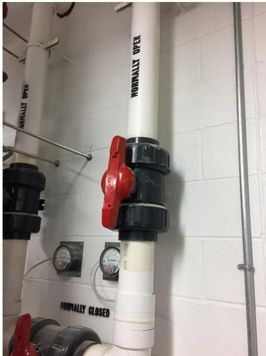
Photograph No. 3 – Sub-slab Depressurization System in basement, depicting stack discharge piping.
