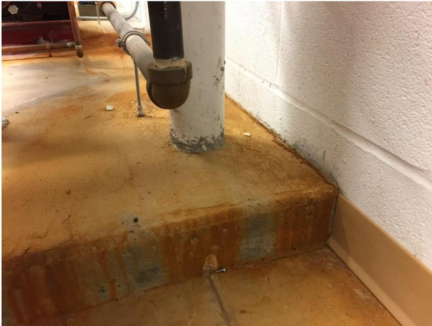
Photograph No. 6 – Sub-slab Depressurization System in basement, depicting stack discharge piping floor penetration.
