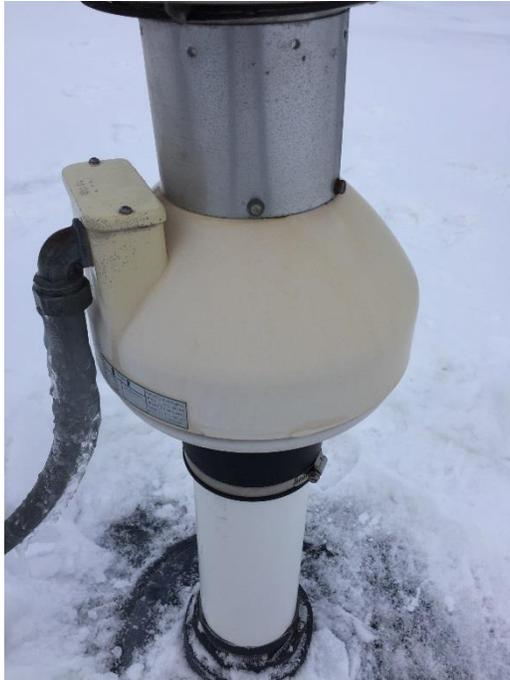
Photograph No. 15 – Close-up of northern discharge blower.
