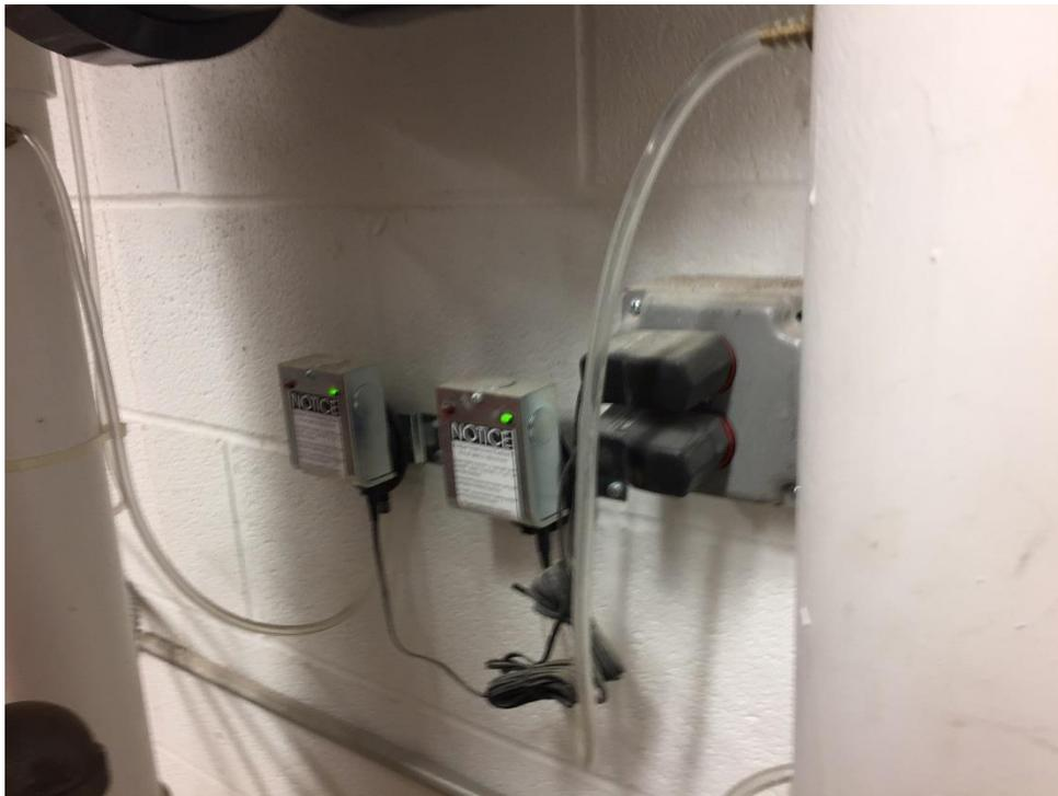
Photograph No. 2 – Sub-slab Depressurization System in basement, depicting alarms.
