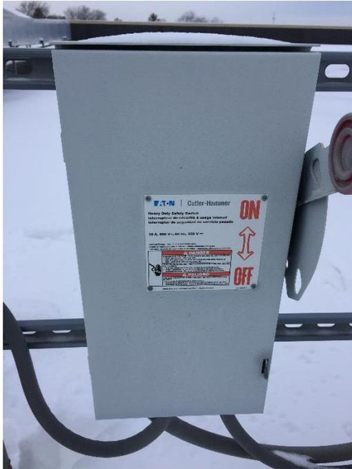
Photograph No. 13 – Sub-slab Depressurization System power control panel.
