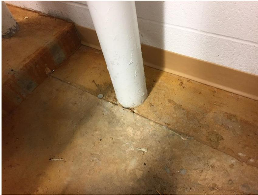
Photograph No. 5 – Sub-slab Depressurization System in basement, depicting stack discharge piping floor penetration.
