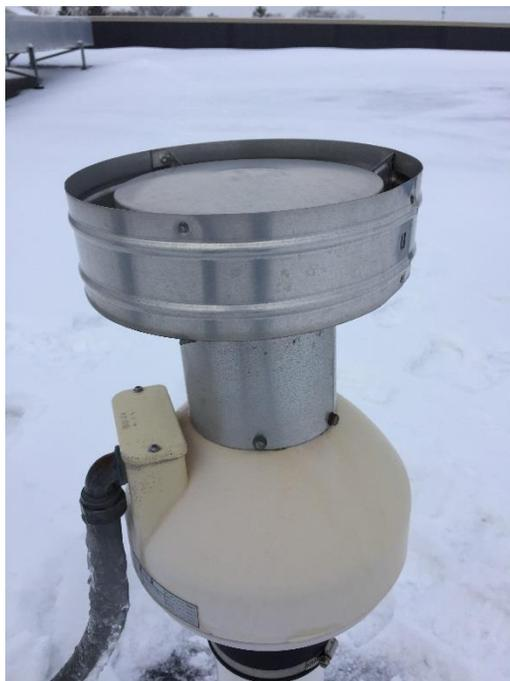
Photograph No. 16 – Close-up of northern discharge vent.
