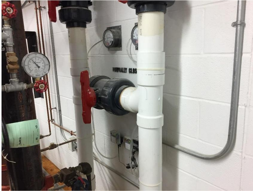
Photograph No. 7 – Sub-slab Depressurization System in basement, depicting alarms and stack discharge piping.
