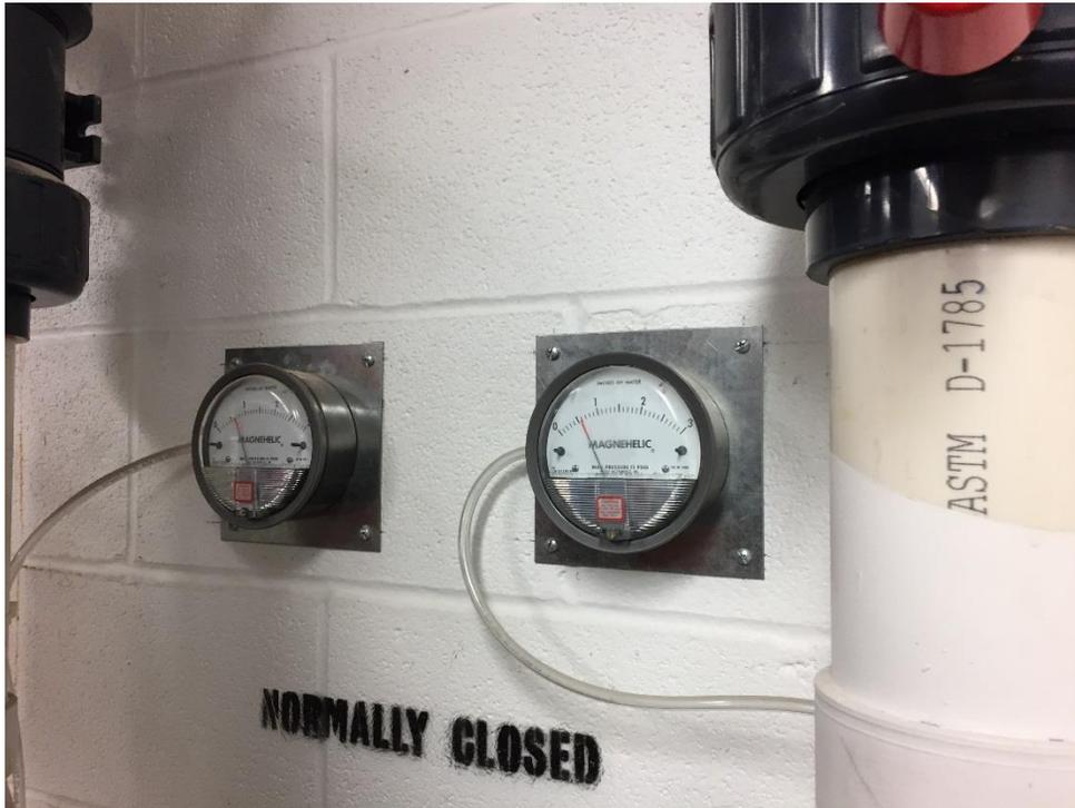
Photograph No. 1 – Sub-slab Depressurization System in basement, depicting pressure gauges.
