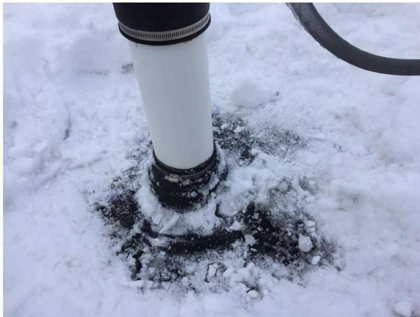
Photograph No. 10 – Roof penetration of southern discharge vent.
