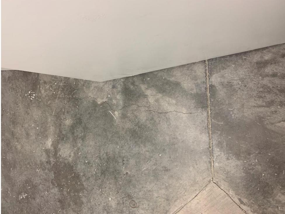
Photograph No. 6 – Minor crack in concrete floor in jail side hallway of the inmate visiting area of the jail.
