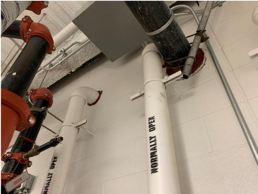
Photograph No. 4 – Sub-slab Depressurization System in basement, depicting stack discharge piping.
