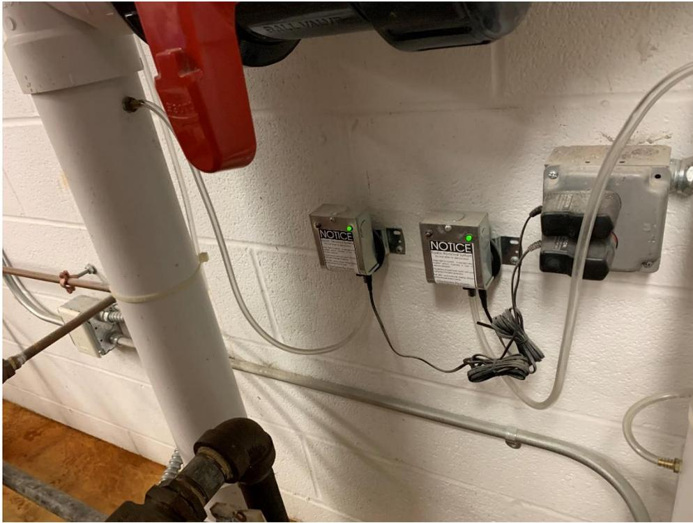
Photograph No. 3 – Sub-slab Depressurization System in basement, depicting alarms.
