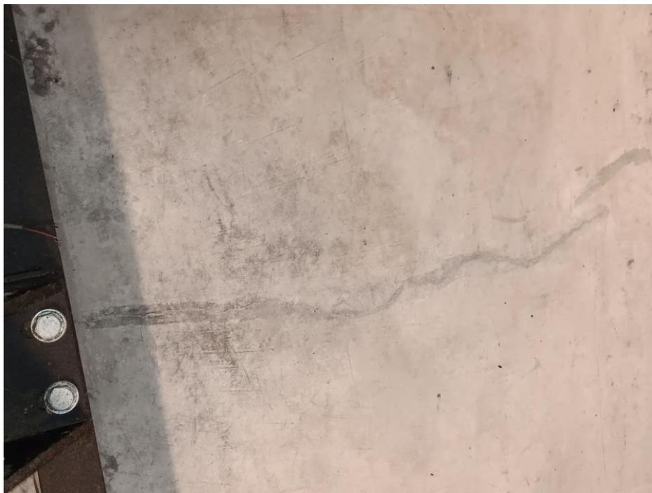
Photograph No. 11 – 2023 Repaired (caulked) crack in concrete floor in Room B-37 (i.e. elevator shaft room).
