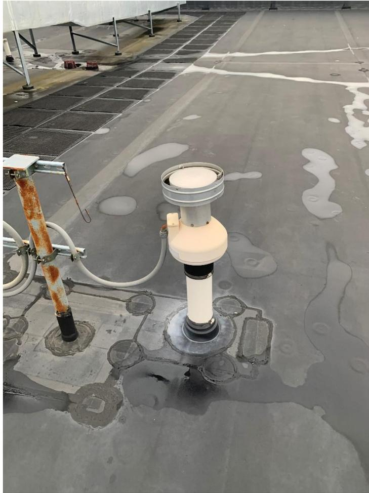
Photograph No. 10 – Roof penetration of northern discharge vent.
