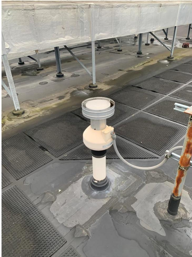
Photograph No. 9 – Roof penetration of southern discharge vent.
