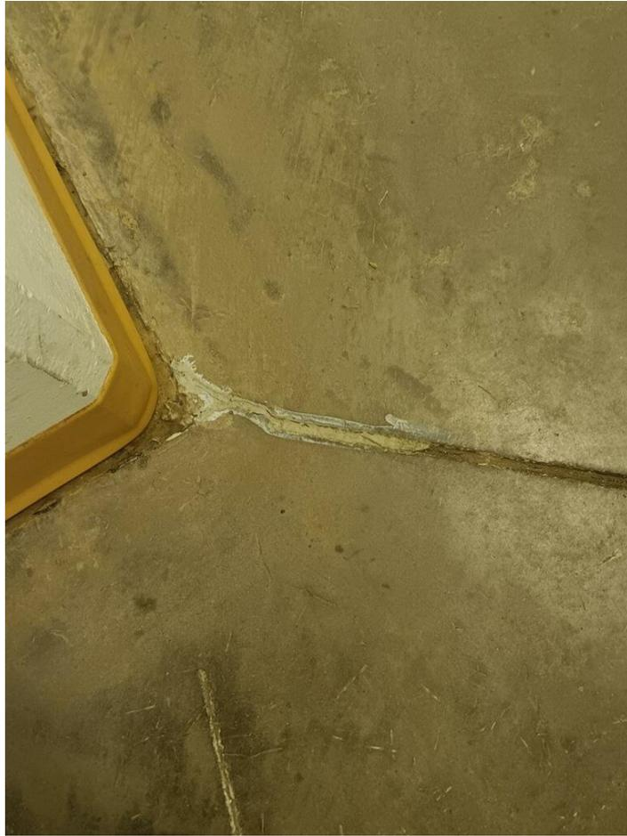
Photograph No. 13 – 2022 Repaired (caulked) crack in concrete floor in men's jail.
