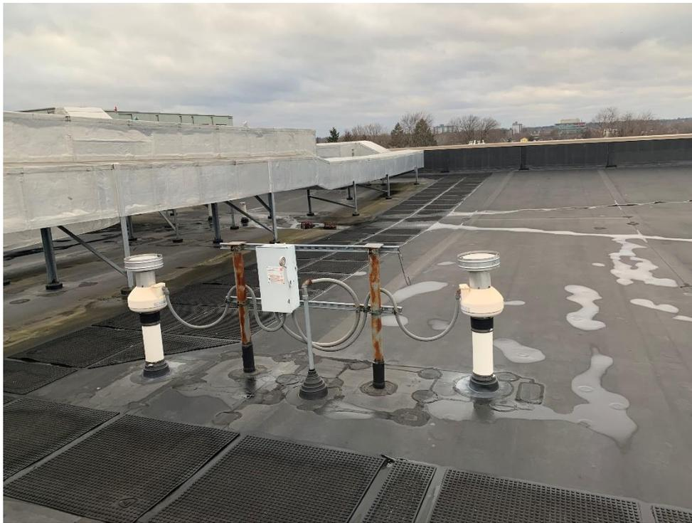
Photograph No. 8 – Sub-slab Depressurization System discharge vents and blowers and power control for discharge vents.
