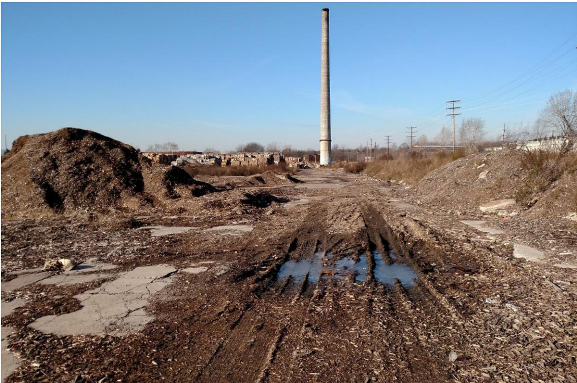
Photo #2 - View of on-Site rutting and cracking in concrete/asphalt.
