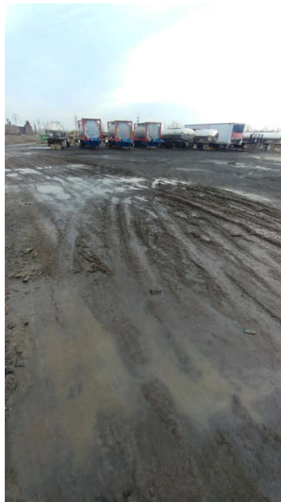
Photos #12 & 13: Additional rutting in high traffic areas.
