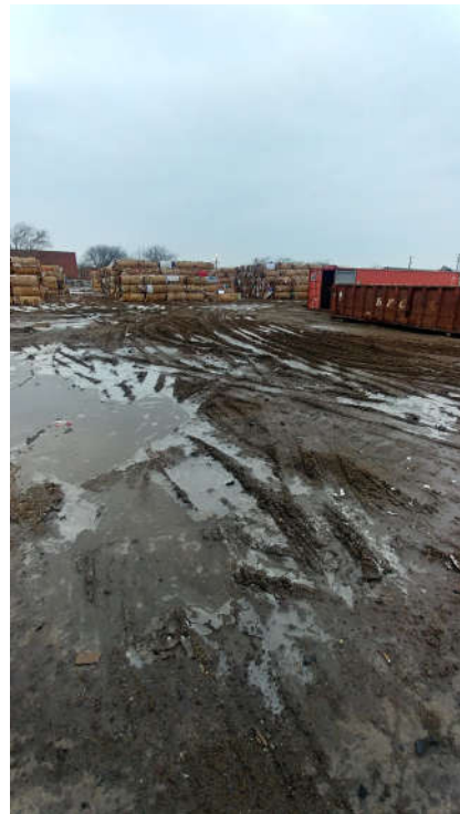
Photos #8 & 9: Rutting/ponding on southwest portion of the Site.
