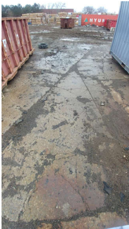
Photos #16 & 17: Areas of cracking concrete.
