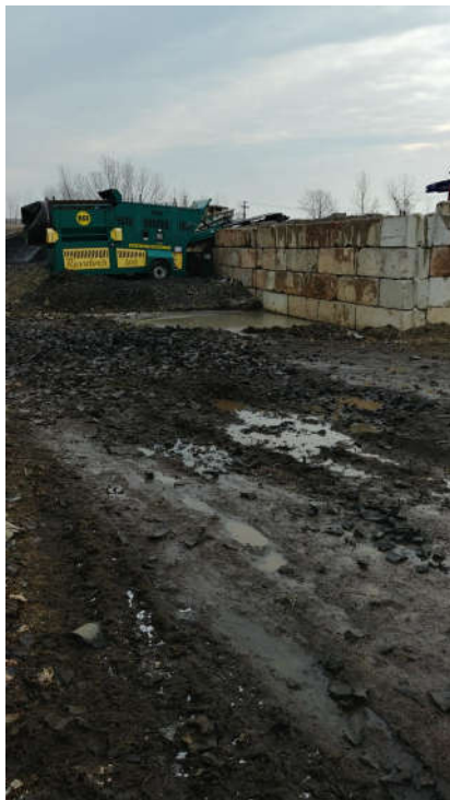
Photos #12 & 13: Additional rutting in high traffic areas.
