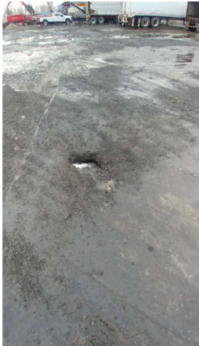
Photos #10 & 11: Small sinkhole penetrating cover system (left). Separation of cover system at smokestack base (right).
