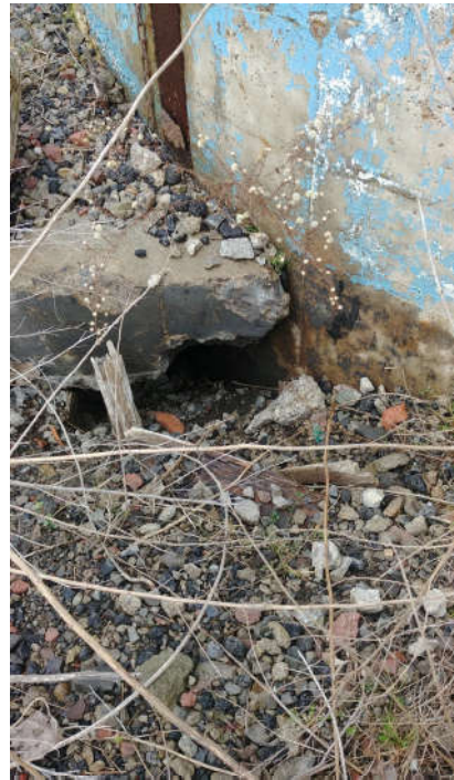
Photos #10 & 11: Small sinkhole penetrating cover system (left). Separation of cover system at smokestack base (right).
