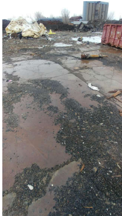
Photos #16 & 17: Areas of cracking concrete.
