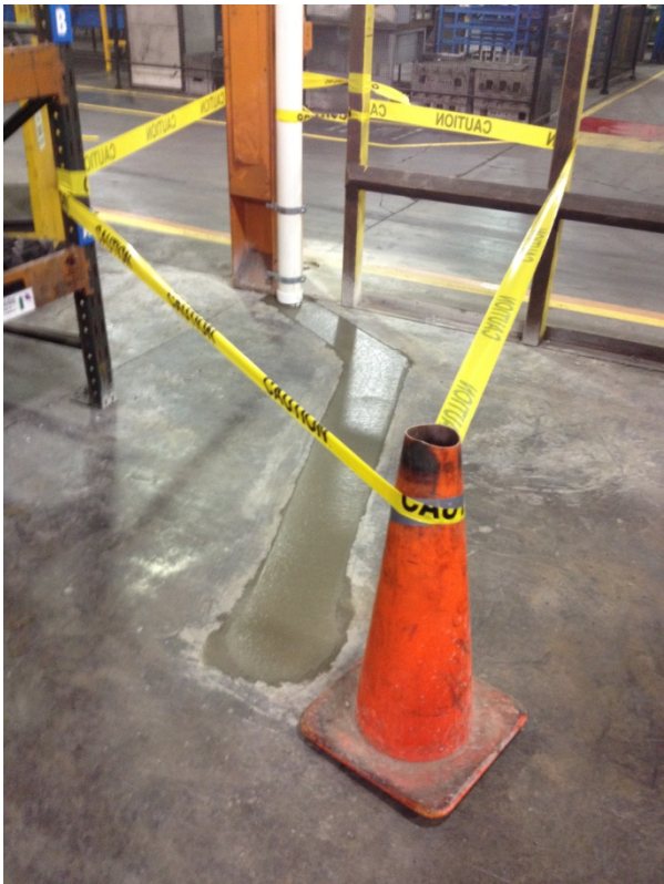
Bldg 7 East – Completed suction pit
