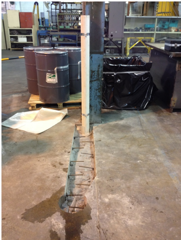
Bldg 8 – Construction of suction pit
