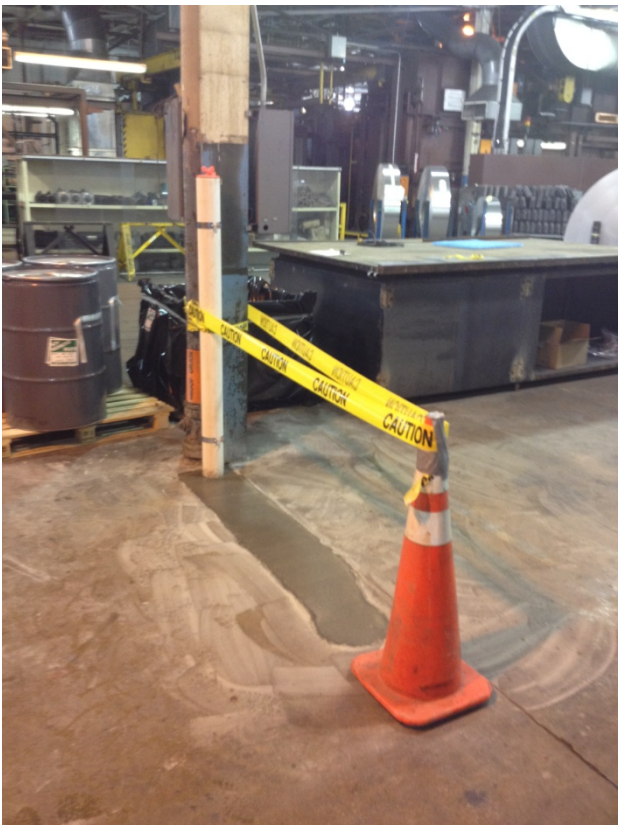
Bldg 8 – Completed suction pit
