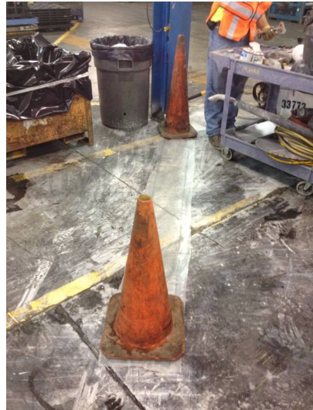
Bldg 7 West – Completed suction pit
