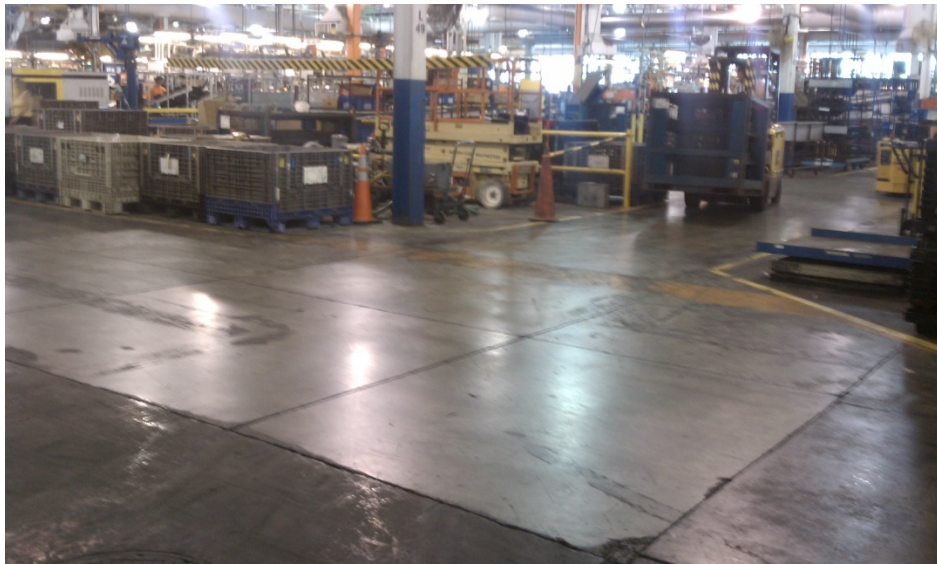
Bldg 7-West Concrete Floor with Cracks and Seams
