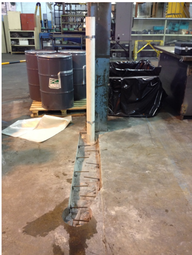
Bldg 8 – Construction of suction pit
