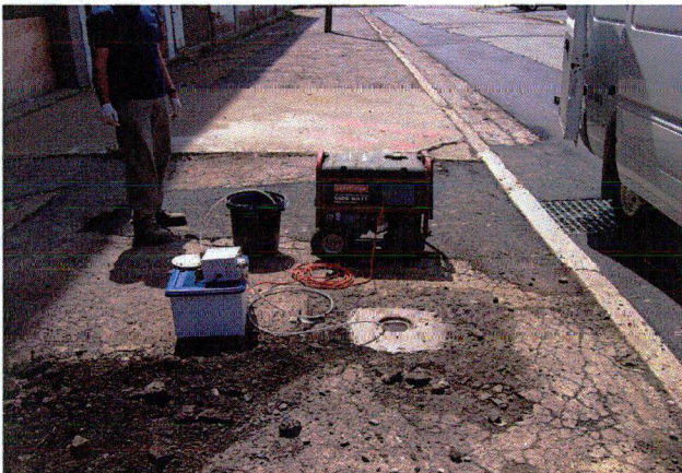
Photograph 9. Developing well at RR-MW-04
