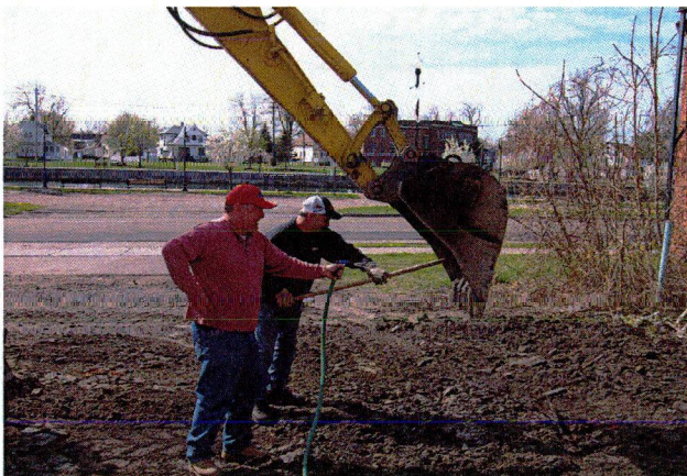
Photograph 11. Decon of the excavator bucket after RR-TP-01
