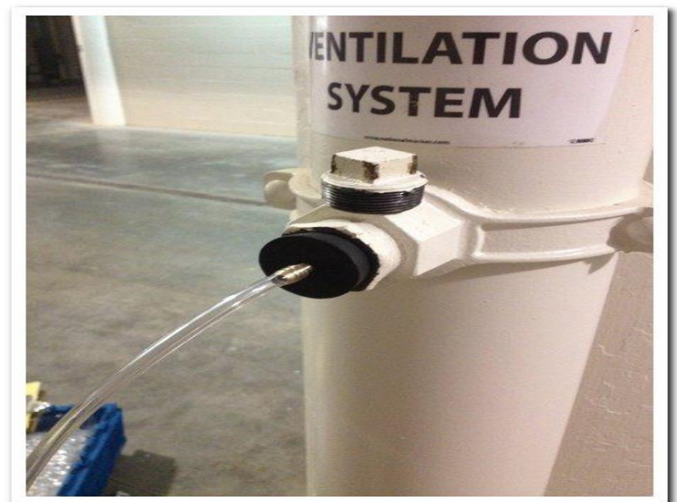
4. Vent Port Vapor Sampling
