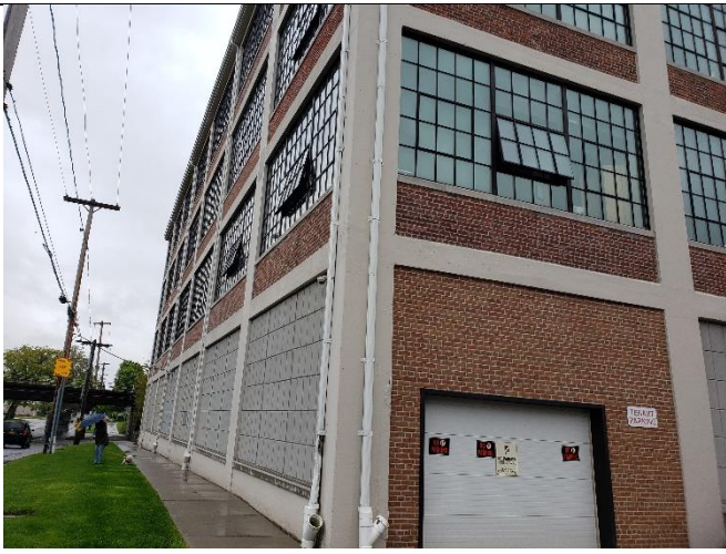
North exterior Site Building
