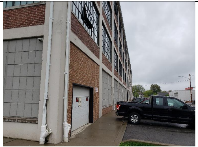
West exterior Site Building
