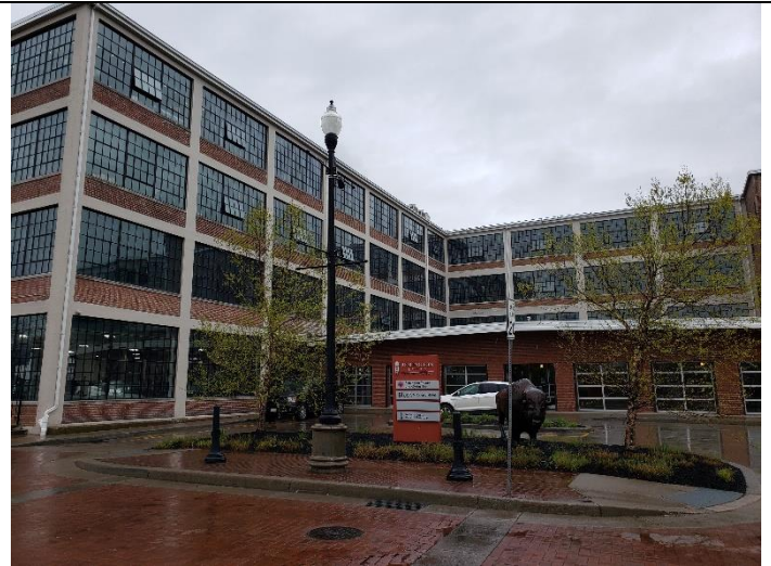
South exterior Site Building
