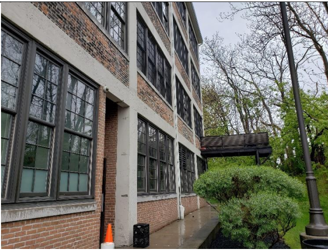
East exterior Site Building
