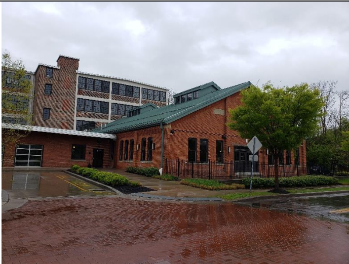
South exterior Site Building
