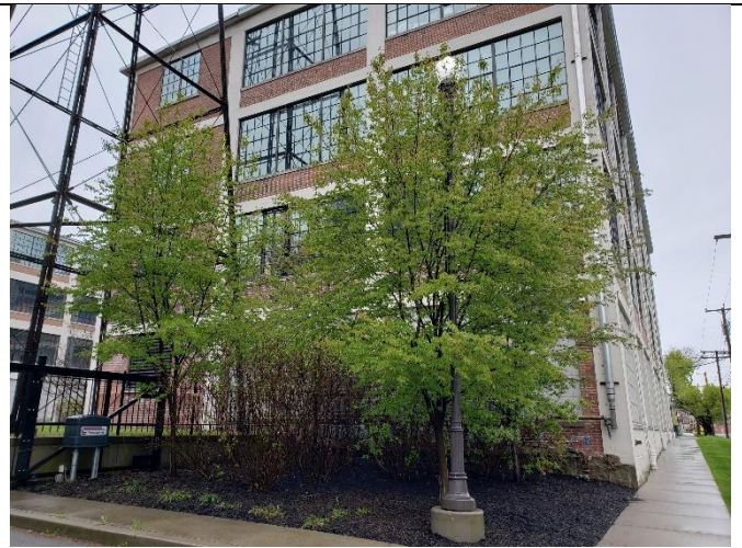
East exterior Site Building
