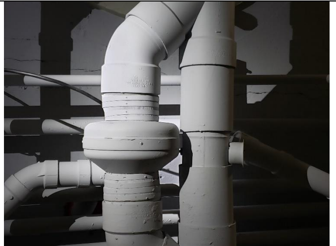
Active fan associated with SSDS system
