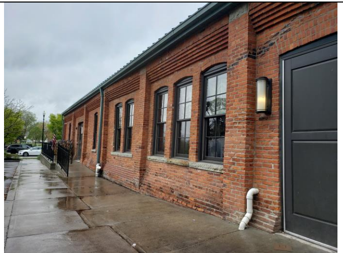
East exterior Site Building
