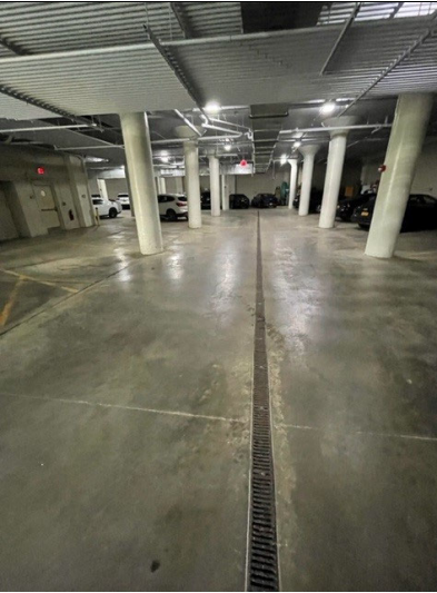
Western portion of parking garage
