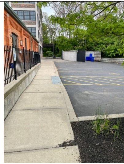
East exterior Site Building
