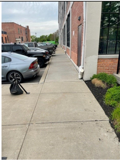
West exterior Site Building
