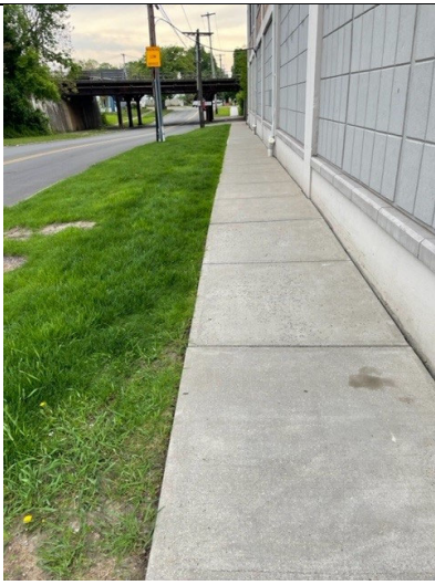
North exterior Site Building
