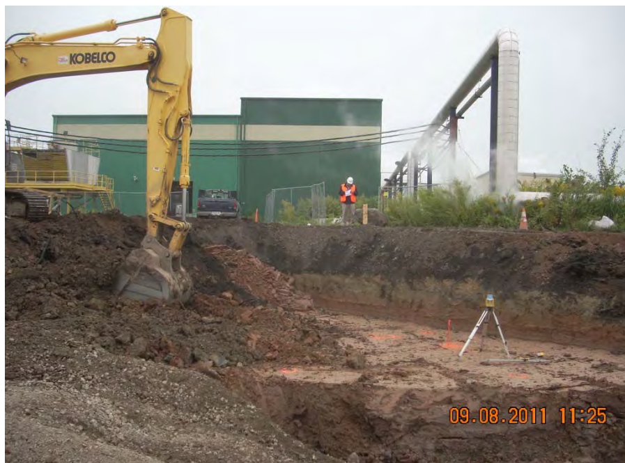
Photo 12: View looking north towards excavation area with laser level used to check excavation elevations. ERM personnel were present to screen for contamination and GRD personnel were present to screen for RAD material (date: 09/08/2011).
