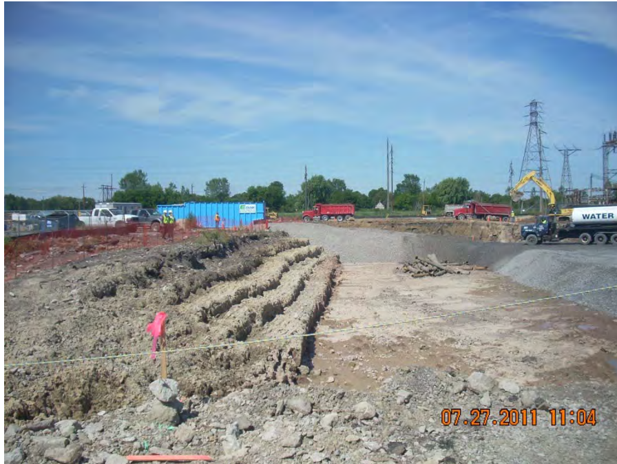
Photo 9: View looking east towards the benched excavation area. Pipes were encountered during excavation and went off-site as contaminated material, and water trucks were used to control dust (date: 07/27/2011).
