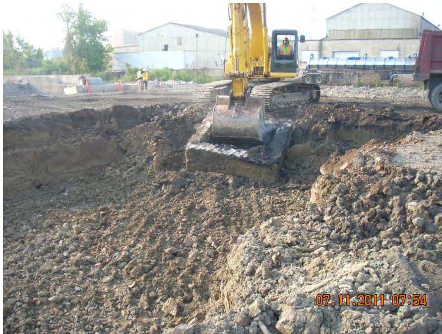
Photo 5: View looking south towards excavation area. Remnants of old building foundations were locally encountered and excavated (date: 07/11/2011).
