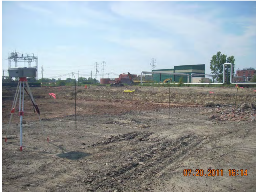
Photo 7: View looking northeast towards excavation area. Community air monitoring equipment is set-up at the excavation extents and areas are marked off prior to backfill (date: 07/20/2011).
