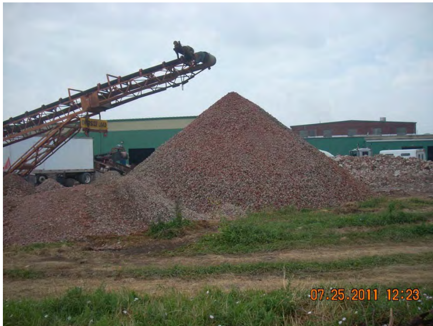
Photo 8: View looking east towards crushed brick piles from demolished building material which was sampled to evaluate potential reuse at the site (date: 07/25/2011).
