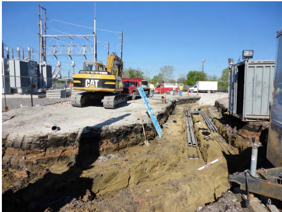
Photo 18: View looking east towards excavation area for utility installation. Soil stratigraphy with black historic fill at the top underlain by yellow-brown sandy silt layers is observed (date: 05/11/2012).
