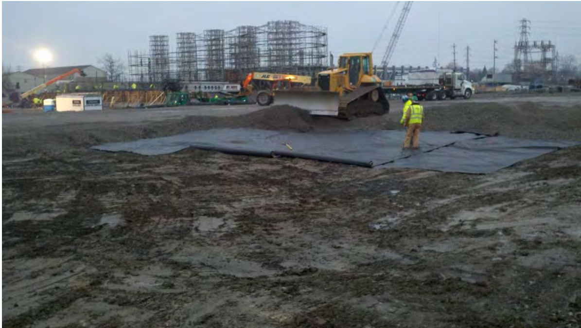
Photo 15: View looking northeast towards excavated area being backfilled with clean stone (date: 12/30/2011).
