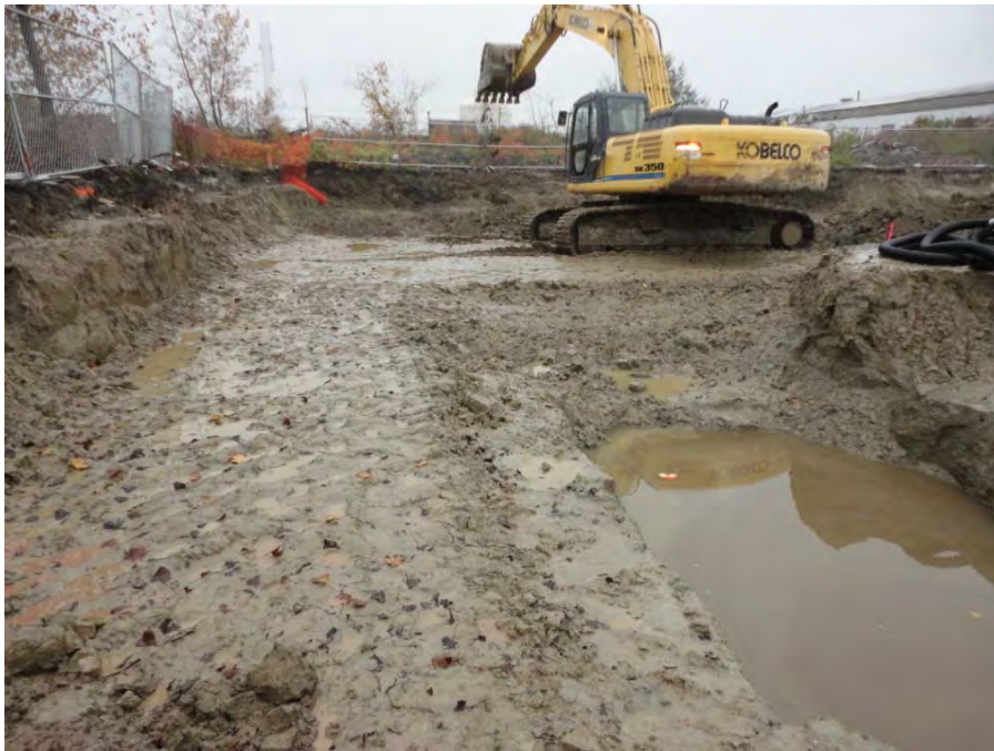
Photo 10: View looking south of the Quad 88 excavated area with RAD and VOC readings greater than action level. Water which accumulated on-site was pumped through hoses into mobile temporary storage tanks on-site for subsequent characterization as shown in Photo 9 (date: 07/27/2011).
