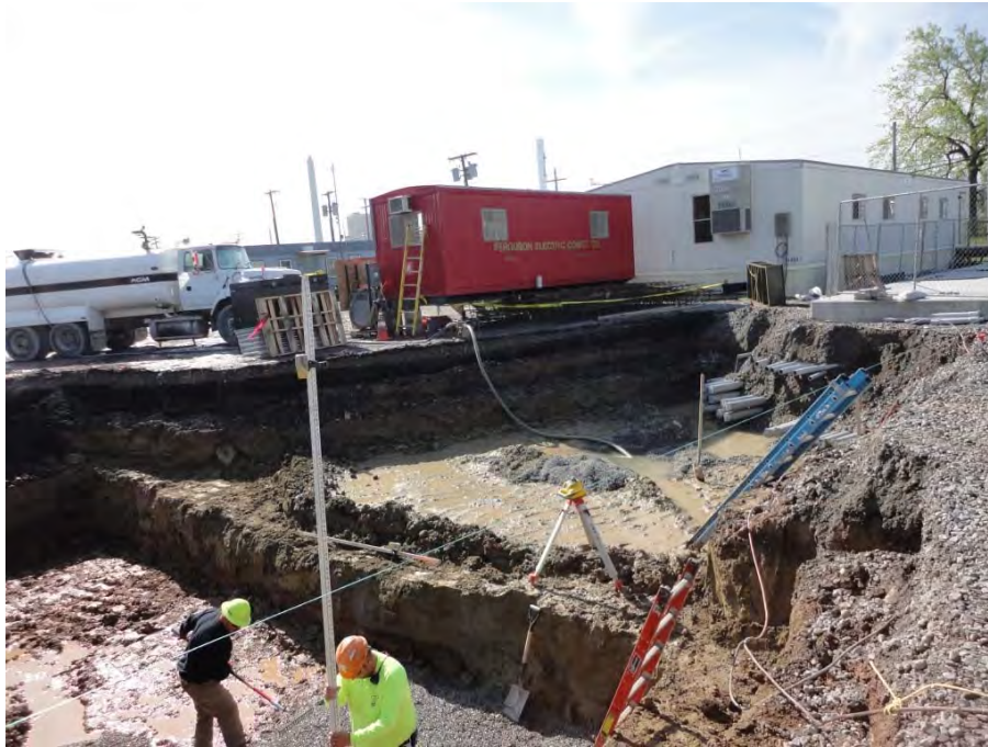
Photo 17: View looking south towards excavated area for utility installation being backfilled with clean stone. Rain accumulated on site is pumped into a holding tank and discharged back onto site (date: 05/09/2012).
