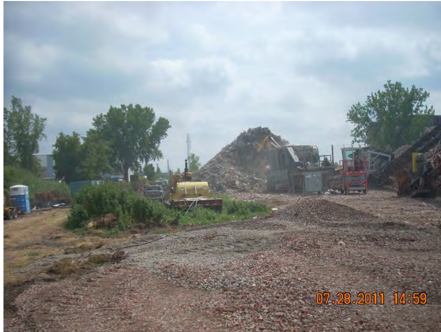
Photo 11: View looking south towards crushed concrete and brick piles. Crushed brick was temporarily used to pave roads. Crushed concrete was approved by NYSDEC and used as backfill on-site (date: 07/28/11).
