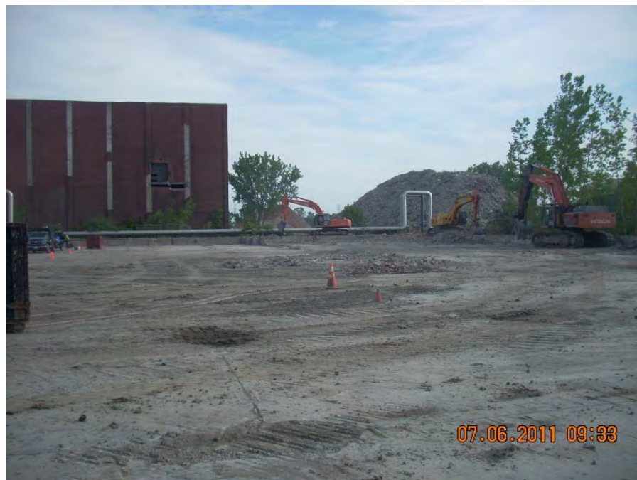
Photo 4: View looking north towards the crushed concrete piles from demolished building material which were sampled for laboratory analyses to evaluate potential reuse on site (date: 07/06/2011).
