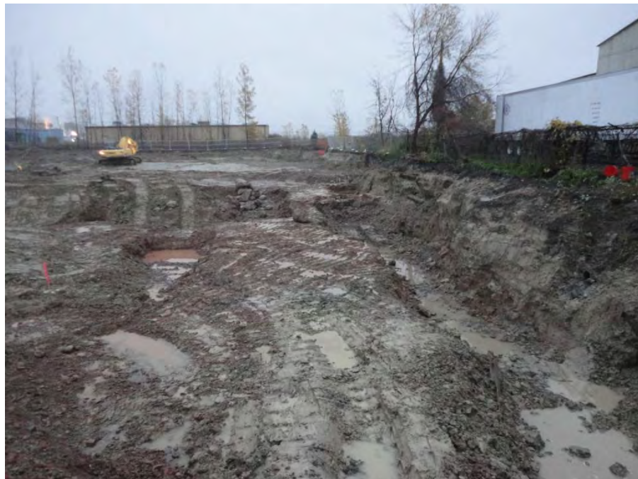
Photo 14: View looking west towards Phase 3 excavation area. Clean soil was reused onsite as backfilling in some excavated areas (date: 10/26/2011).
