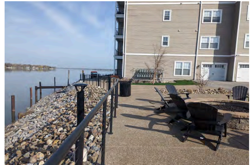
4. Southwest corner facing north
