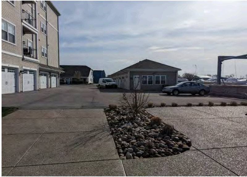
5. Southwest corner facing east
