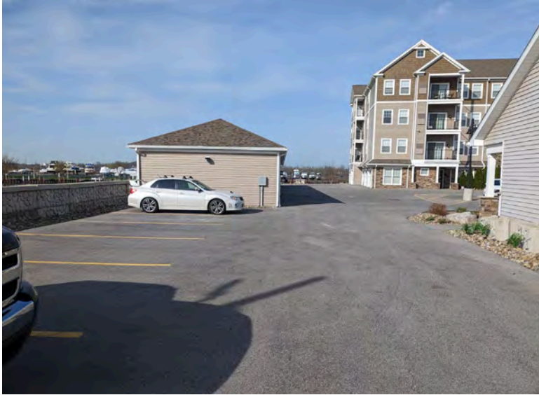
1. 600 River Rd. property southeast border facing west
