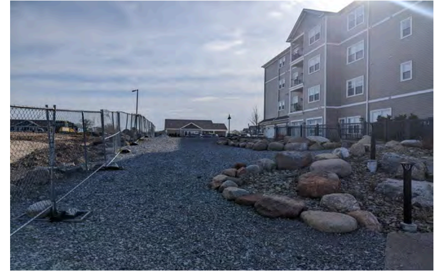
10. Northwest facing east
