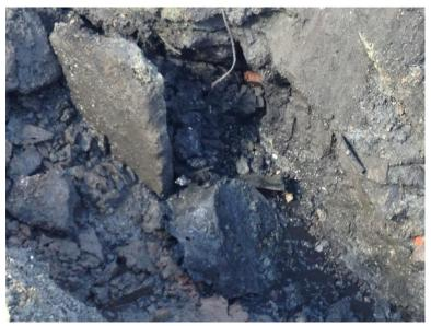
Photo 1: Remains of a 55-gallon drum encountered in the water utility line excavation facing southwest
