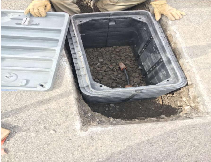
Photo 5: New vault installed over repaired communications line.
