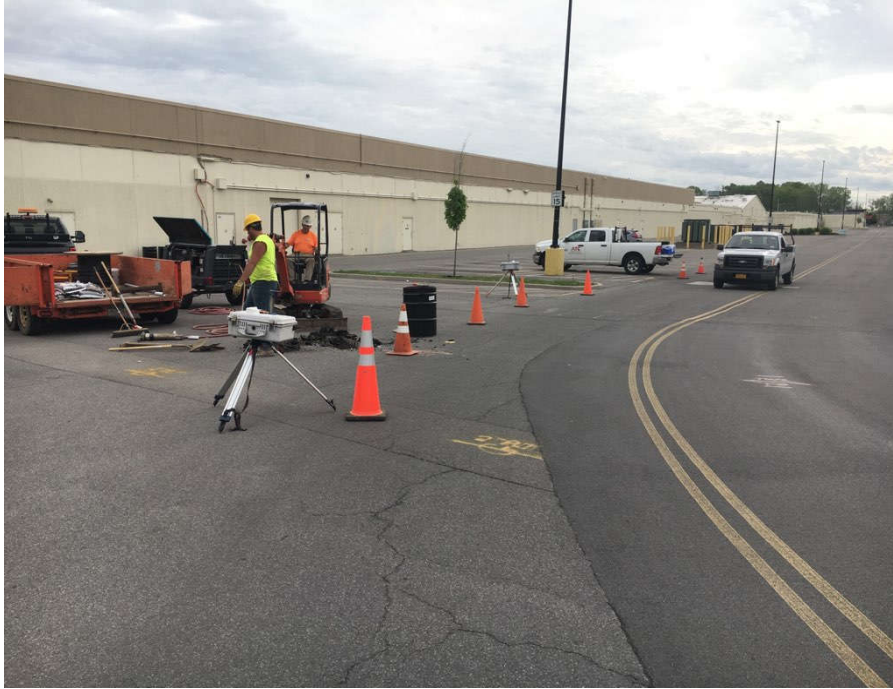
Photo 1: Work zone perimeter with two air monitoring stations set up.
