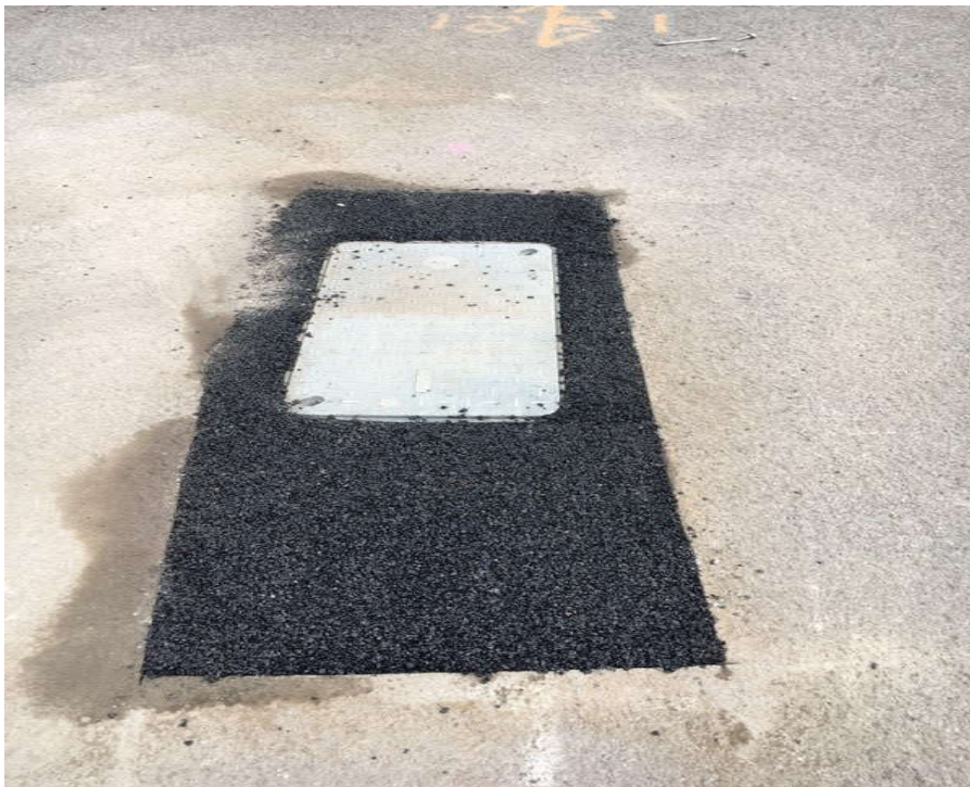
Photo 6: Excavated area with new vault backfilled and completed with blacktop.
