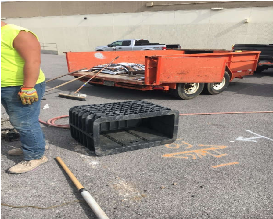
Photo 4: New vault to be installed over the repaired communications line.
