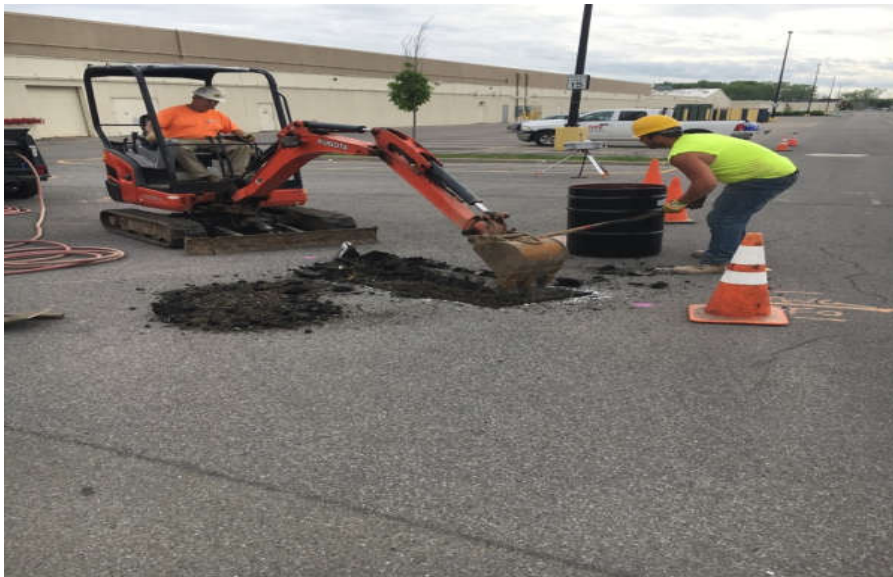
Photo 2: Beginning of excavation for the damaged communications line.
