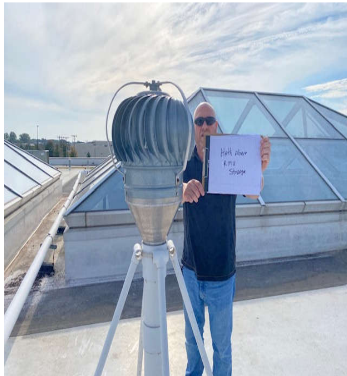
Photo 8: Outlet fan near Hatch above RMU Storage.
