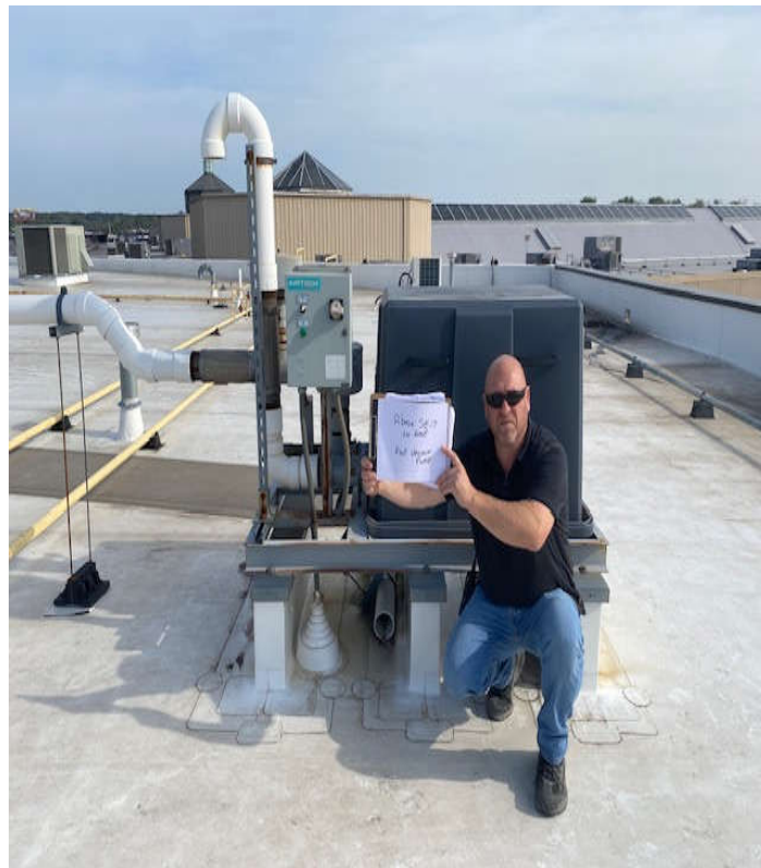
Photo 10: This is the SVE pump above SE-7 on roof. It was not operating.
