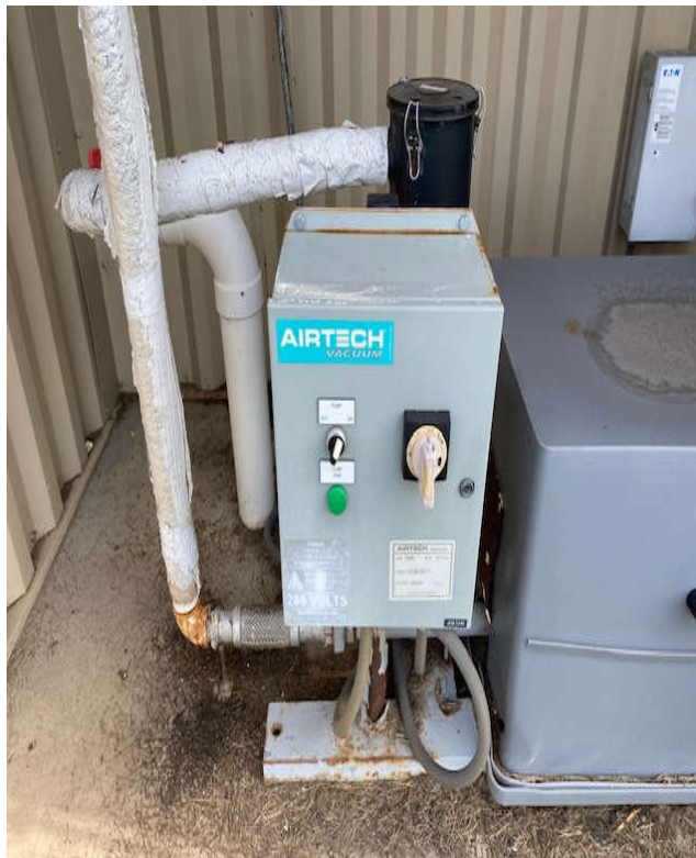
Photo 19: Control panel of the SVE system at the Extra Space Storage Building.
