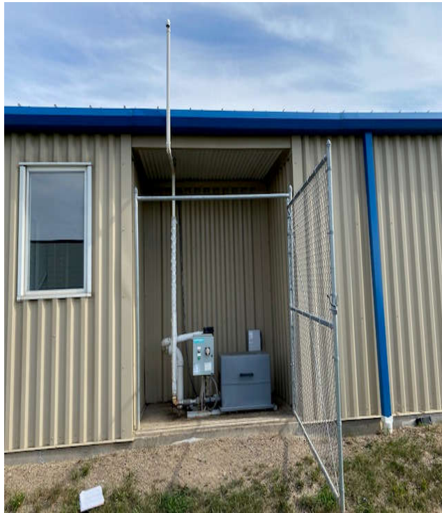
Photo 15: SVE system at the Extra Space Storage Building.
