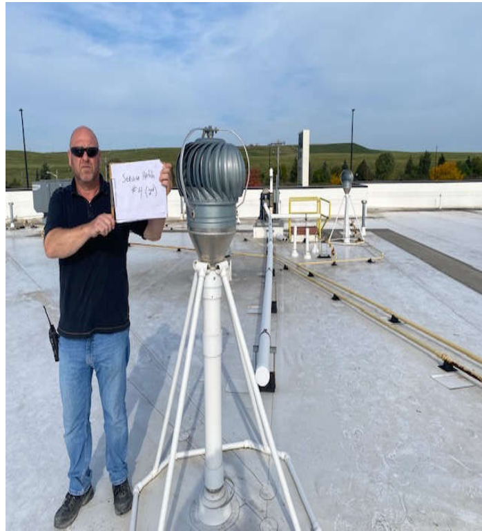
Photo 7: Second outlet fan near Service Hatch #4.
