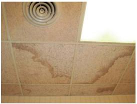
Minimal water damage on ceiling tiles within Site building
