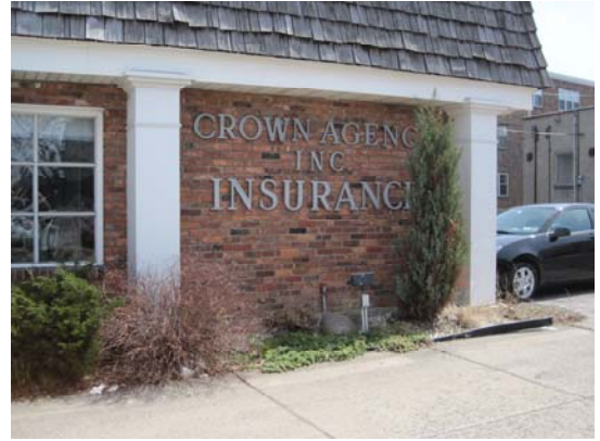
Site building looking east
