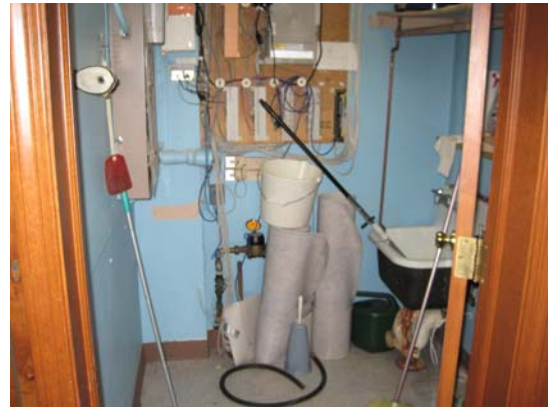
Janitorial closet within Site building
