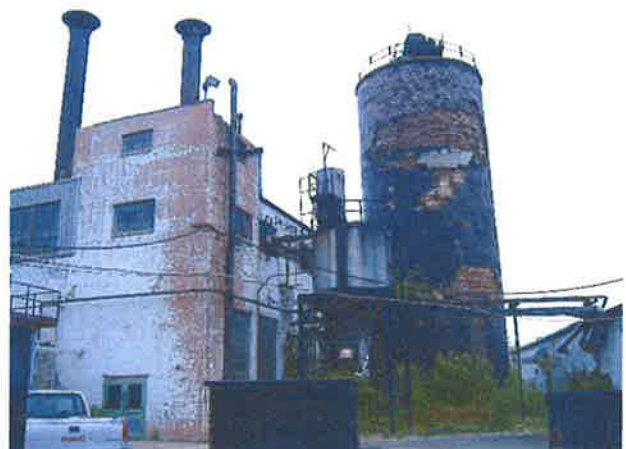
Boiler Building, coal storage silo, and fly ash hopper.
