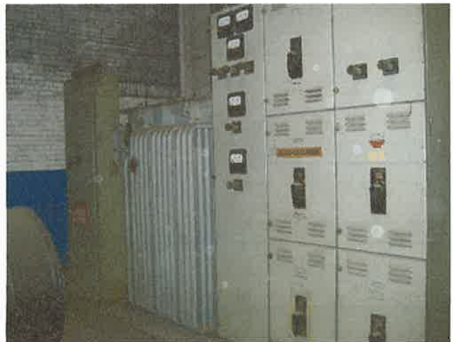
One of two PCB containing transformers located in a room within Building W, facing northeast.
