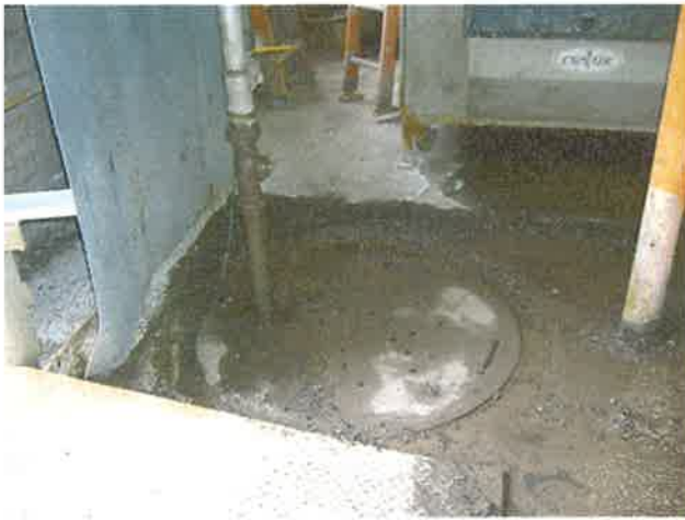
Sump pit with pump in south end of Building J-2. Water noted on floor from recycling process.
