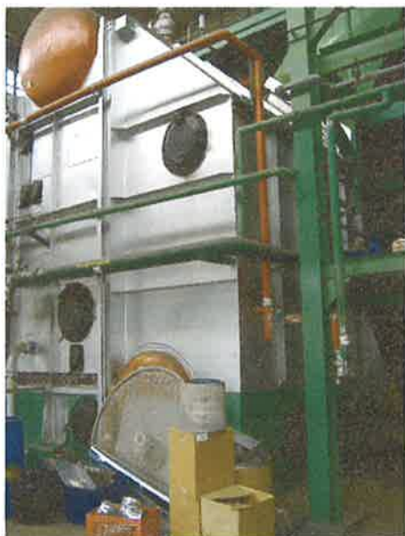
Boiler, no longer in use. Note asbestos wrapped piping.
