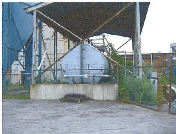
Formerly used above ground storage tank, located north of Building X, facing south. Stored naphthetic oil used for rubber compression molding.
