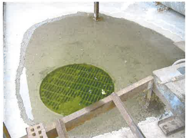
Sump pit below chip/storage bins. Previously oil storage area required this sump. Now just used to collect storm water (e.g. rain water).
