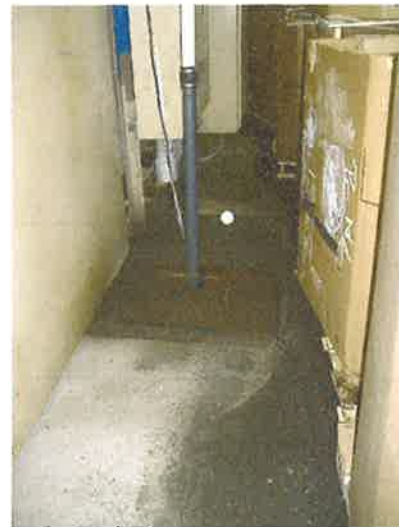
All floor drains in extrusion room located in north end of building J-2 go to this central pit, facing south. From pit, fluid goes to holding tank. Fluid used for make-up water in chip recycling processing room.
