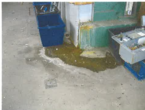
Water leak from overhead pipe in boiler room. Leaking water runs over asbestos covered pipes.
