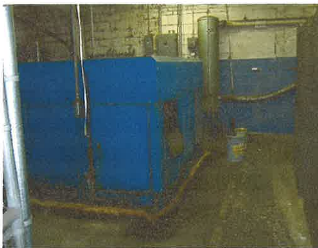
Facility backup air compressor located in Building Q, facing east. Oil noted on floor with oil boom placed.
