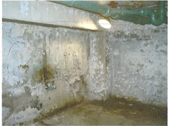
Deteriorating paint on basement walls of boiler building.
