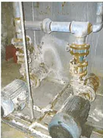
Recirculation water pumps and tank in boiler building basement.
