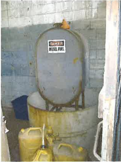
Diesel fuel AST in former Bushing Dip Room.
