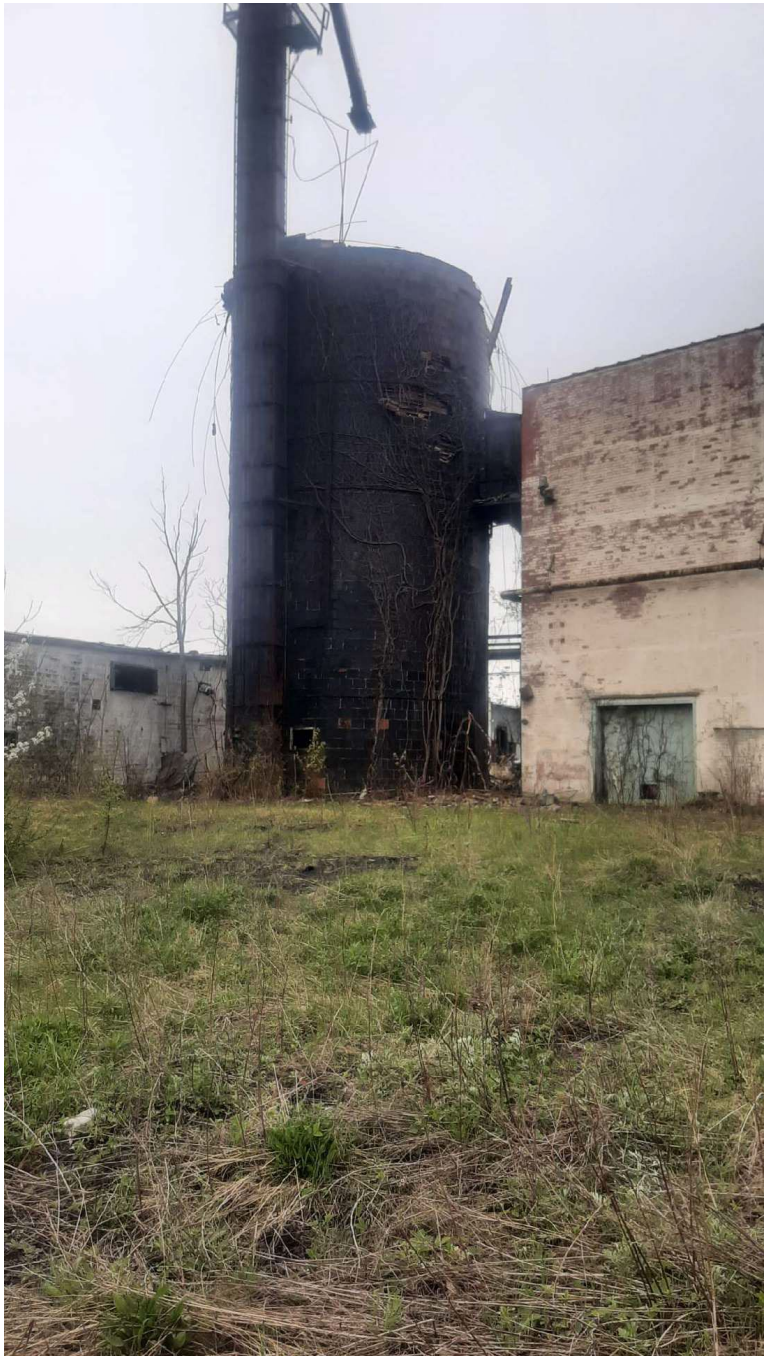
Figure 3. Former Coal Storage Silo
