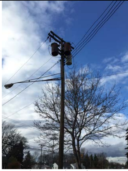
Pole-mounted transformers
