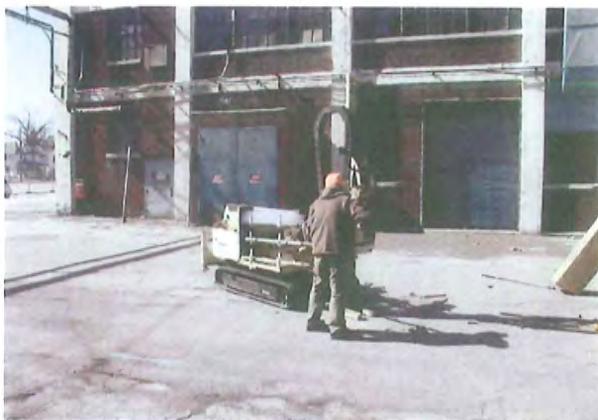
Photograph 3. Location of CS-BH-05, facing west and Building #4
