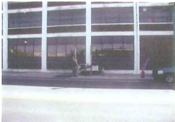
Photograph 5. Location of CS-BH-08, facing south across Walnut Street at Building #2
