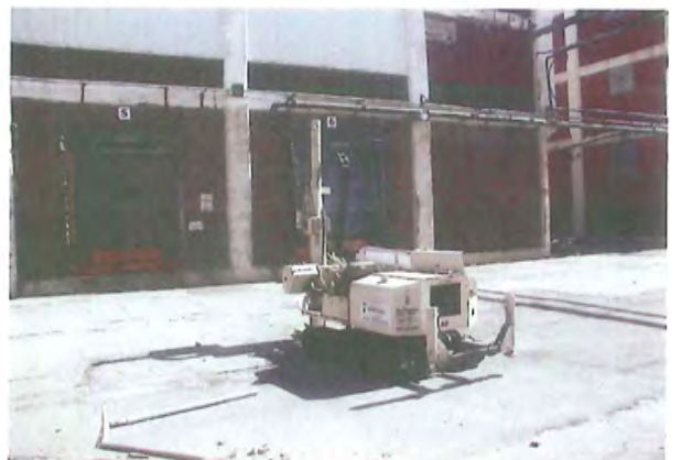
Photograph 4. Facing east, Building #2 and location of CS-BH-06
