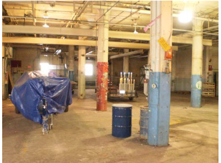
Looking south from within center of Building #4
