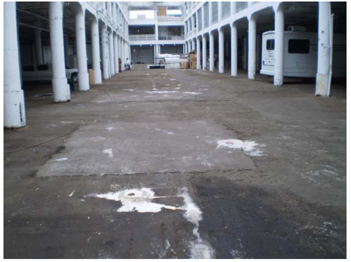
Looking west down center - inside Building #3
