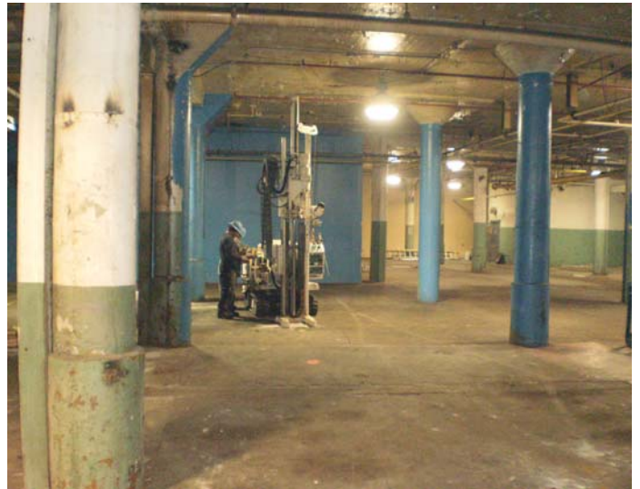
Geoprobe within south central Building #2, location B2-14
