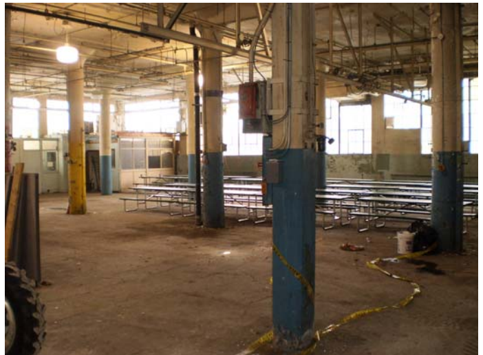
Northeastern corner of Building #4
