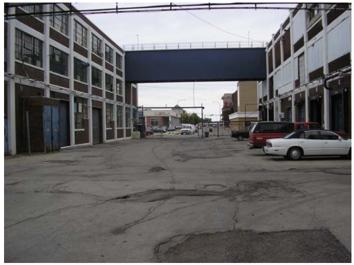
Looking north – Building #4 on left; Building #2 on right
