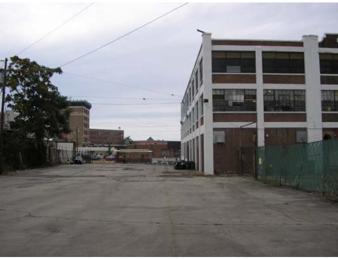
Looking north at southwest corner of Building #4
