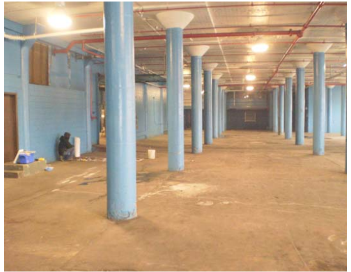
North side of Building #2 - center section – looking west
