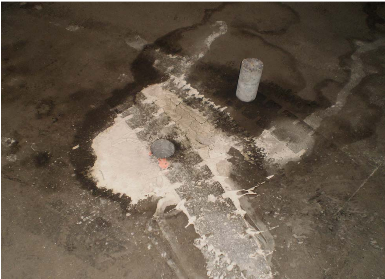
Concrete floor coring from south central portion of Building #2
