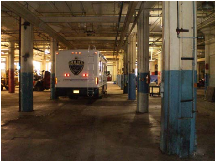
Looking east in Building #4
