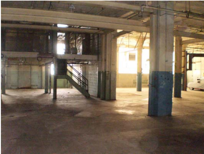
Looking north from within center of Building #4
