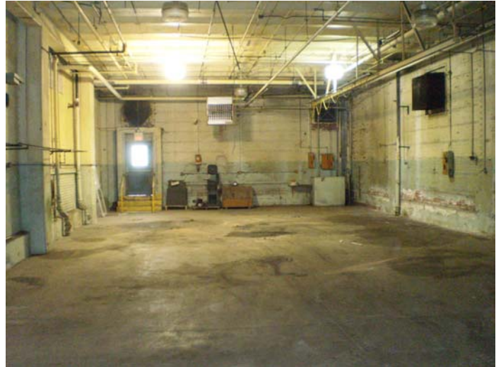
Southwestern end of Building #4
