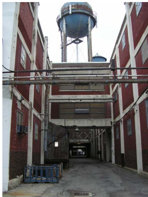
Looking east – Building #2 left; Building #3 right
