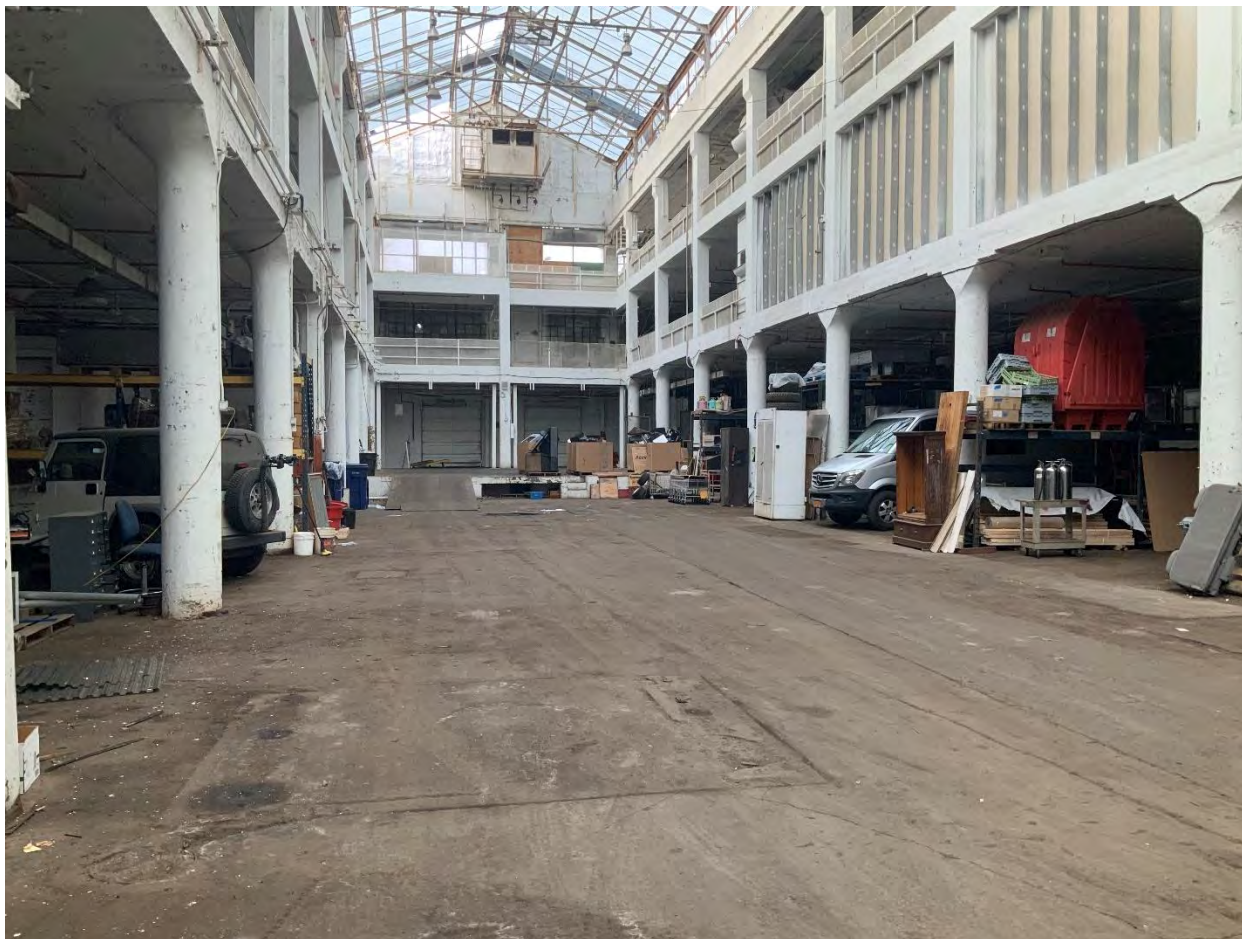
Site Photos - View of west end of building shows extent of storage preventing access
