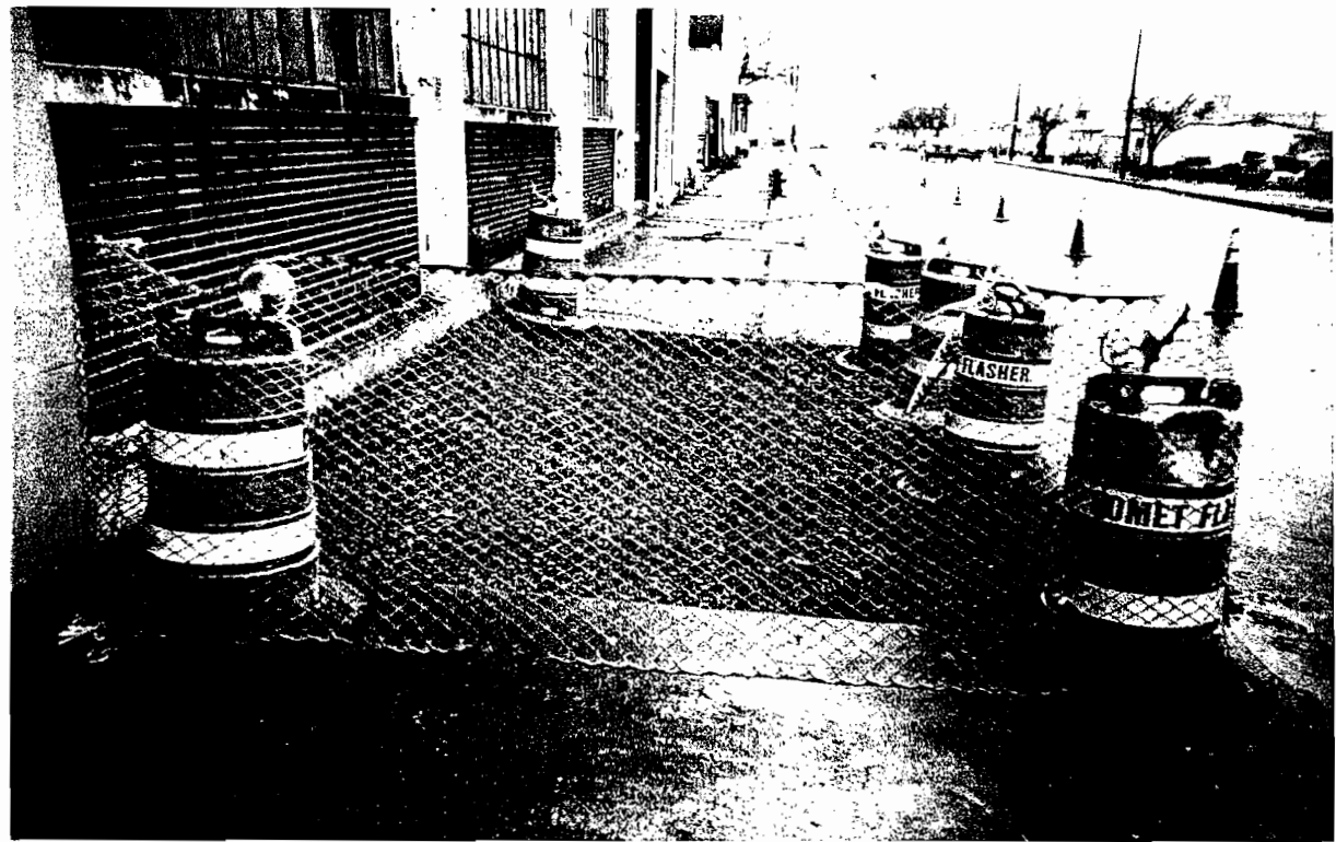
Photo #18: Bldg. #4 excavation backfilled.
