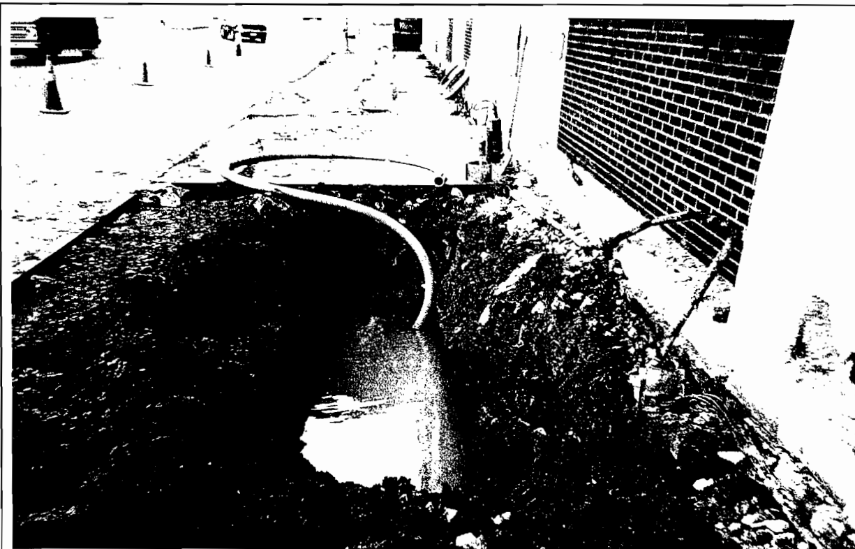
Photo #16: Bldg. #4 excavation filled with water from leaking line.
