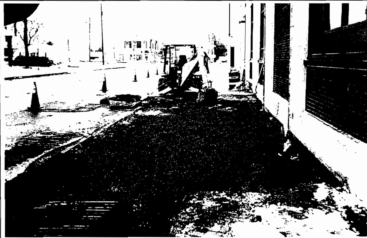
Photo #20: Bldg. #2 (T-5/T-6) excavation backfilled.
