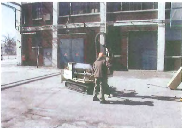
Photograph 3. Location of CS-BH-05, facing west and Building #4
