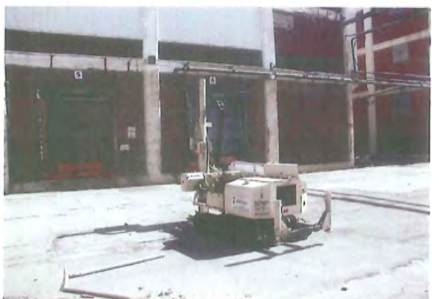
Photograph 4. Facing east, Building #2 and location of CS-BH-06
