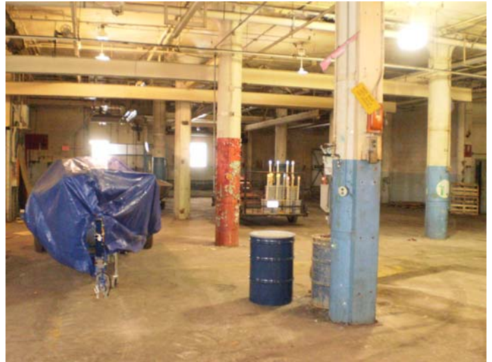
Looking south from within center of Building #4
