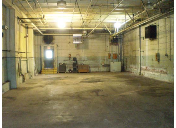
Southwestern end of Building #4
