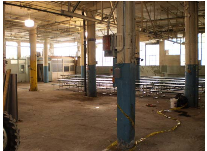
Northeastern corner of Building #4
