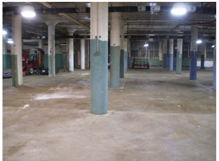
Eastern end of Building #2
