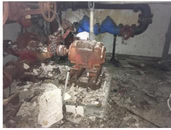
25. Old pump in utility room on first floor. Possibly containing PCB oil.
