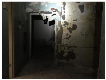
17. Seond floor former medical offices. Peeling paint, asbestos tile.
