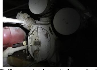
22. Old pump motor in basement boiler room. Possibly contains PCBs.
