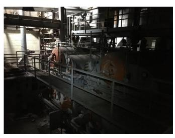
19. First floor boiler room. Asbestos lined tanks.
