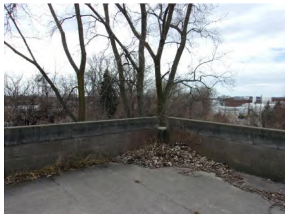
View from Property fire tower roof
