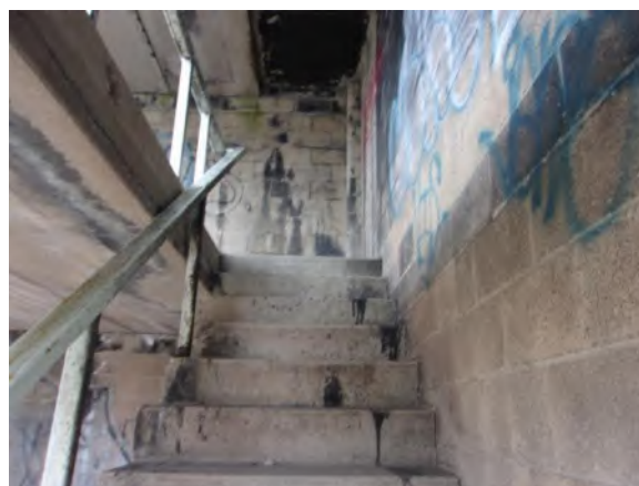
Property fire tower interior stairwell
