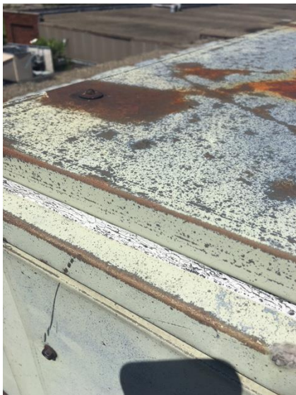
Photo 7: Tan Asbestos-Containing Floor Caulk Located on Roof HVAC Unit.
