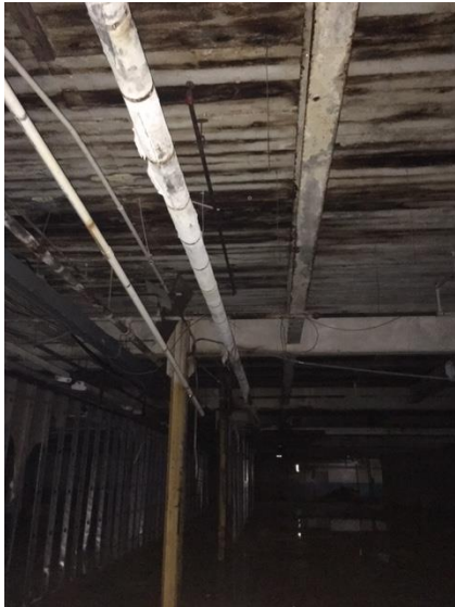
Photo 1: Gray Aircell Pipe Insulation in Warehouse 2.
