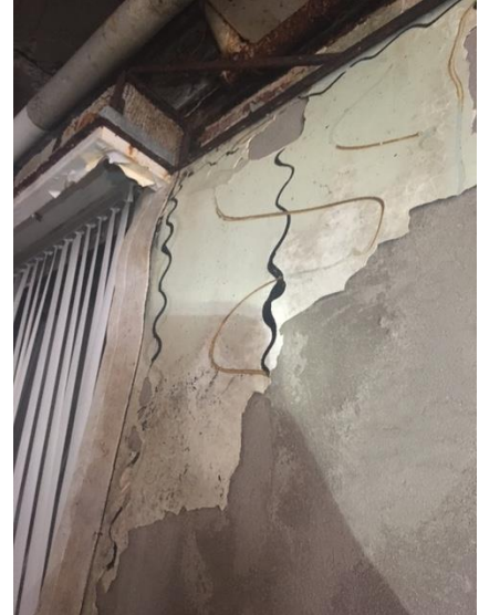
Photo 6: Black Asbestos-Containing Wall Mastic on the 1 st Floor North Wall Near Former HR Area.
