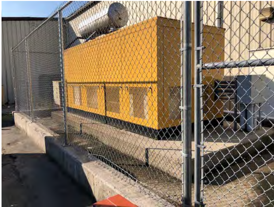
View of the diesel generator located at the rear of the Site, note the AST on top of the unit.
