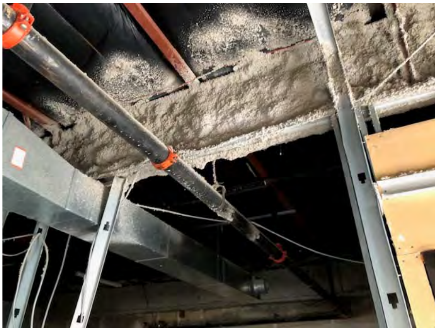
View of the spray-on fire proofing noted on Site.
