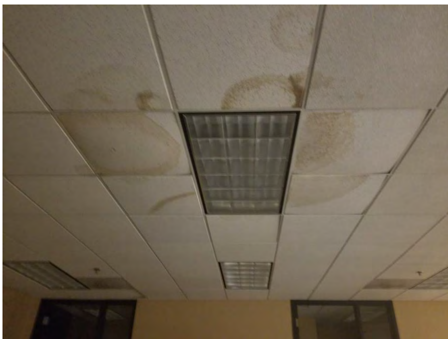
View of water damage to the ceiling tiles of the 1 st floor.
