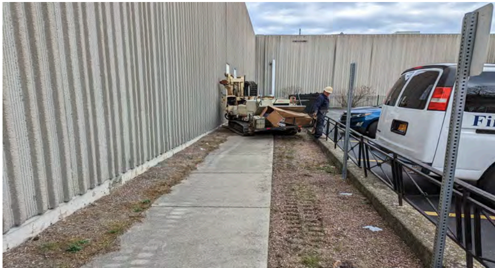
27. BH10 Location. (Facing East)
