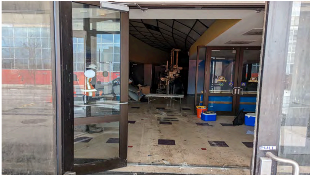
25. BH9 Location. (Facing East)
