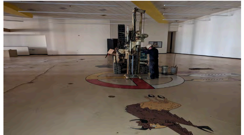
16. BH6 Location. (Facing East)
