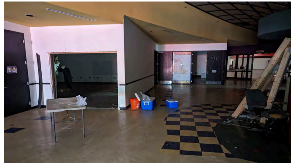
20. BH7 Location. (Looking Northeast)
