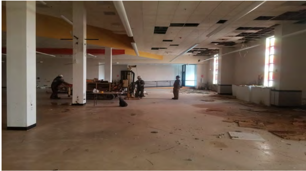
1. BH1 Location. (Facing West)
