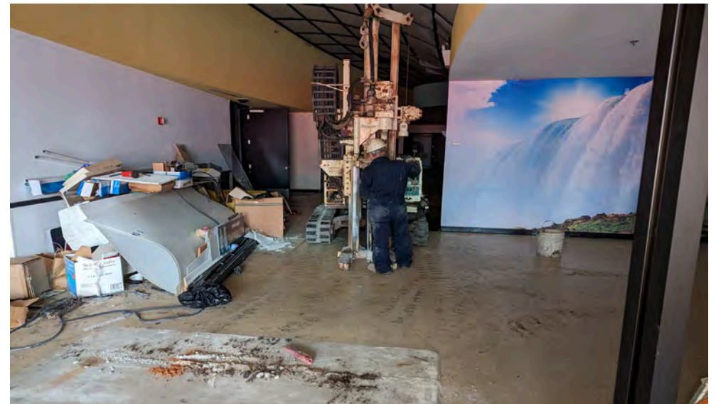
24. BH9 Location. (Facing East)
