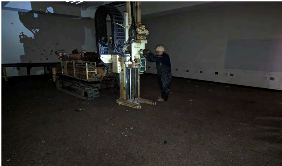
19. BH7 Location. (Looking Northeast)
