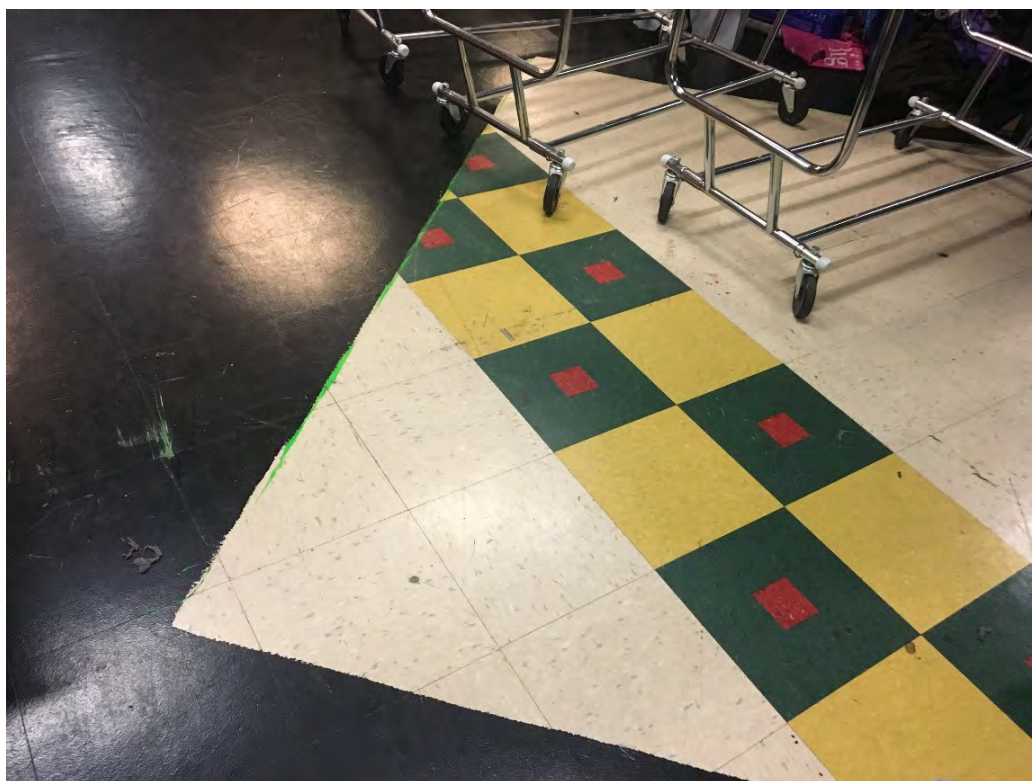
Photo 8 – View of floor tiles in the southeast former indoor miniature golf area and coffee shop. No asbestos was detected in samples of floor tiles or the associated mastic.
