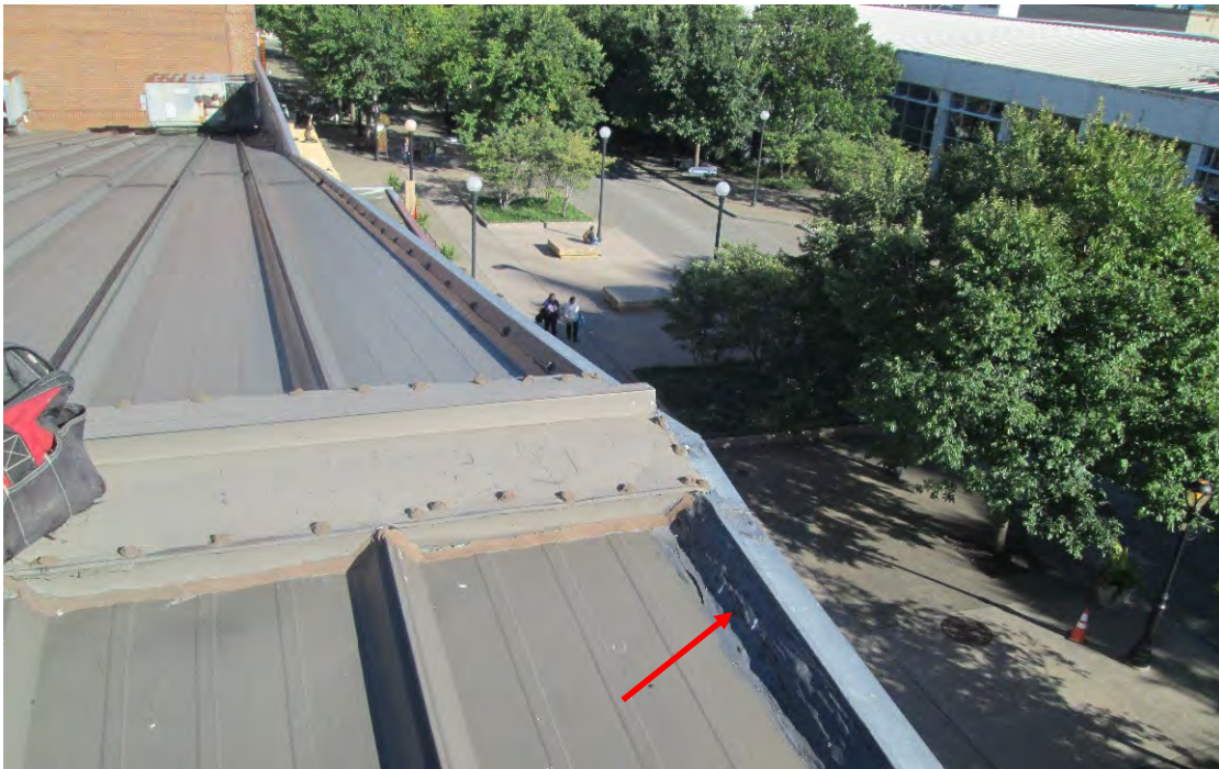
Photo 17 – View of ACM tar along the south parapet of the north-south wing roof (arrow). The tar was observed along the western half of the south parapet only.
