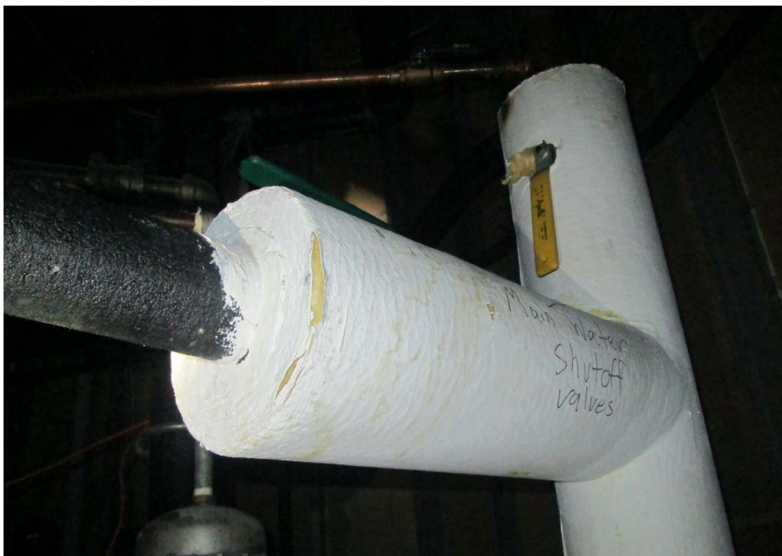
Photo 7 – View of insulation on piping. No asbestos was detected in gaskets, pipe insulation or end sealant.
