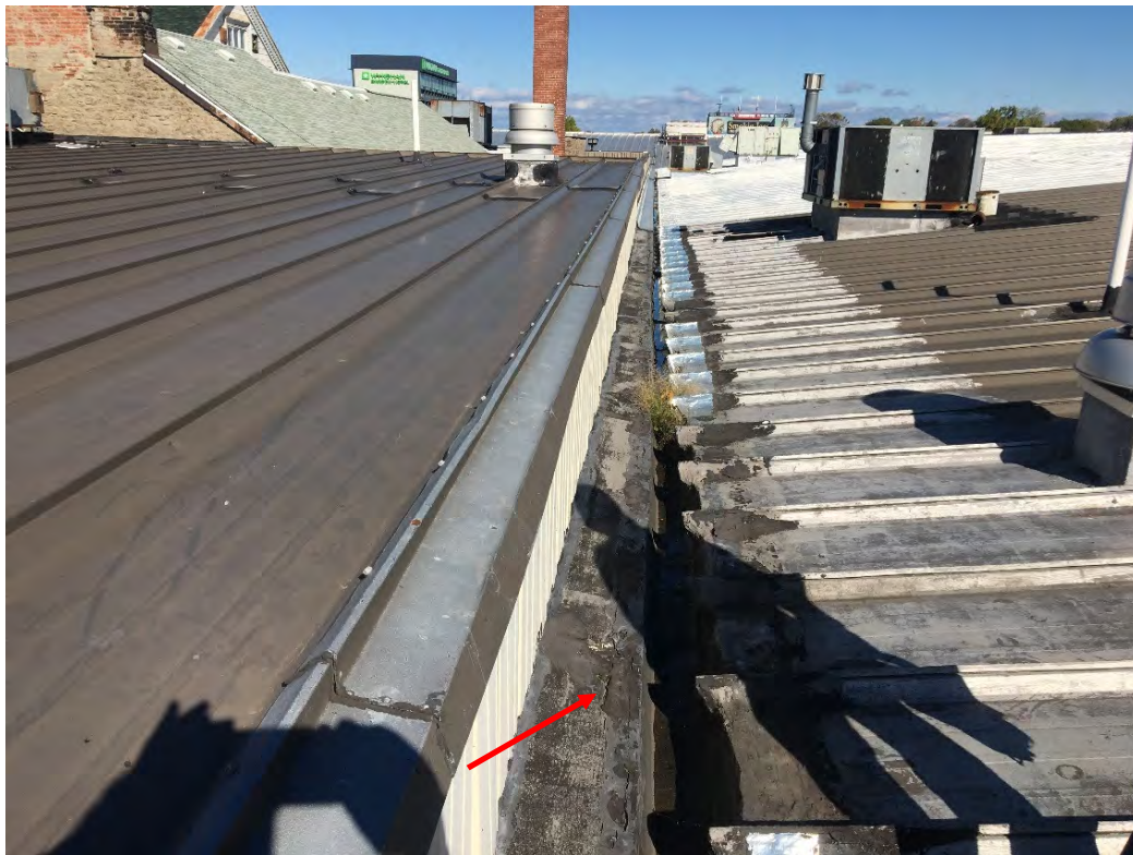
Photo 16 – View of ACM gray-black tar along the eastern edge of the southwest roof (arrow). The same tar was observed as patches along the southwest edge of the adjacent north-south wing roof.
