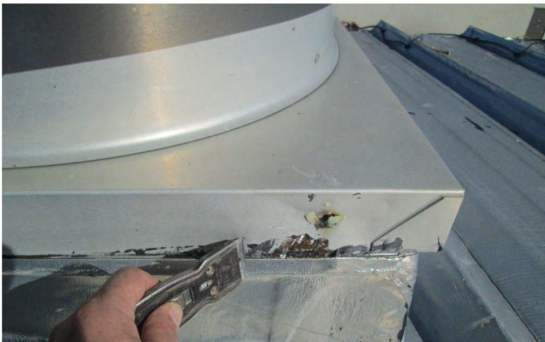
Photo 17 – View of ACM tar along the south parapet of the north-south wing roof (arrow). The tar was observed along the western half of the south parapet only.
