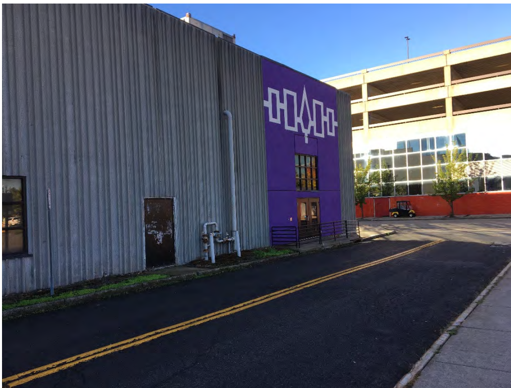
Photo 11 –Exterior view of the north wall of the facility. No asbestos was detected in samples of window glazing compound or window frame caulk, door glazing compound or door frame caulk.
