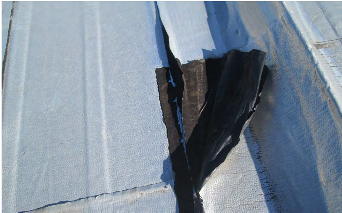
Photo 14 – Close-up view of a section of the metal foil and underlying non-ACM tar across the majority of the roof metal deck. The foil was not observed on the southern portion of the north-south roof or the southwest wing roof.
