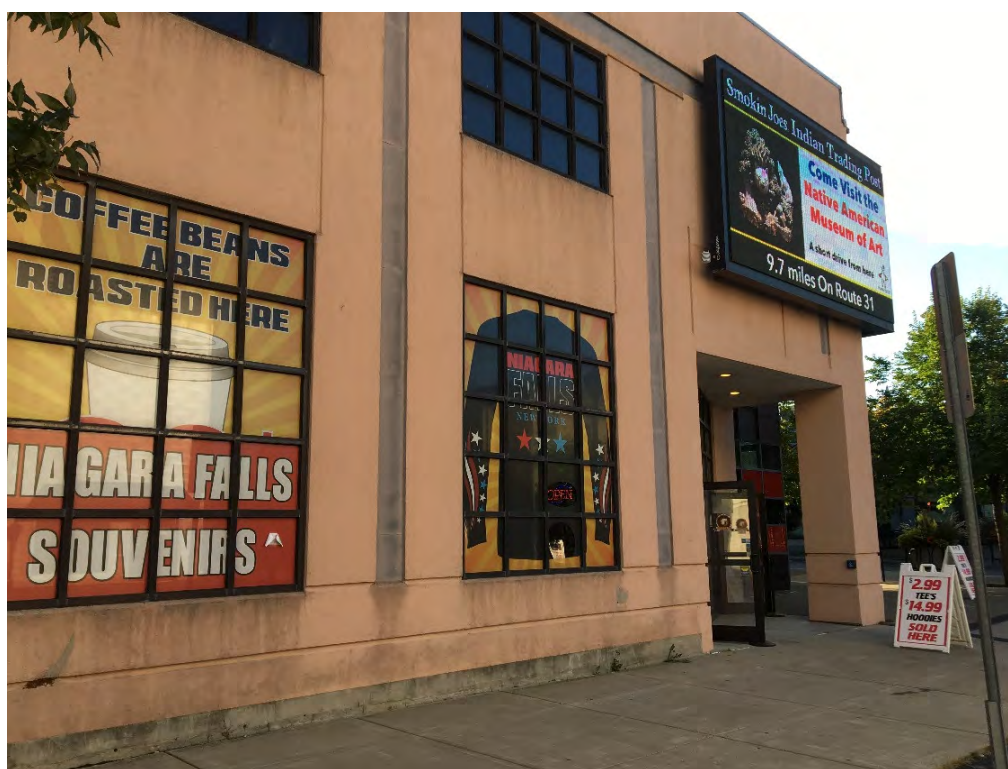
Photo 12 – Exterior view of the southwest elevation. No asbestos was detected in samples of stucco, window glazing compound or caulk.
