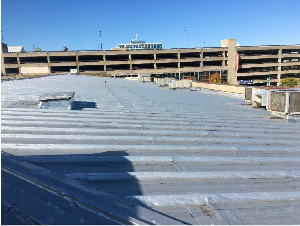
Photo 13 – View of the metal foil and tar surface covering the majority of the metal deck to the roof. ACM black tar was observed at the base of roof mounted components, vents and pipes.
