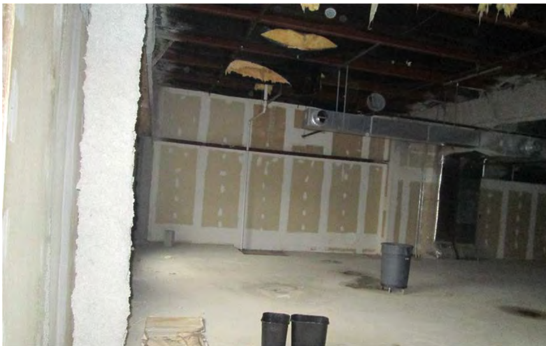
Photo 10– View of the unfinished second floor level. No asbestos was detected in samples of drywall, joint compound, tape, window glazing compound, duct sealant or spray-on fireproofing.
