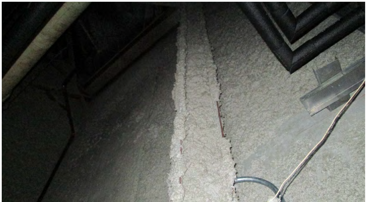
Photo 4 – View of spray-on fireproofing on beams and columns. No asbestos or vermiculite was detected in samples of the spray-on fireproofing.
