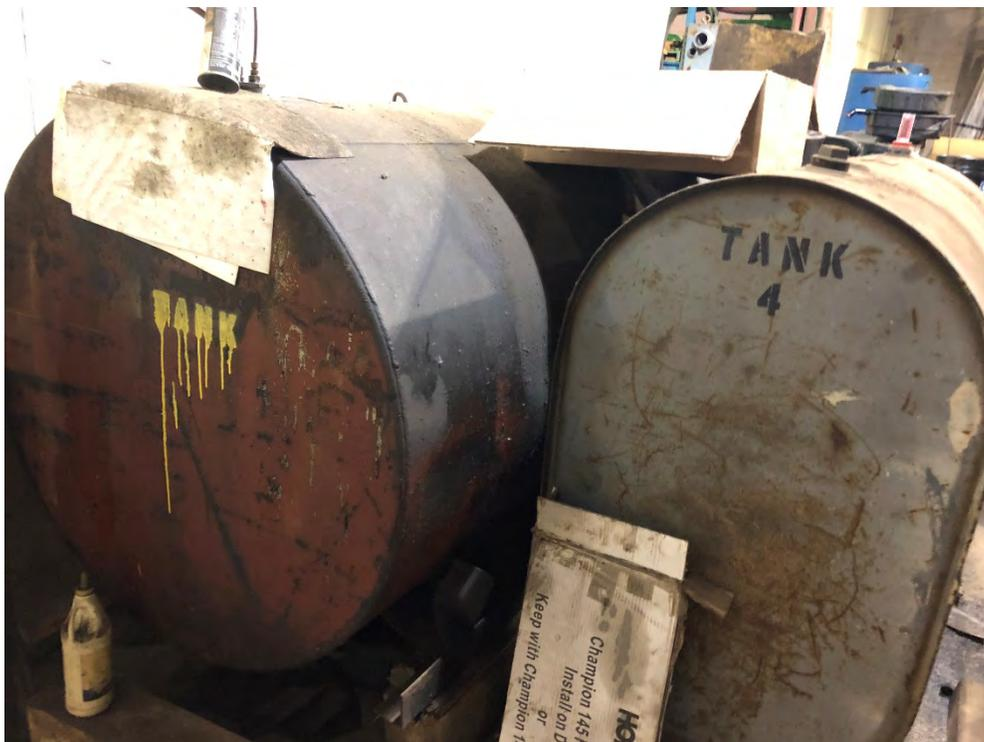
**Tanks 3 and 4 – waste oil tanks. Evidence of consistent spilling below tanks.**
