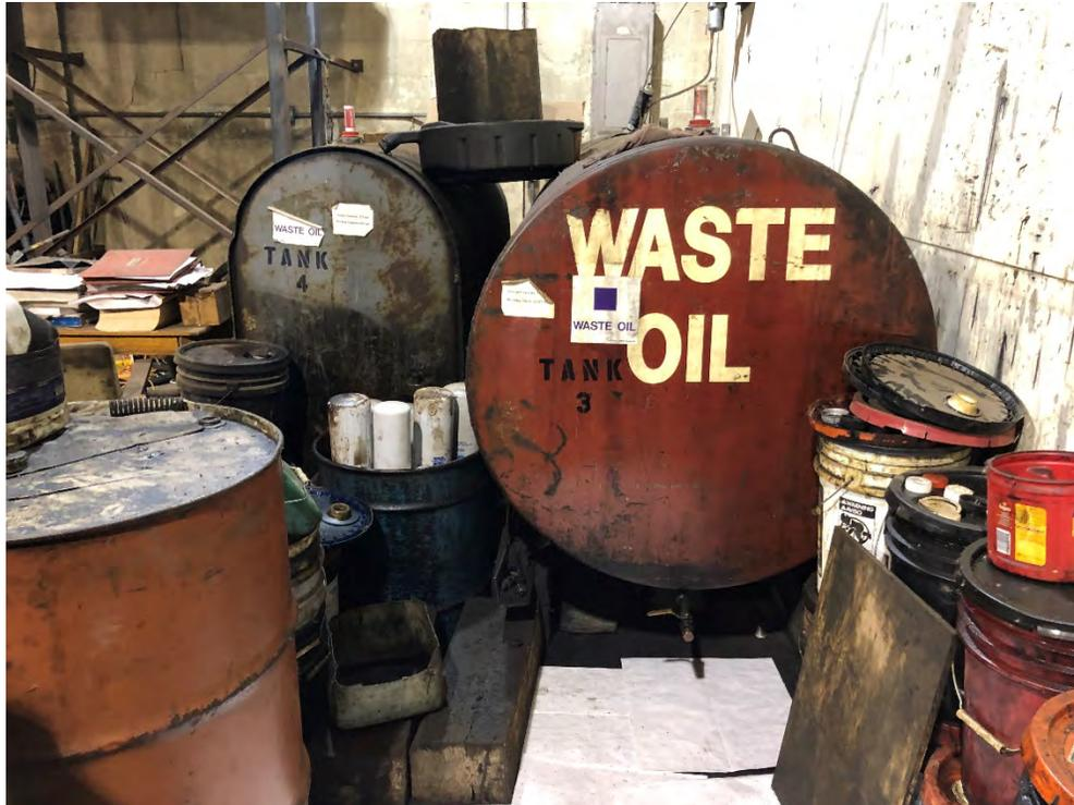
**Tank 3 – 275 gallons; Tank 4 – 575 gallons. Evidence of spilling on floor.**
