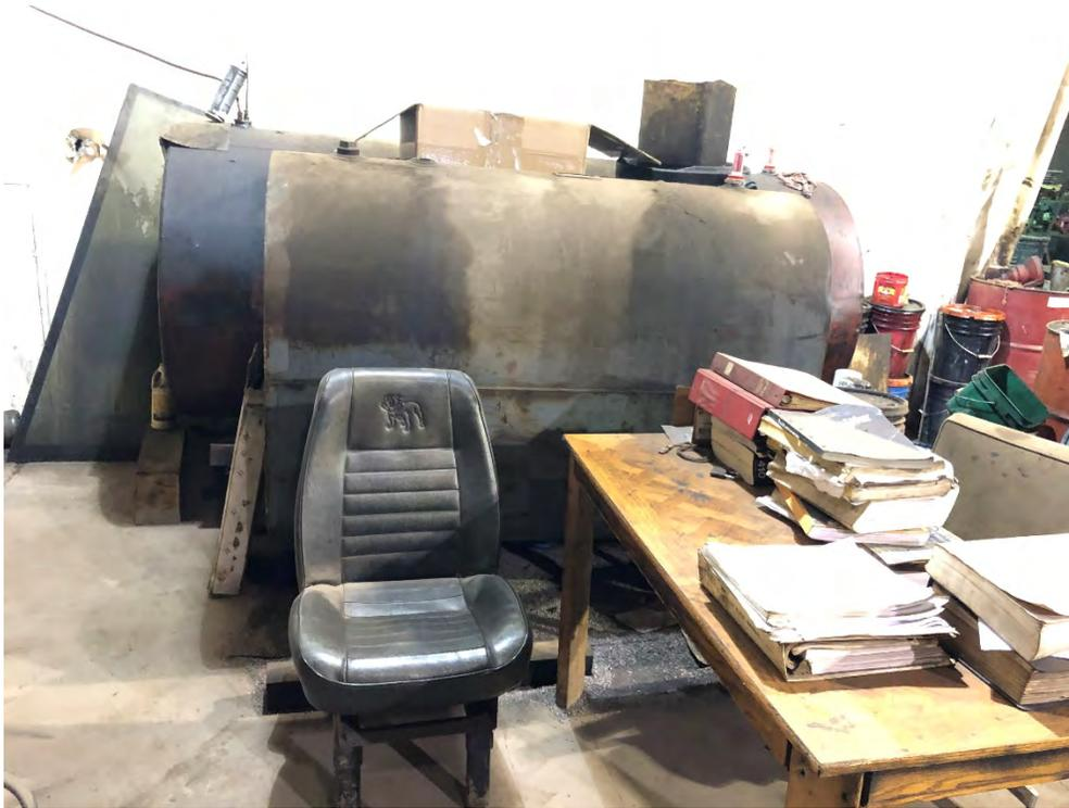
**Two above ground waste oil tanks found inside Building 1. Connected to waste oil burner and used as heating fuel source.**
