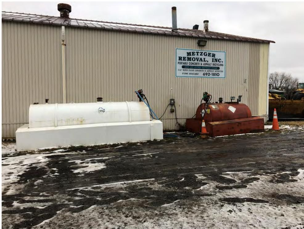
**View of two exterior ASTs (registered Tank Nos. 1 and 2) on west side of Building 2. Contain diesel fuel.**
