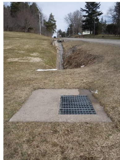
Image 12: Catch basin diverting flow from north side of Route 430 to concrete lined ditch on south side (northeast view direction).
