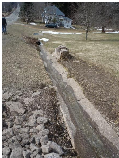
Image 11: Concrete lined ditch on north side of Route 430 leading to catch basin (southwest view direction).
