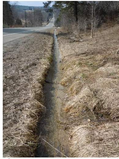
Image 2: Concrete lined ditch on north side of Route 430 (southwest view direction).
