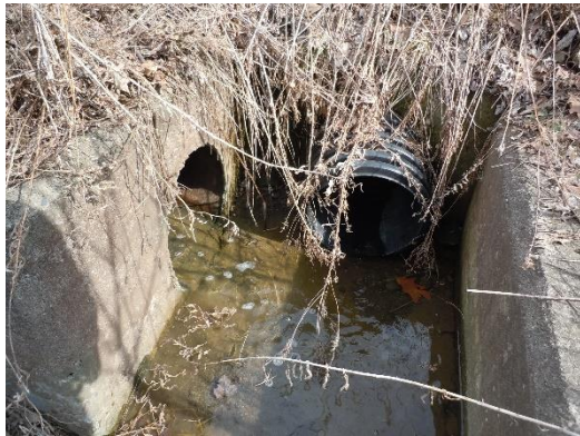
Image 13: Pipe from catch basin (discharge end) diverting flow to south side of Route 430.
