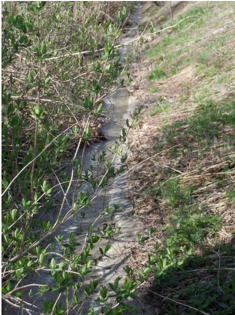
Image 1: Concrete lined highway ditch along north side of Route 430.
