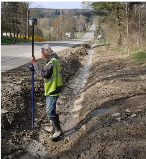
Image 3: Surveying concrete lined ditch along Route 430 (southwest direction)
