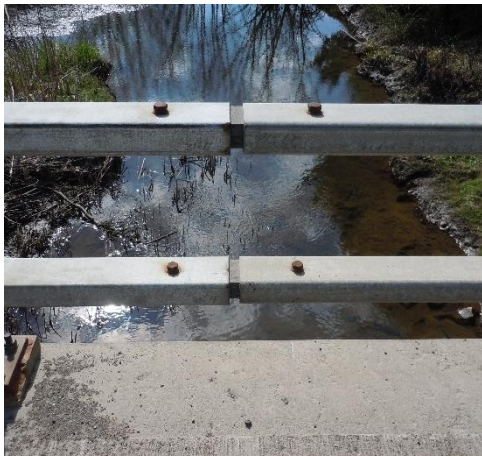
Image 7: Surveyed saw cut on bridge along Sherman-Mayville Road.
