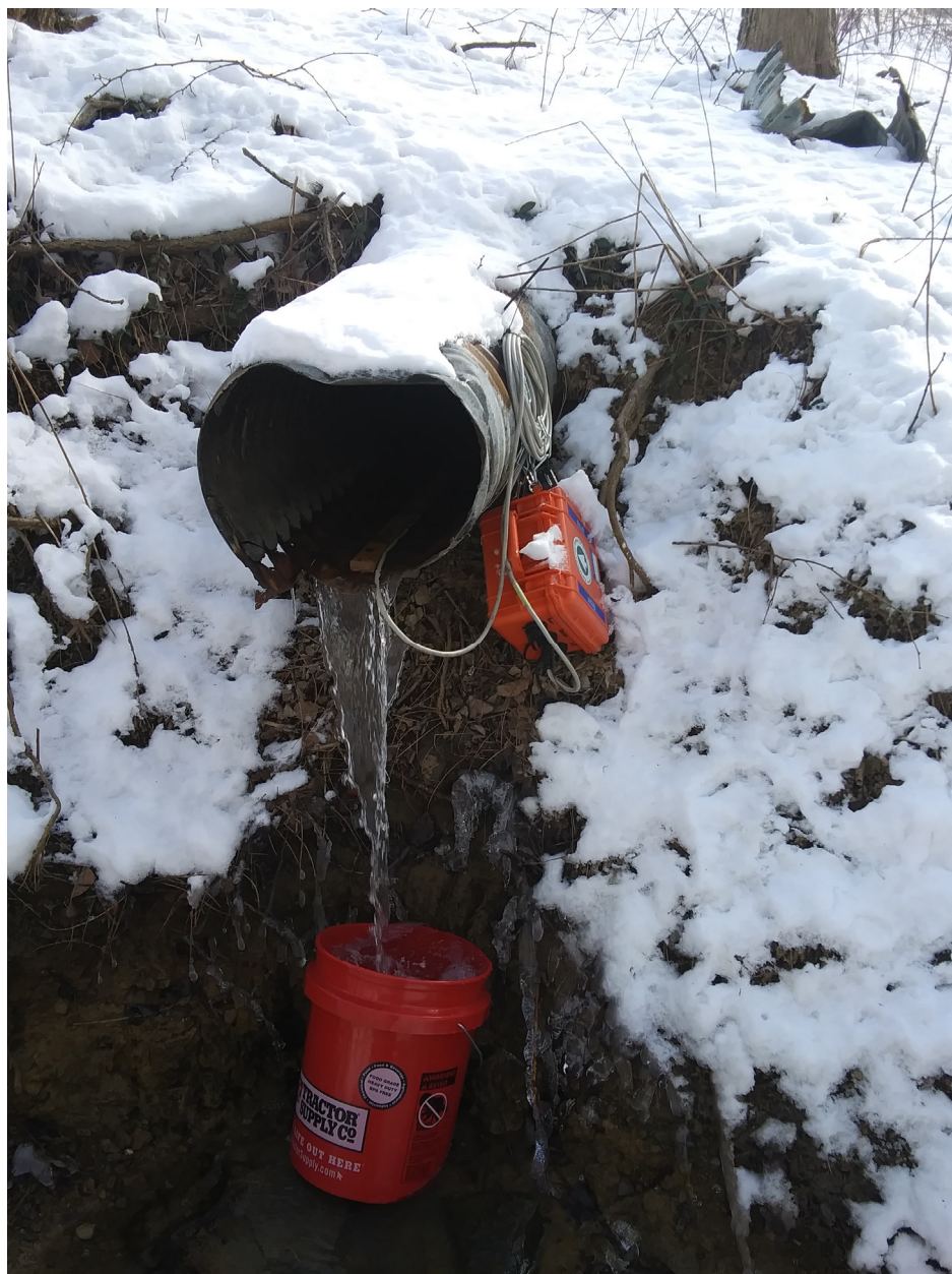
3/9/2023 10:20 AM - View to the north. Typical March discharge flow volume.
