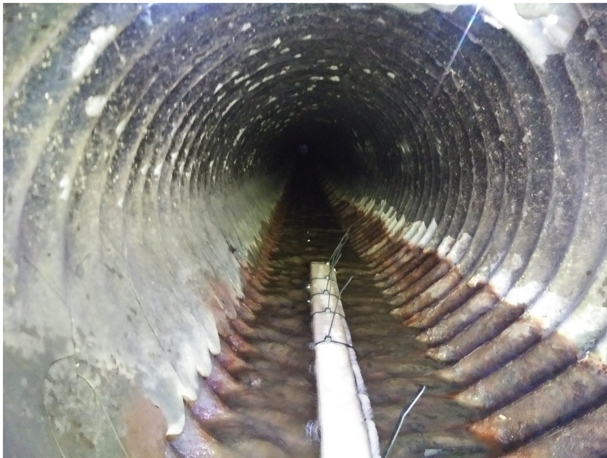
2/8/2023 10:25 AM - View to the northeast Interior of discharge pipe and view of sensor anchor/mount.
