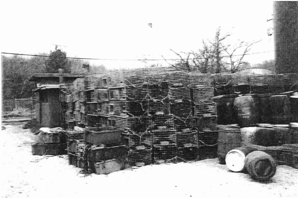
Pump station building and stored lobster pots
