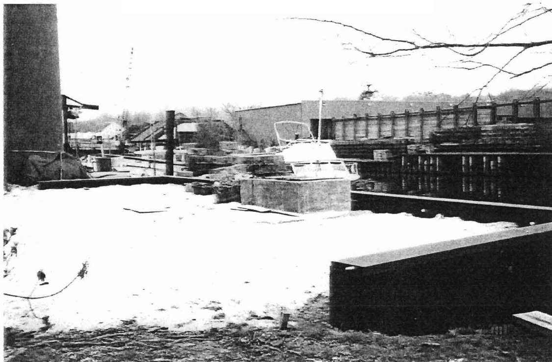
Pump station bulkhead
