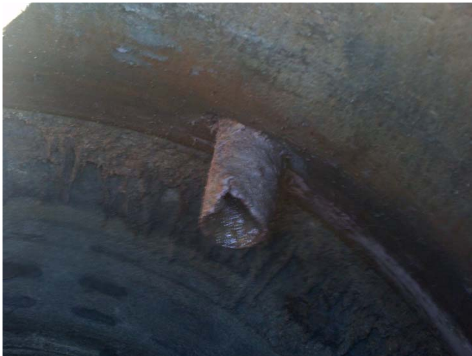
A single four inch diameter pipe was observed in the structure heading towards the northeast.
