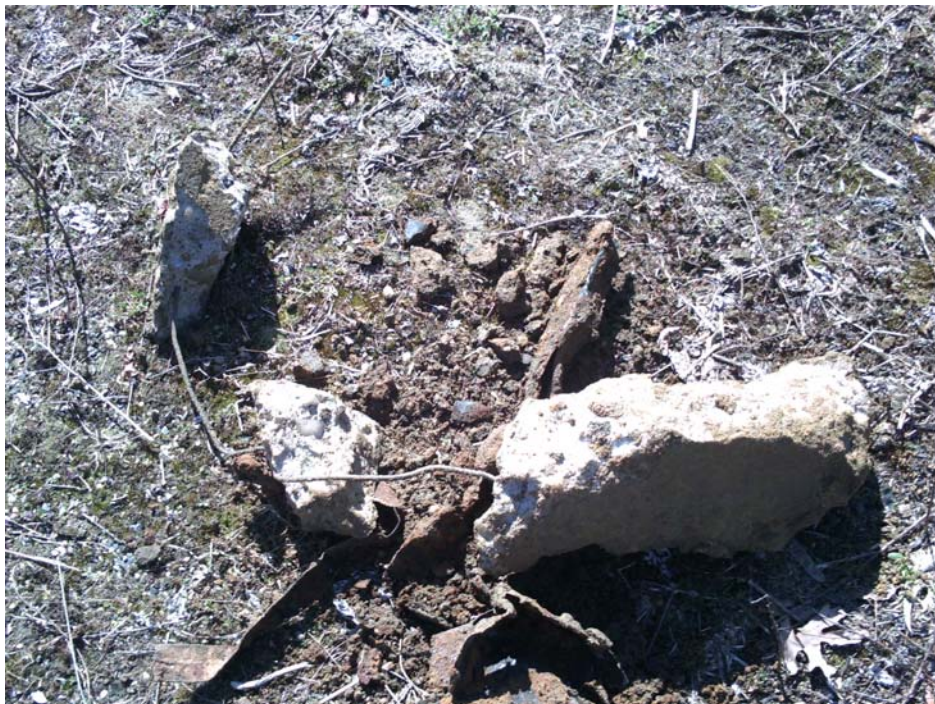
Reinforced concrete debris found at three feet below grade.
