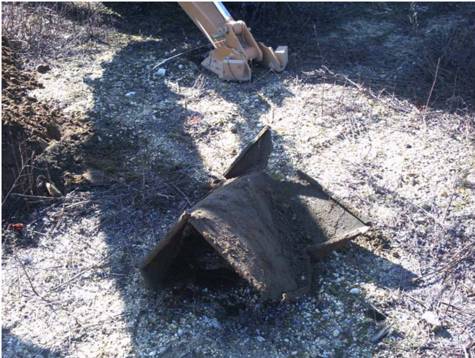
Square piece of sheet metal found at three feet below grade. This is most likely the source of the EM anomaly.
