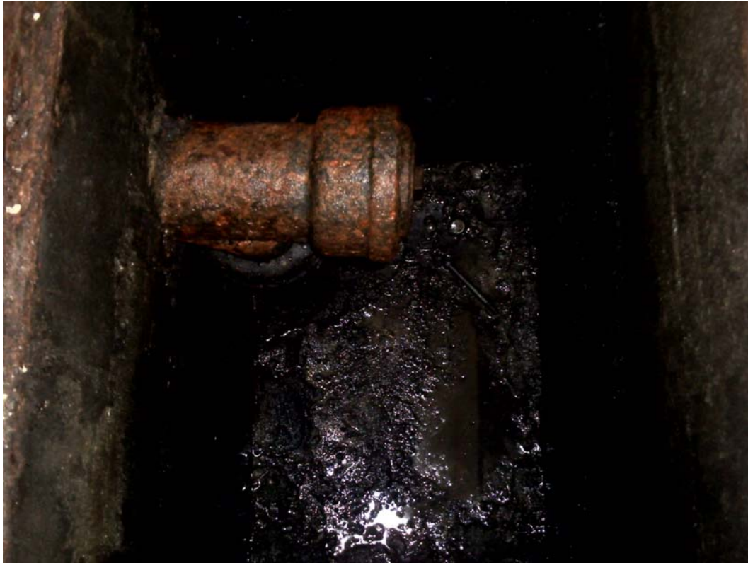
Photo 3: View of floor drain after remediation.
