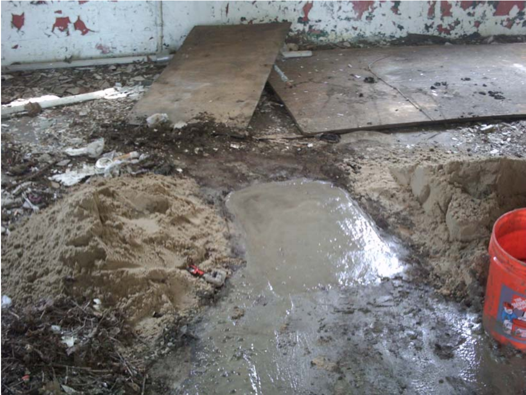
Photo 7: Floor drain backfilled and sealed with concrete.
