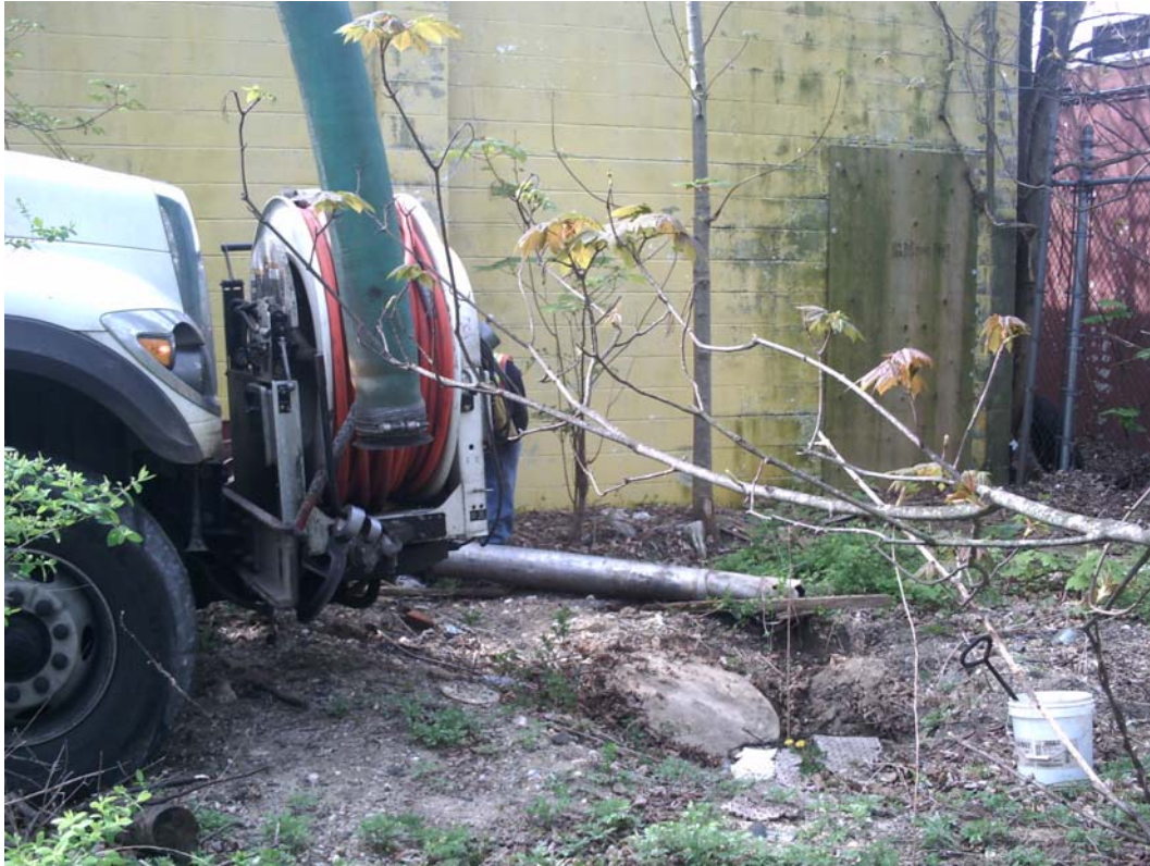
Photo 1: Guzzler truck set up to remove impacted sediment from DW-3.
