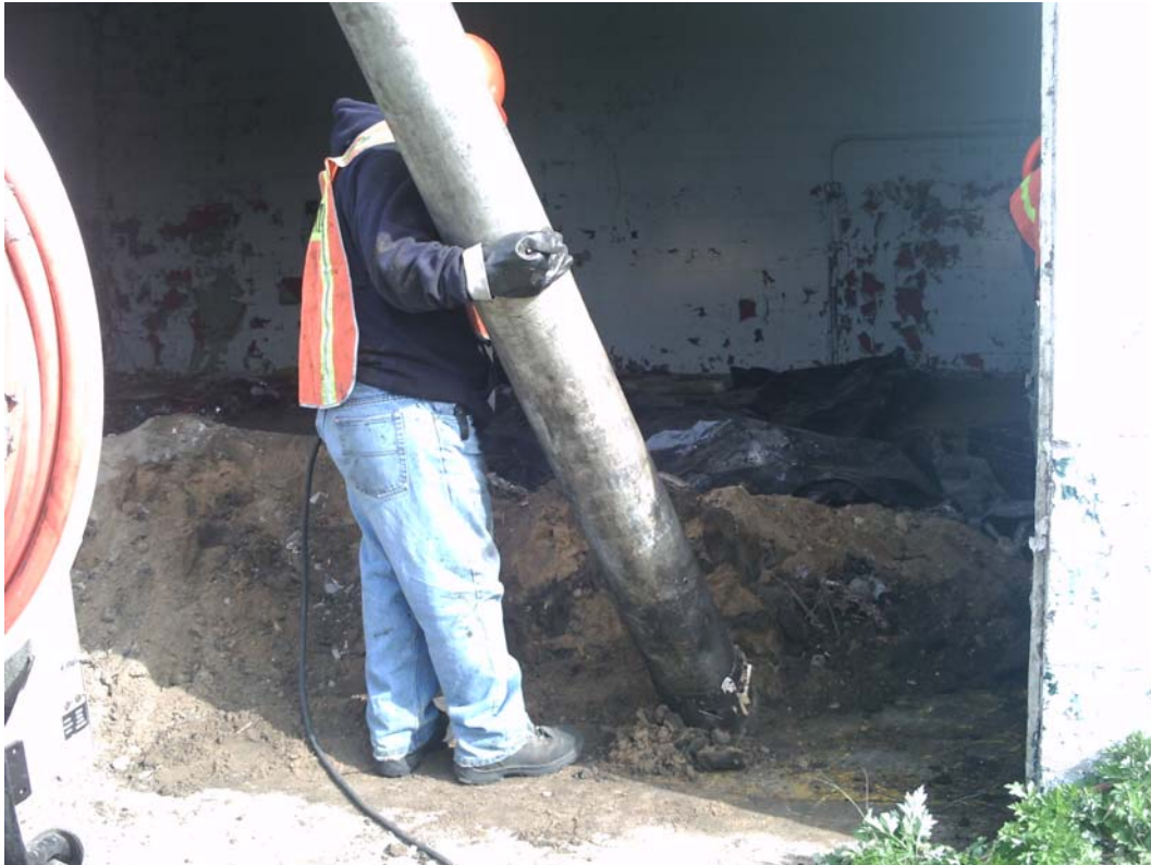
Photo 4: Guzzler removing soil stockpile.
