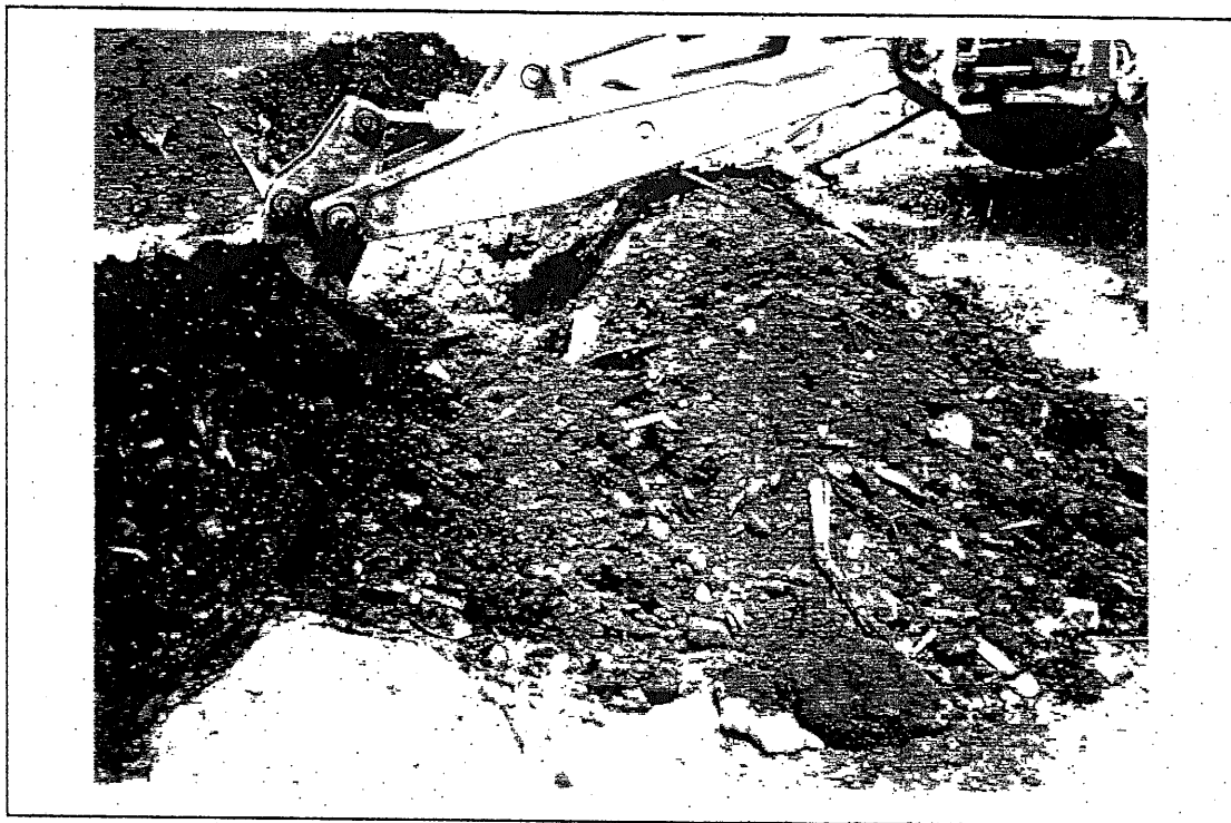
Photo 9: Test Pit 5 C & D material consisting of wood, plastic, and metal pieces.
