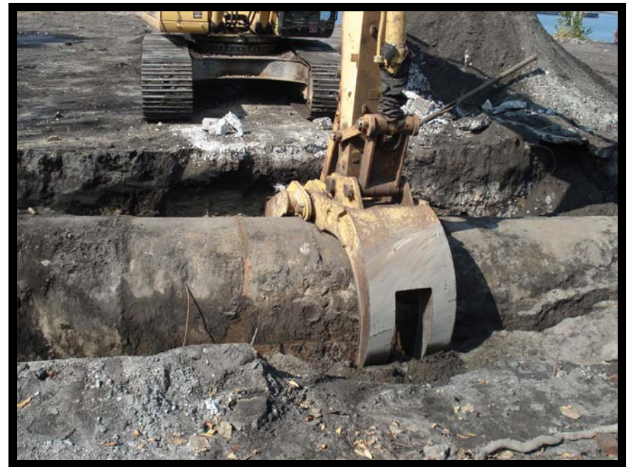
Photo 8 - Removal of UST A
