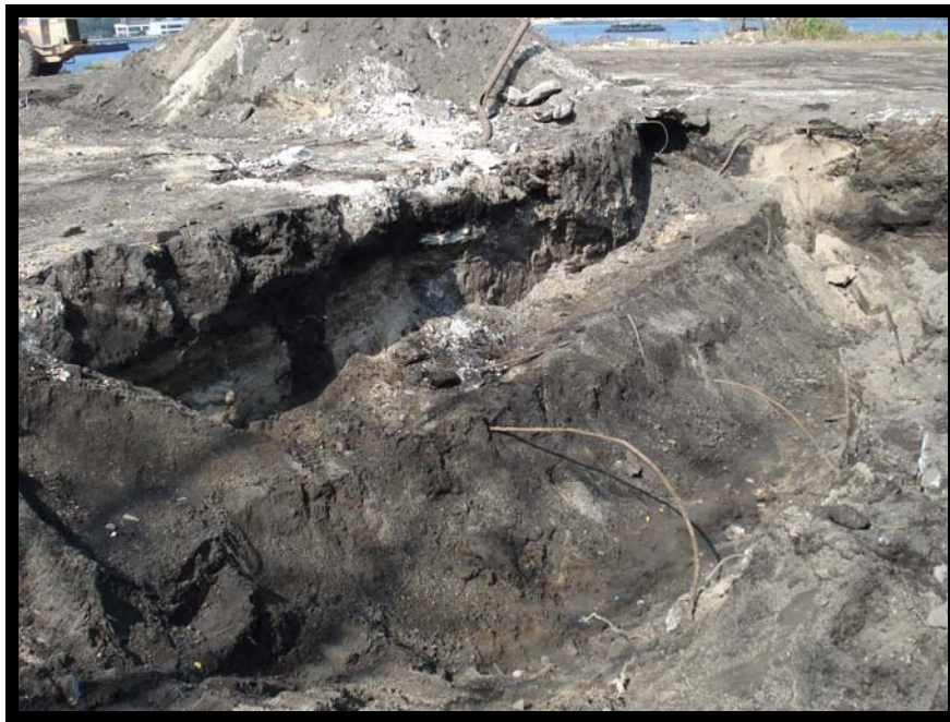
Photo 17 - View of UST A Excavation East Wall
