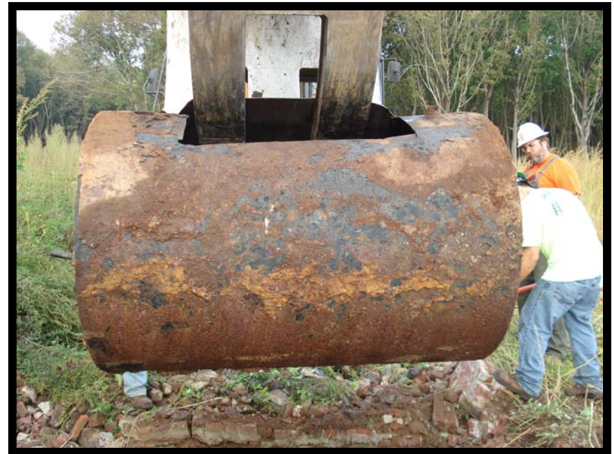
Photo 36 - UST B Removal and Scale Cleaning
