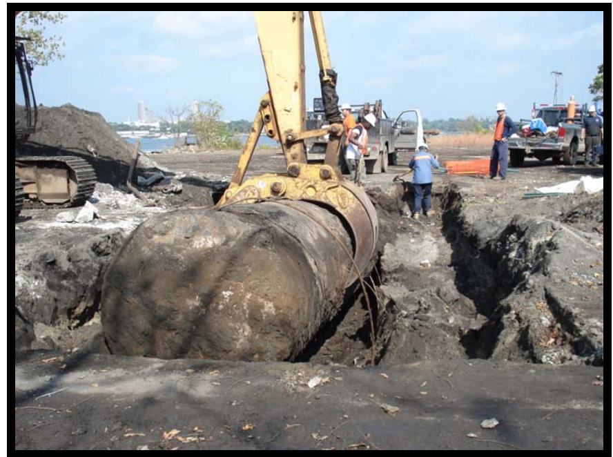
Photo 10 - Removal of UST A
