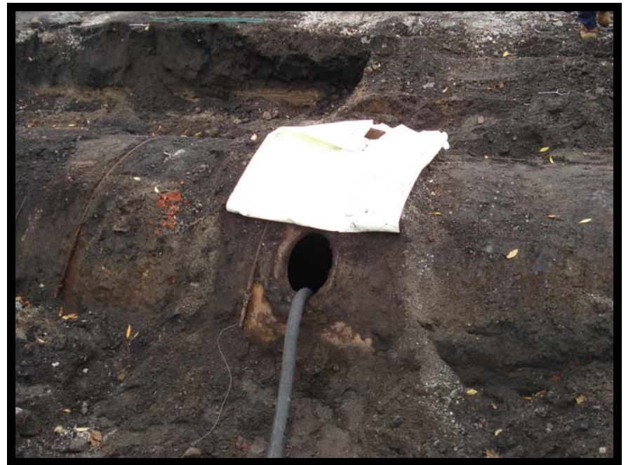
Photo 6 - View of UST A Cleanout
