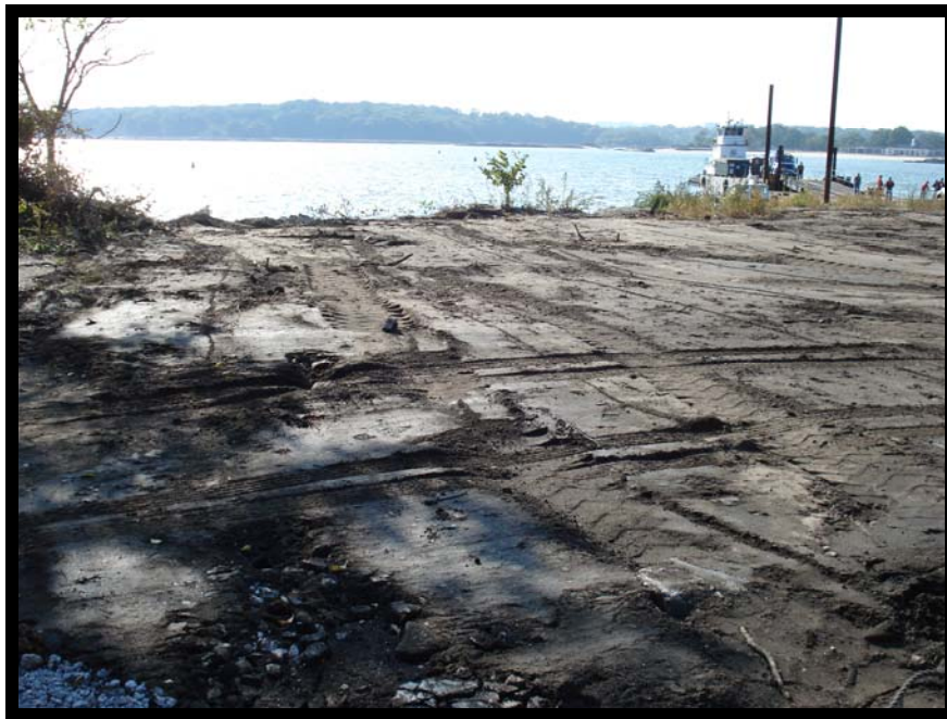
Photo 27 – View of UST A Excavation Restored
