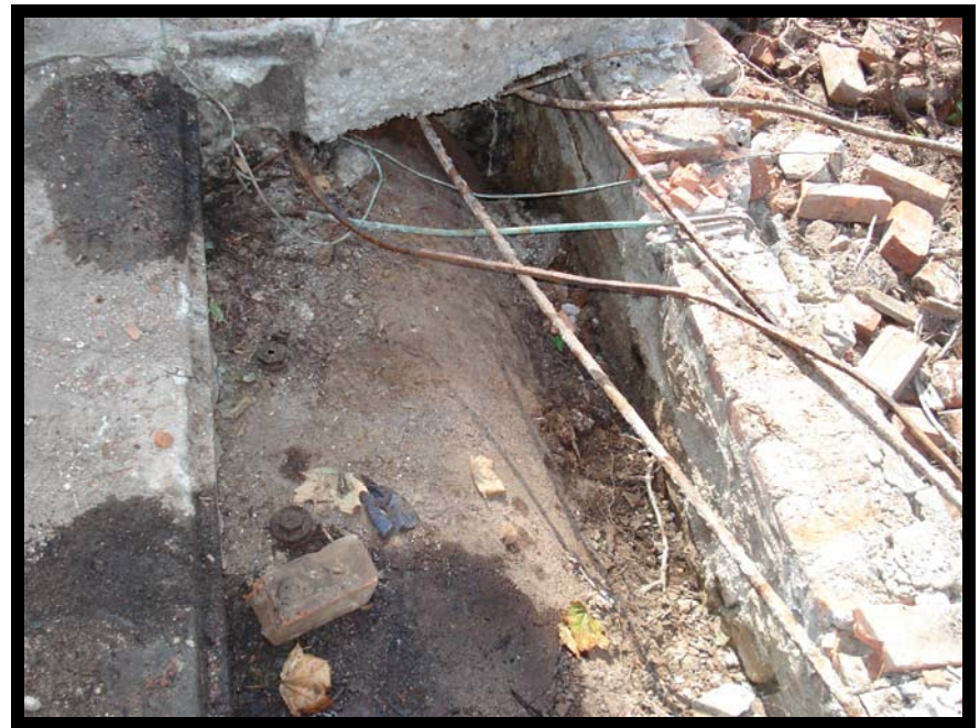
Photo 30 – UST B Prior to Removal
