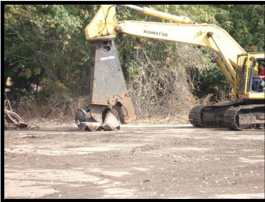
Photo 43 - Shearing of UST B for Disposal
