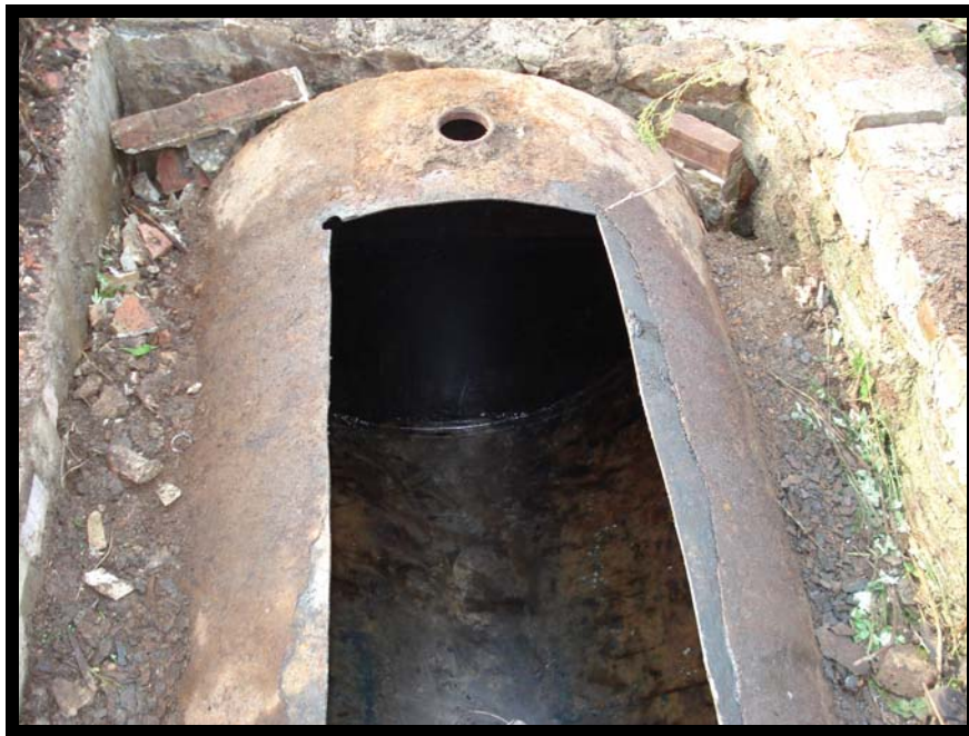
Photo 33 - View of UST B Cleaned Looking North
