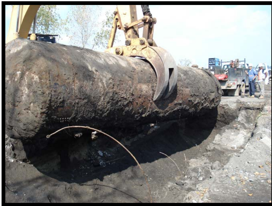
Photo 11 - Removal of UST A
