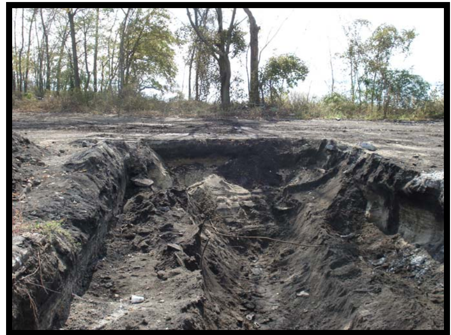
Photo 16 - View of UST A Excavation Looking North
