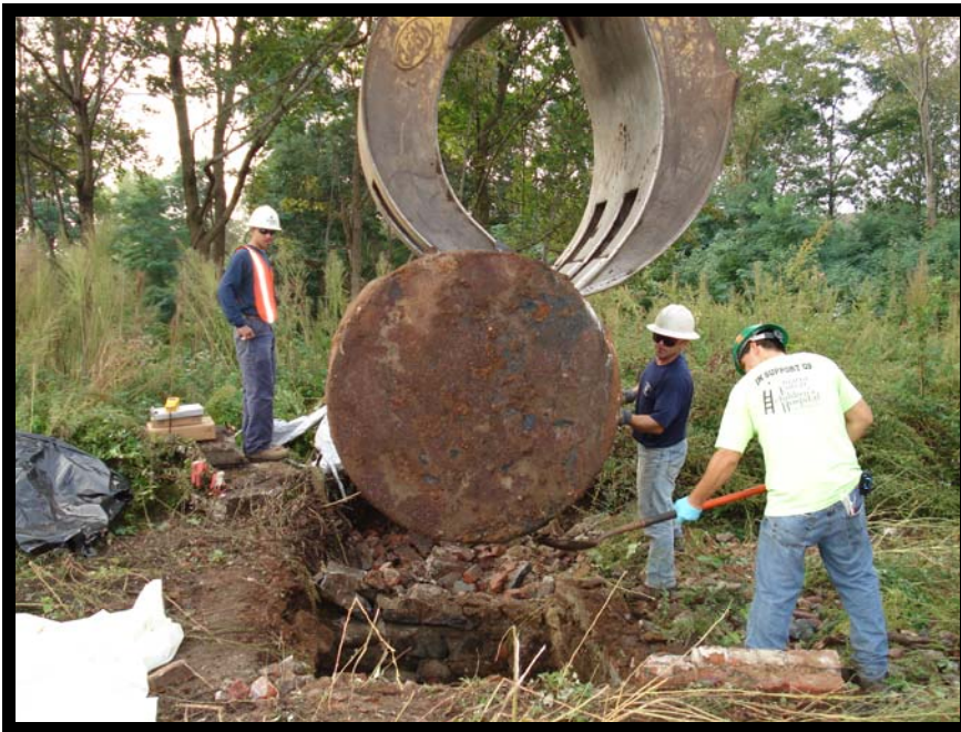
Photo 35 - UST B Removal and Scale Cleaning
