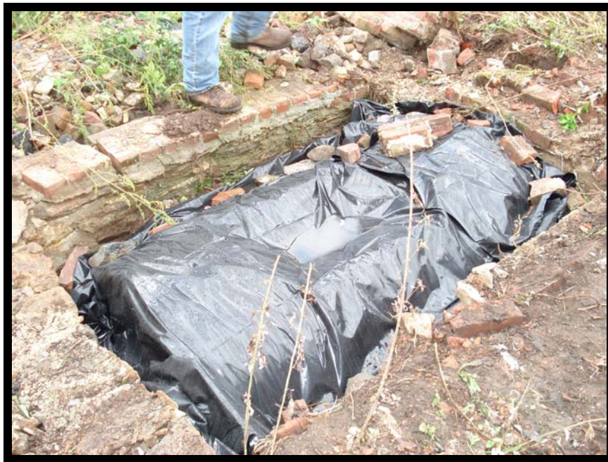
Photo 31 - View of UST B
