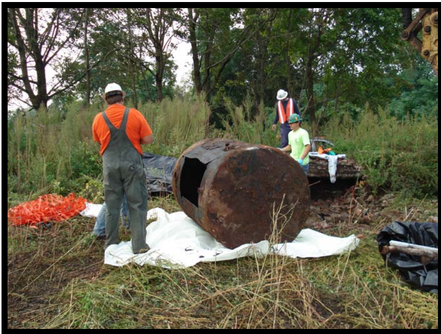
Photo 37 - UST B Removal and Scale Cleaning
