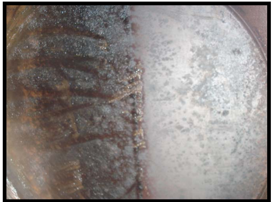
Photo 38 - View of Interior North Side of UST B
