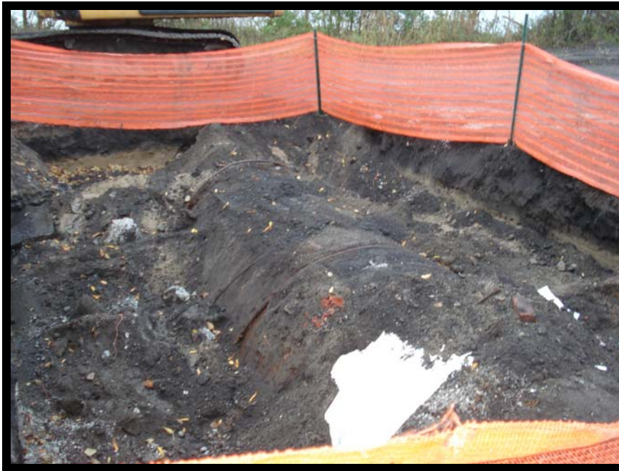
Photo 1 - View of UST A Looking South
