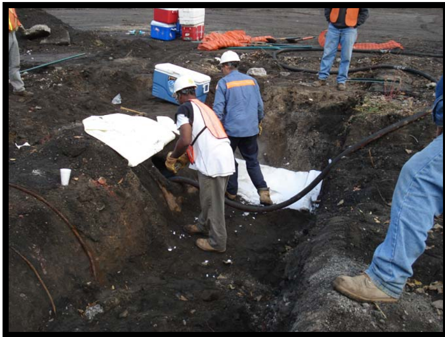
Photo 5 - View of UST A Cleanout
