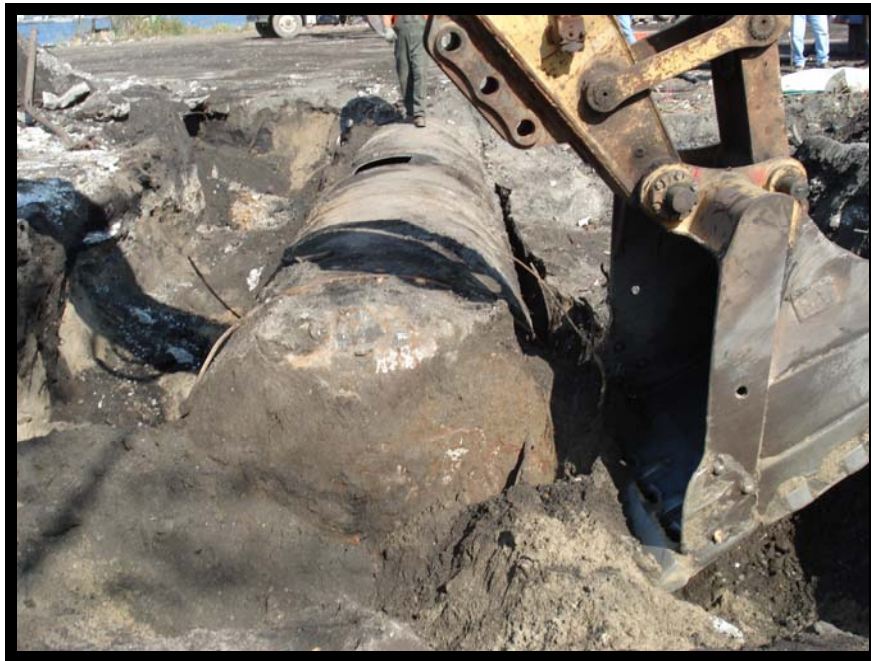
Photo 3 - Excavation of UST A
