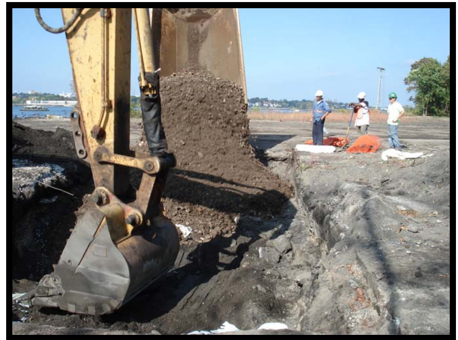
Photo 26 - Backfilling UST A Excavation
