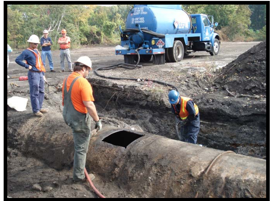
Photo 4 - View of UST A Cleanout
