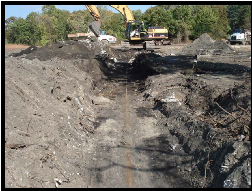
Photo 21- View of UST A Piping Looking North
