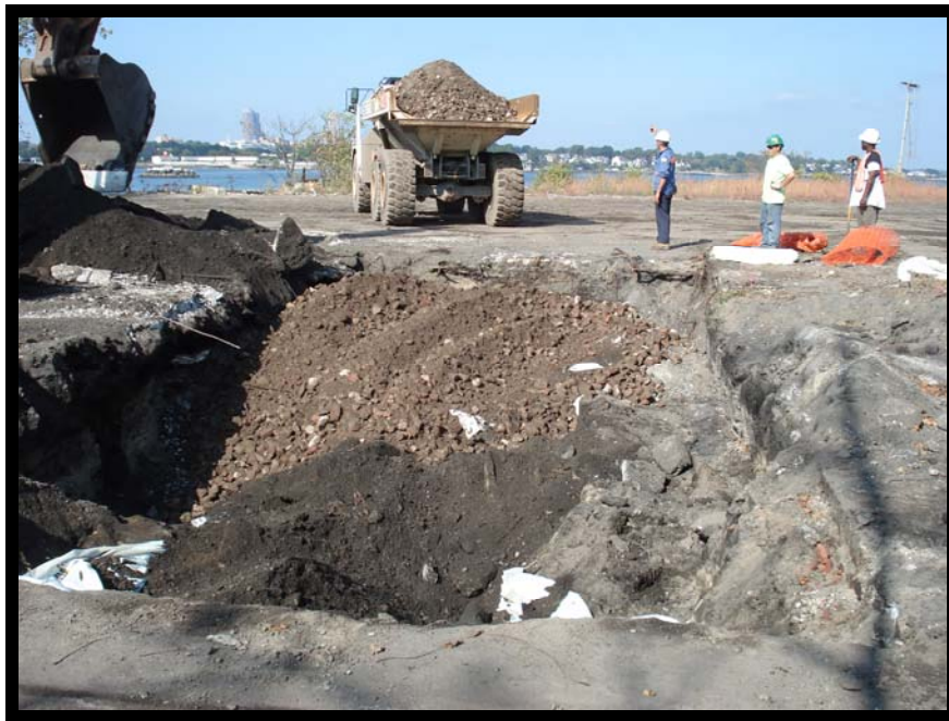
Photo 25 - Backfilling UST A Excavation
