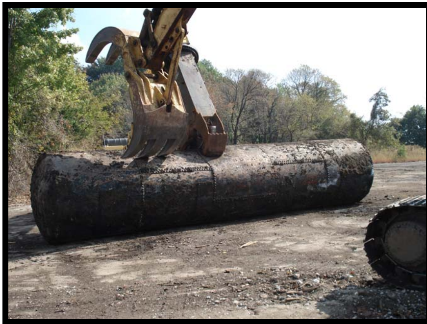
Photo 29 - Shearing UST A for Disposal
