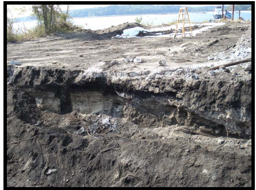
Photo 18 - View of UST A Excavation West Wall
