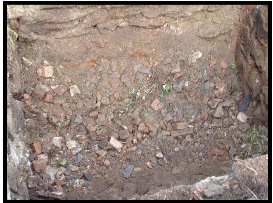
Photo 42 - View of UST B Tank Vault
