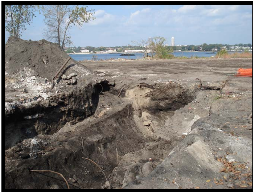
Photo 15 - View of UST A Excavation Looking South
