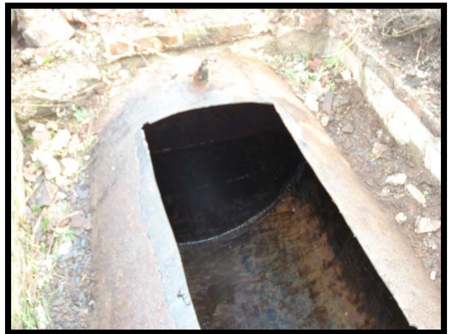
Photo 34 - View of UST B Cleaned Looking South
