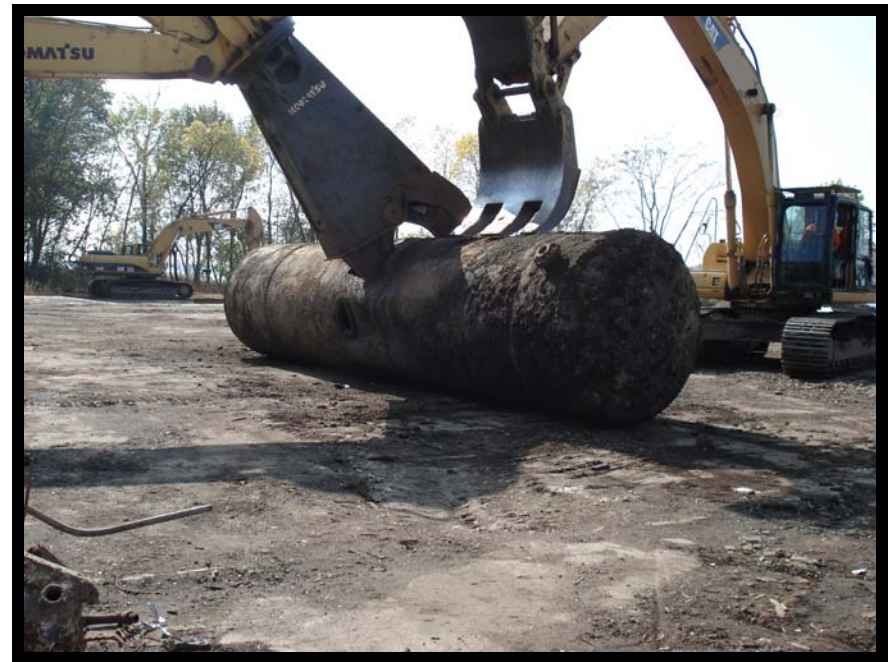
Photo 28 – Shearing UST A for Disposal
