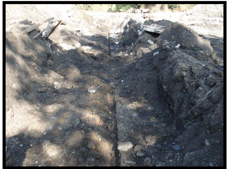
Photo 22 - UST A Piping Excavation
