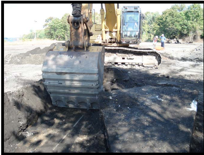
Photo 19 – Excavation of UST A Piping
