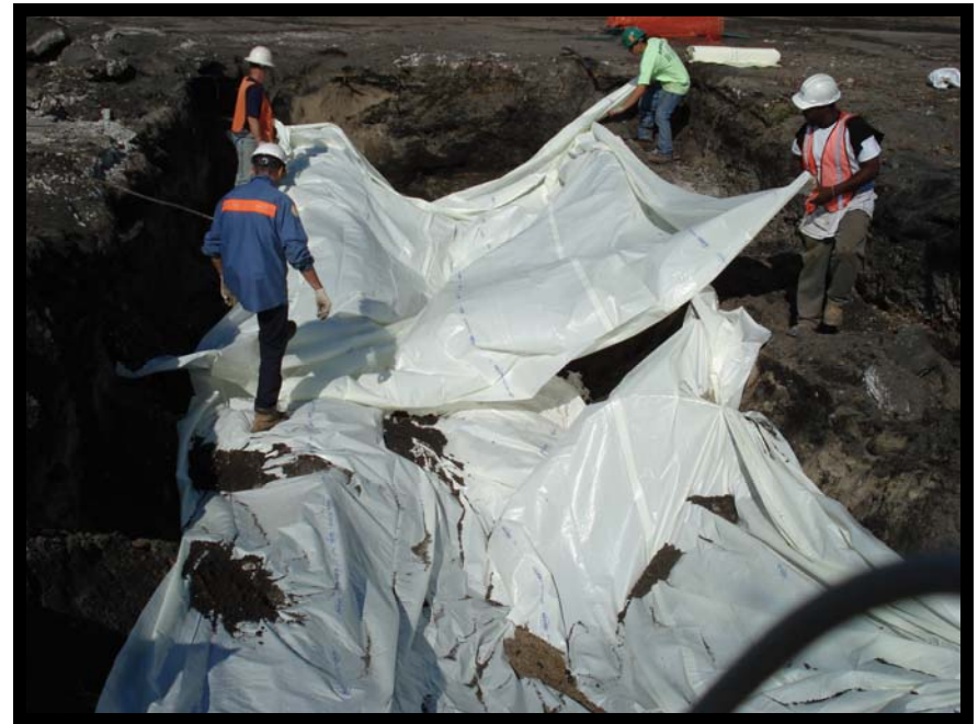
Photo 24 - Laying Plastic in UST A Excavation
