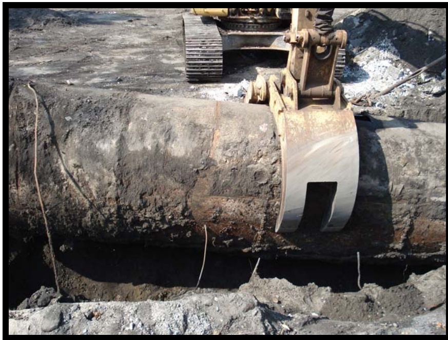
Photo 9 - Removal of UST A
