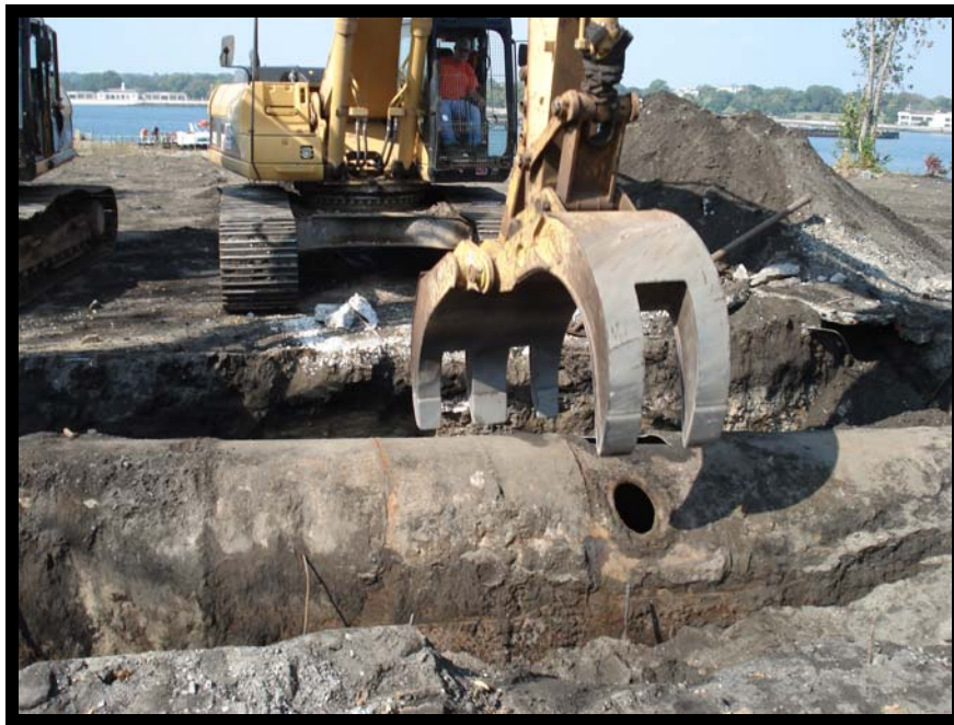
Photo 7 - Removal of UST A
