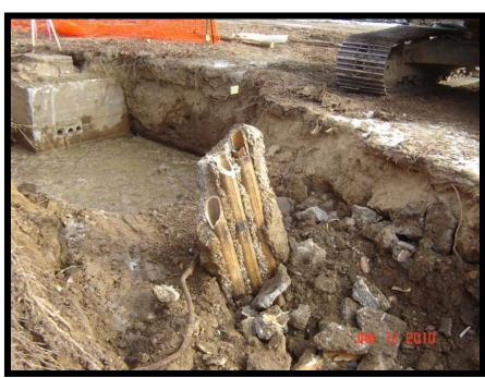
Photo 12 – View of Conduit and Electrical Junction Box in Area 4-2
